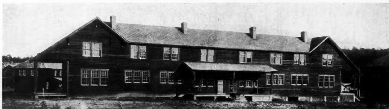
Group of Four 4-Room Workingmen's Houses at Bodin, N. C. (Southern Aluminum Co.) Constructed Largely of Carey "Ceil Board."
