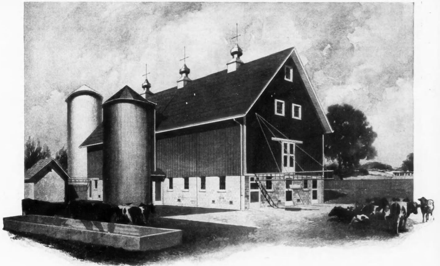
The Remodeled Dairy Barn. A Heavy Timber Frame Raised Up and Set on a 12-Inch Glazed Tile Wall. Size of Barn, 100 by 36 Feet. We will gladly answer all inquiries for further information about this Cow Barn.—Editor.
