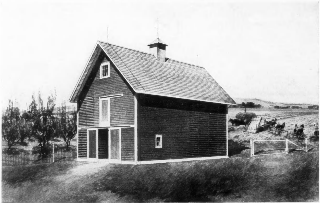
Design for 2-Story Corn Crib and Granary. A Popular Labor-Saving Grain Storage Building. Dimensions 48 by 26 Feet. If you wish further particulars concerning the plans for this building or special materials used in its construction, write to us.—Editor.
