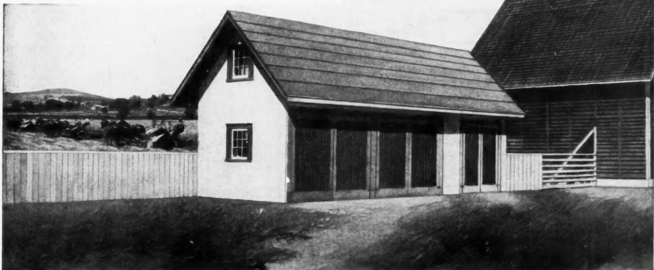
Design for Implement Shed and Farm Blacksmith Shop. Dimensions 48 by 16 Feet. Walls are Constructed of Cement Plaster on Metal Lath, Attached to 2 by 4 Studs, Door Posts, 8 by 8.
