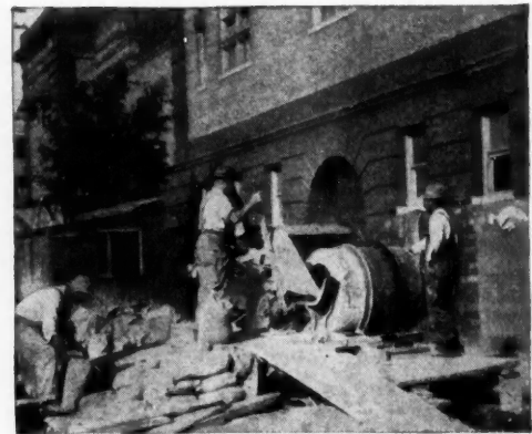
"Standard" Low-Charging Mixer at Work on Large Pasteurization Plant for the Borden Condensed Milk Co., New York.
