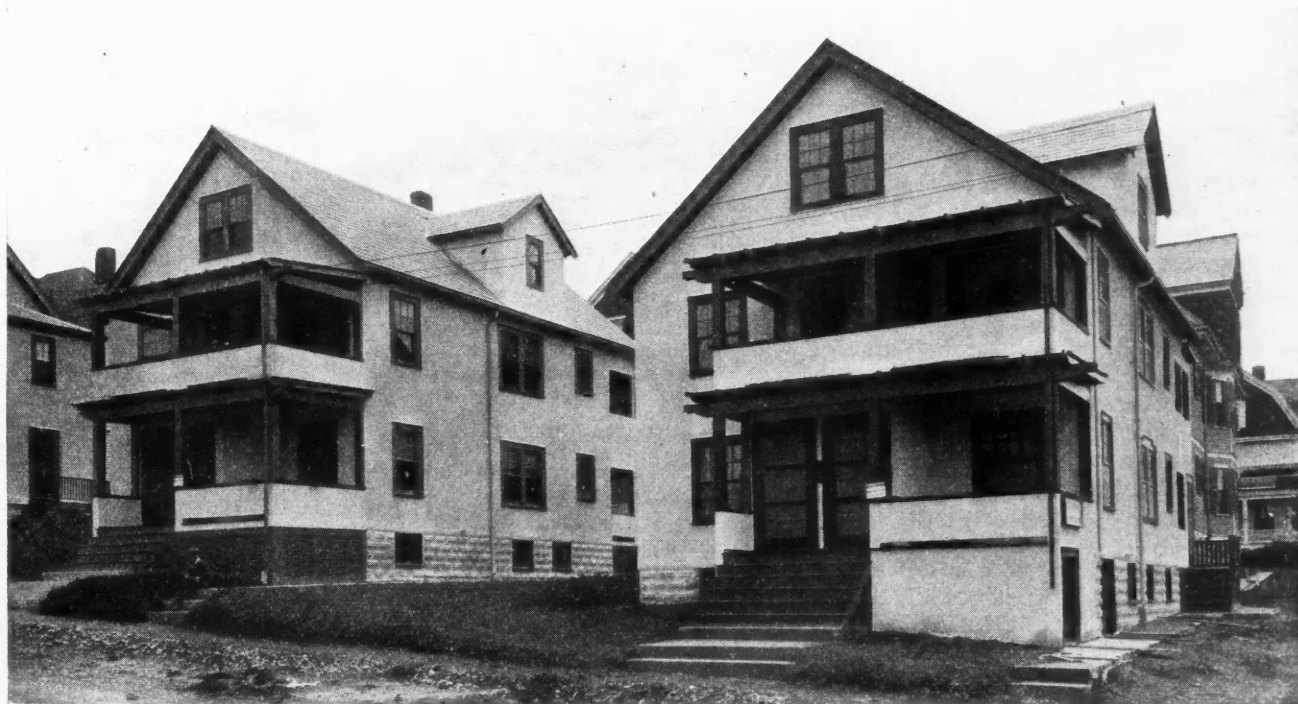
Two Duplex Apartments at Arlington, Mass. Designed and Built by John C. Cameron. Examples of the High Quality Work Being Done with Cement Plaster on Stucco Board.
