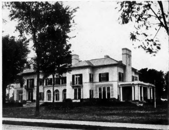
Residence of S. S. Kresge, Detroit, Coated with "Bay State."
