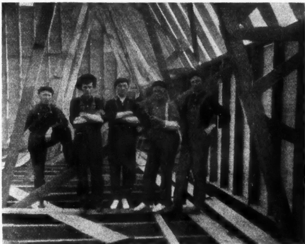
Barn Builder Bjorklund and Crew.
