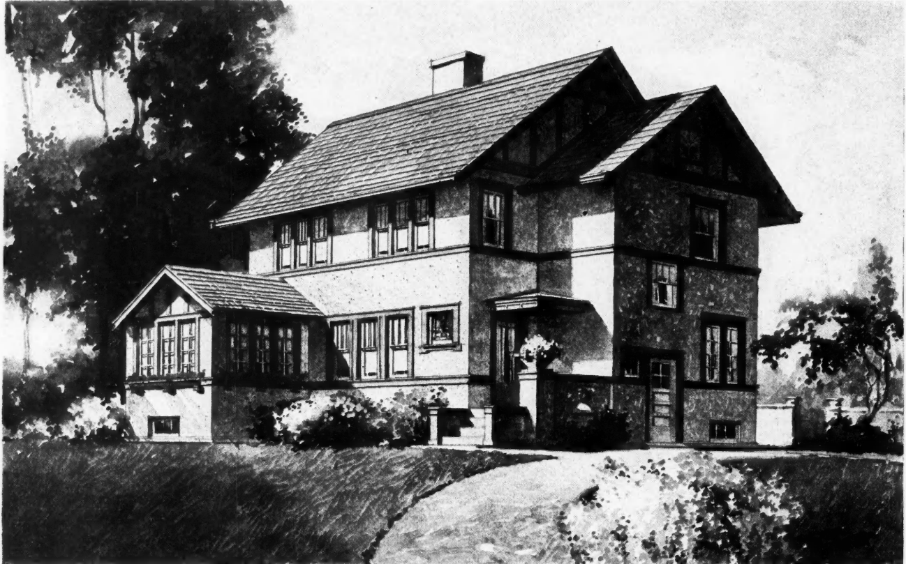
Hollow Tile, Stucco Covered Residence. Size 35 feet by 25 feet 6 inches. We can furnish complete set of blue-printed working plans and typewritten specifications for only $12.00 per set. Blue-prints consist of basement plan; roof plan; first and second floor plans; front, rear, two side elevations; wall sections; and all necessary interior details. Specifications consist of twenty-two pages of typewritten matter. When ordering, ask for Design No. 6675.
