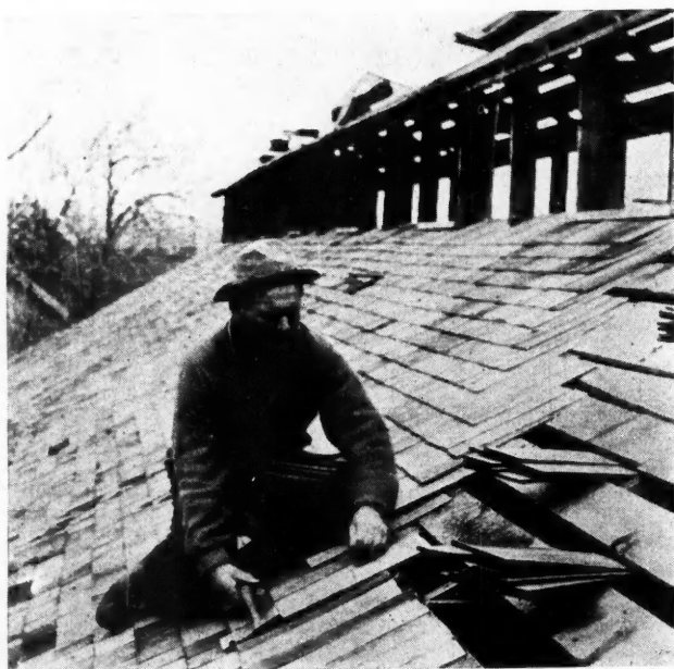
Shingler Pierce on the Job—He Puts on a Bundle in 12½ Minutes.
