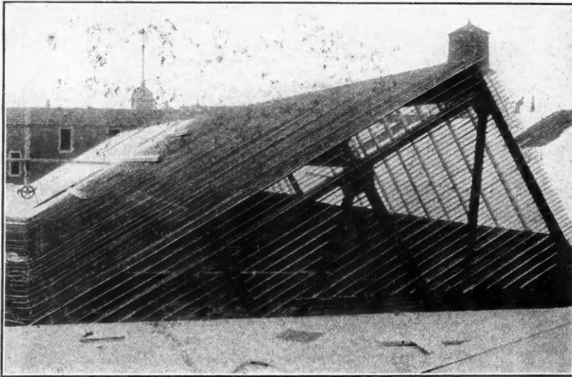
The Saw-Tooth Roof of the Mack Motor Truck Garage, Cambridge, Mass., is Constructed of "Corr-Mesh," which Serves Both as Reinforcing Steel in the Finished Slab and as Forms for the Wet Concrete.
