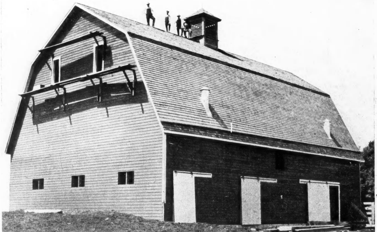
Gambrel Roof Barn of Self-Supporting Plank Frame Construction; Size 42 by 62 feet. Built Near Moosomin, Sask.
