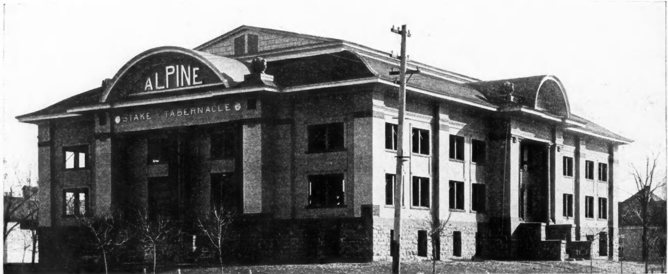
View of New Tabernacle at American Fork, Utah; Photo Taken Shortly Before Completion. Construction Superintended by J. H. Pulley.
