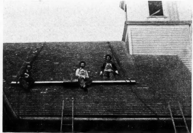
Holt and Lande Roofing a Church with Block and Tackle Scaffold.
