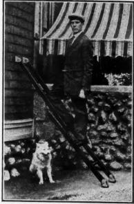
Friday. It is a suction foot grip that is placed on both ends of the ladder and is said to eliminate all the danger of slipping or sliding that happens quite frequently with disastrous results. The manufacturers say that this ladder can be used on a very steep angle on polished iron work, glass, stone work, concrete, or any smooth material, and that it will not slip even under these circumstances.
