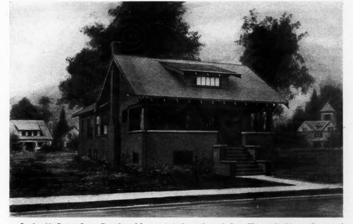
Comfortable Cement Stucco Bungalow of five rooms, 22 by 45 feet 6 inches. We can furnish complete set of blue-printed working plans and typewritten specifications for only \$6.00 per set. Blue-prints consist of basement plan; roof plan; main floor plan; front, rear, two side elevations; wall sections; and all necessary interior details. Specifications consist of twenty-two pages of typewritten matter. When ordering, ask for Design No. 6699.
