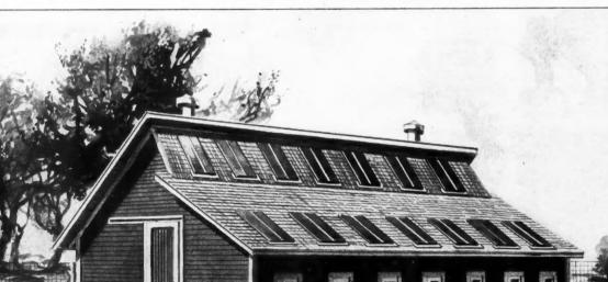
A Fourteen-Pen Winter Hog House, measuring 42 by 22 feet, of a modified saw tooth roof design to use the Sunshine windows, which are made with galvanized iron frames and sash. We can furnish complete set of Blue Printed Working Plans and Typewritten Specifications for only \$6.00 per set. When ordering, ask for Design No. A302.
