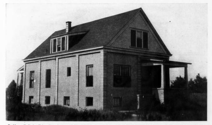
Residence Built by Using New System of Block Pilasters and Poured Curtain Wall Panels. A very pleasing architectural effect is produced.
