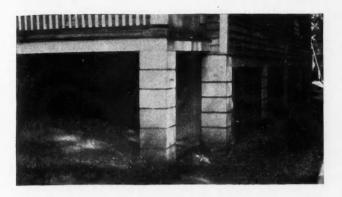
Foundation Construction of Block Pillars and Monolithic Panels or Curtain Walls.
