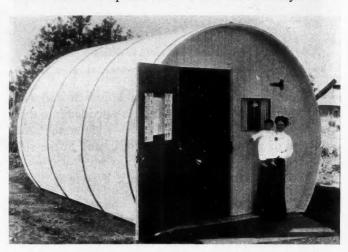
Garage Built of 2-Inch Tongue and Groove Staves, Secured by Four Iron Hoops. A Coming Garage Style in the Northwest.
