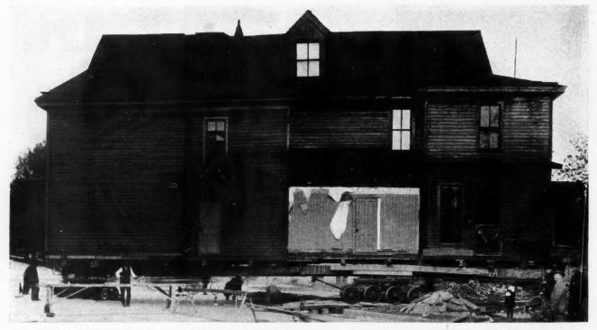
Fig. 5. Note the Springing of the Rear End of the Running Sills and Also that the House is Being Carried in a Straight Line. The Three Point Loading Combined with the Springing of the Running Sills Protects the House Against Racking.
