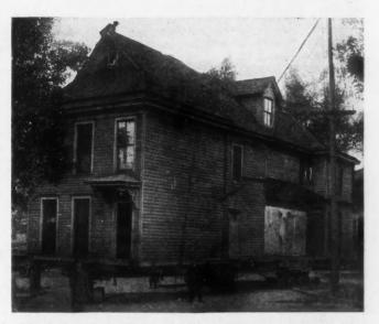
Fig. 4. Turning a Corner with House Mounted on Trucks. The House is Leveling Itself up as Shown by the Sag at the Right-Hand Corner.
