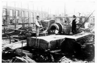
Charging Side of Mixer Used in Handling Mortar for Brick Work.
