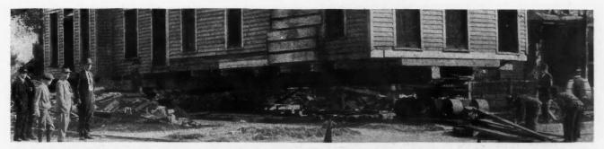
Fig. 2. Building Half Way Off of Its Foundation. The Track from Curb to Street Does Not Have to be Exactly Level as the Three Point Method of Loading Takes Care of This.
