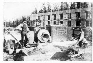
Discharge Side of "The Standard Mixer" Which is Handling Mortar Without Clogging.
