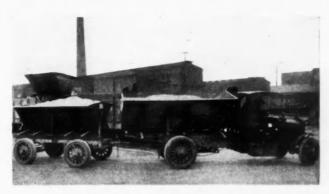
Heavy Trailer with Special Side Dumping Body for Handling Sand and Crushed Stone.
