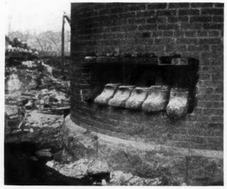
Fig. 2. Back Cut Away and Filled with Jacks.
