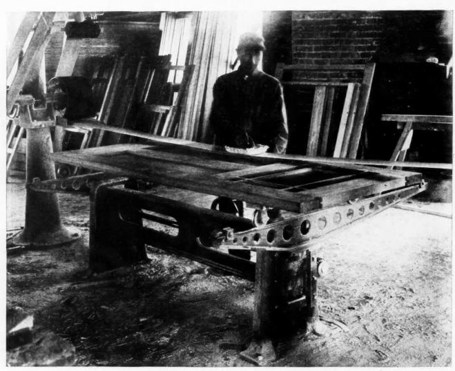
Finishing Stiles and Rails of a Door with the Yates Flexible Belt Sander.
