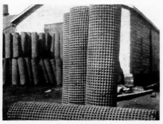
Showing Composite Metal Lath in Rolls Ready for Shipment This is a Combination of Wire and Brick Clay and is Made by Composite Metal Lath Co., 128 Broadway, N. Y.
