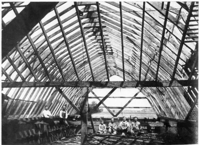
Trussed Frame Straw Barn Built Near Bradford, Ohio, by W. R. Inman. Tie Rods are Used Extending from the Plate to the Girders to Prevent Spreading, Each Rafter Forms a Complete Truss and Spans the 40 Feet Without a Purlin Plate.
