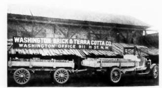
Heavy Four-Wheel Truck Used as Trailer and Loaded with Brick.
