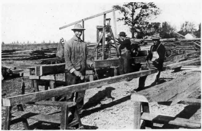
Homemade Boring Machine Mounted on Truck for Heavy Mortise Work on Timber Barn as Used by C. H. Toellner, Jr., Carpenter and Builder, Bunceton, Mo.
