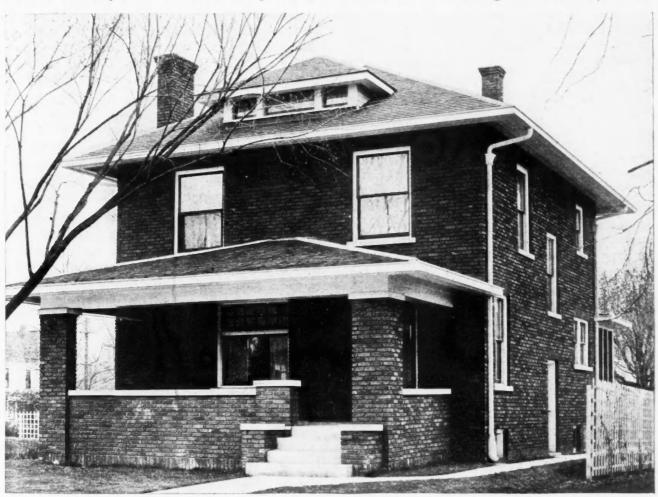
Photograph of Well Planned Brick Veneer House. Design No. 6857. This House, Requiring Twenty Thousand Face Brick, Has Been Built for \$4800. The Brick, Moderately Rough in Texture, Shows a Beautiful Play of Color Tones.
