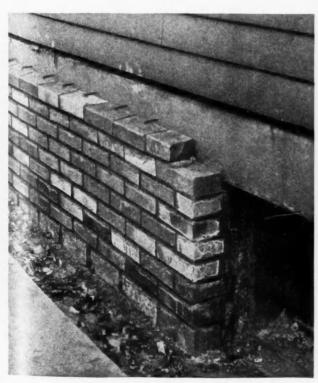
Method of Tieing Brick to Framework of House by Means of 10-Penny Cut Nails.
