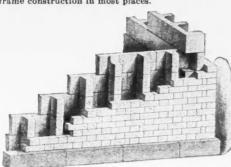
50 blocks, (100 sq. ft. of inner wall), made per hour, and laid in one-third the time required for brick.
