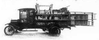
"Truckmobile" Unit Attached to Ford Chassis Makes Strong, Simple and Durable One-Ton Truck. Picture Here of Rig Loaded with Building Supplies Shows Extra Long Wheel Base of Truckmobile.
