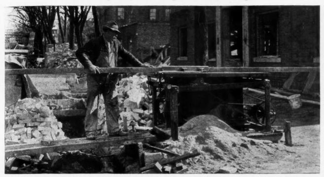
The Power Saw Rig Has Revolutionized Building Methods and Cut Down Costs on Every Building Large and Small.
