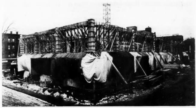
Showing How the Fred T. Ley Co., Builders, of Springfield, Mass., Protected the Fresh Concrete on the Overland Service Section. The Work Was All Done Last Winter During January and February, Much of the Time Zero Weather.
