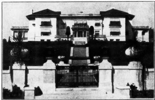
Residence of Mr. Hulett Merritt, Pasadena, Calif., an Example of Beautified Stucco.
