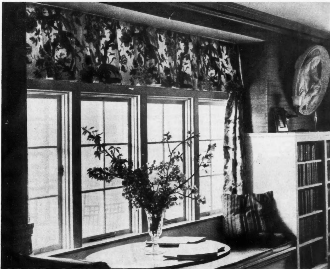
Four Outward Opening Casements in a Group with Transoms Above. The Grouping of Windows Increases Lighting Efficiency.
