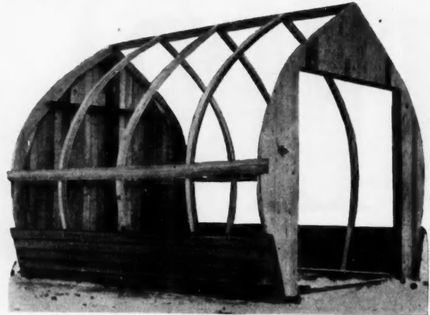
View Showing Framing of Small Gothic Roof Garage.
