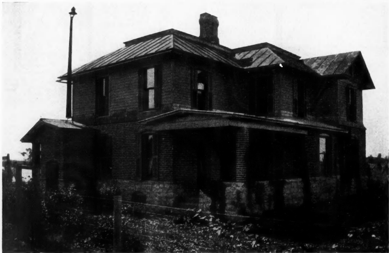
The Above House After Mr. Ford Had Overcoated the First Floor with Brick Above a Stone Foundation Wall.
