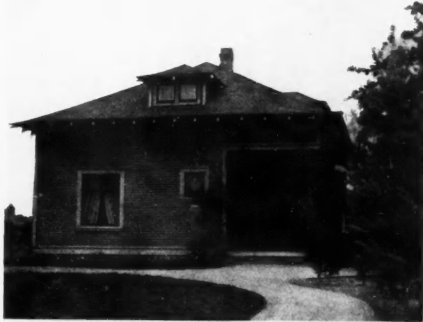
View of Bungalow on Which H. H. Mount, Pasadena (Cal.), Wishes to Build a Modern Brick Porch.
