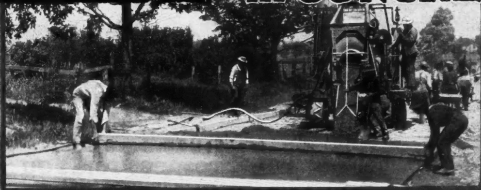
Rex Paver owned by George J. Markey, Milwaukee, Wis., at work on Milwaukee County Road.
