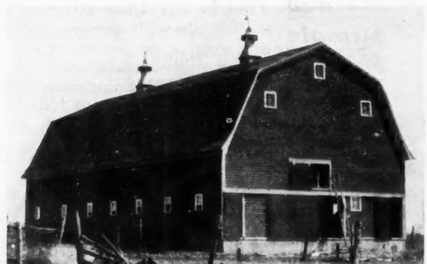
Well-Built Barn Erected During Last Season by E. H. Sheppard.
