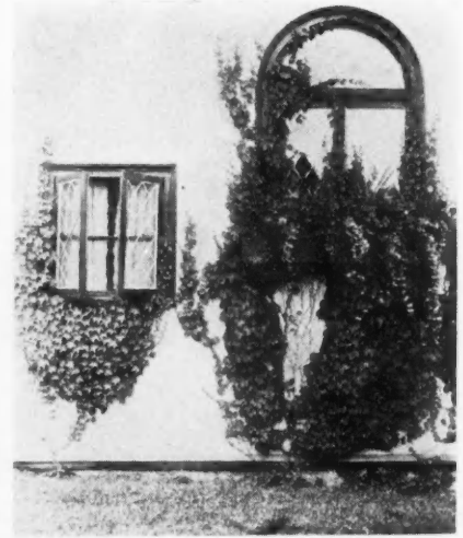
Casement Windows in Stucco Wall.
