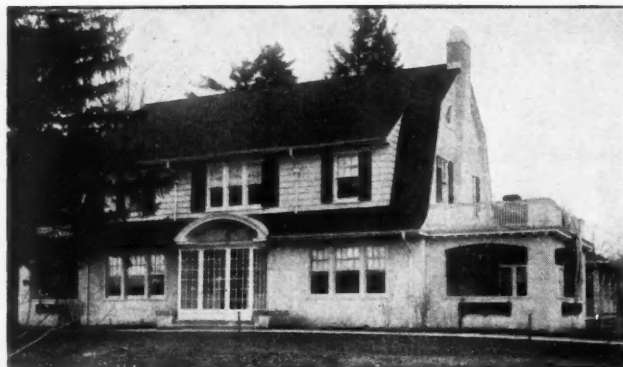
Architect, Edward C. Smith, Poughkeepsie, N. Y., for George I. Lumb. "Dixie-White" "CREO-DIPT" Stained Shingles on dormer side walls. "CREO-DIPT" moss-green shingles on roof.
