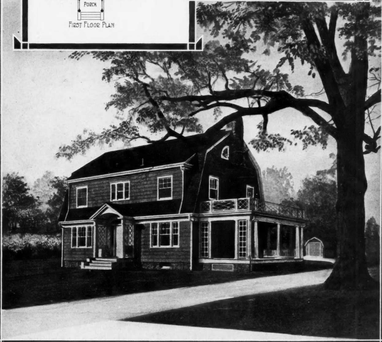
GAMBREL ROOF HOUSE WITH EXCELLENT ROOM ARRANGEMENT. This Dutch Colonial House is the Home of C. E. Bogardus, Stamford, Connecticut. It Was Designed by Frank M. Ellsworth, Architect. Attention is Called to the Arrangement of Rooms, Which is Excellent. Notice Especially That Each Bedroom Has Windows in Two Walls. Bedrooms are Entirely Independent of One Another. Size of House, 36 Feet by 25 Feet.
