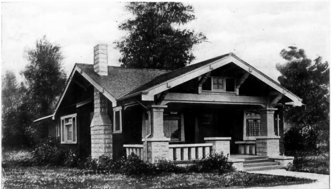
The Ornamental Details of This Little Bungalow Are Interesting. Concrete Has Been Used Effectively in the Porch and Chimney Construction.
