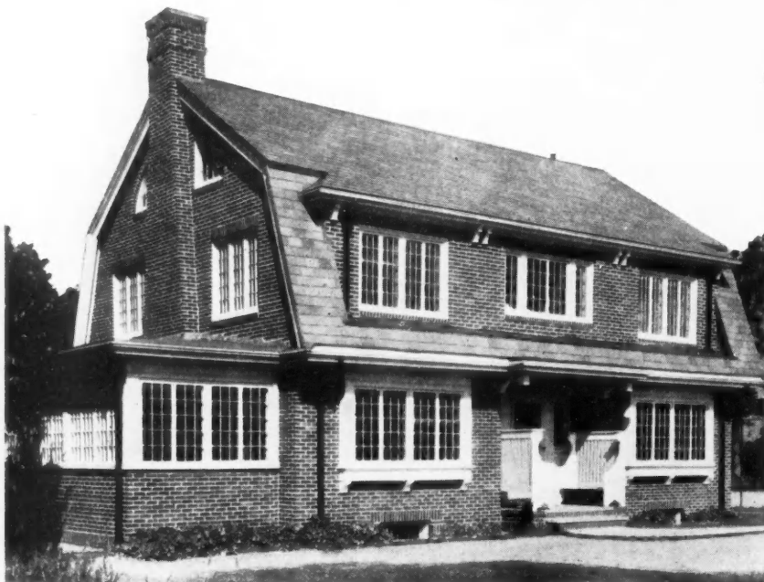
Distinctive Dutch Colonial House, Walls Built of Interlocking Channel Brick.
