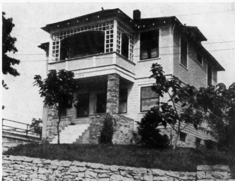
View of Remodeled House in Which the Original First Floor Has Become the Second Floor. A Family Continued to Live in the House While the Work Was Being Done.
