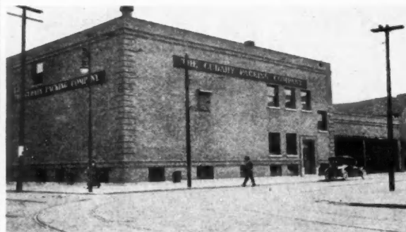
Cudahy Packing Co. Plant, South Chicago, Ruffner-Blos Co., Contractors, Chicago. R. T. Newberry, Arch. Working floors; below waterline foundations; walls and floors of cooler and dry storage rooms made watertight and waterproof with Medusa Waterproofing.
