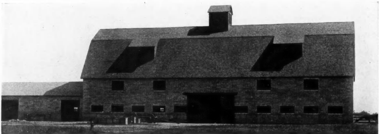
Horse Barn and Implement Shed of the Idaho Industrial Training School, J. T. Humphries, Superintendent, Anthony, Idaho. The Horse Barn is 120 Feet Long by 40 Feet Wide and the Implement Shed is 84 Feet Long by 30 Feet Wide. These Buildings and Several Others at the School Are Built of Concrete Blocks.
