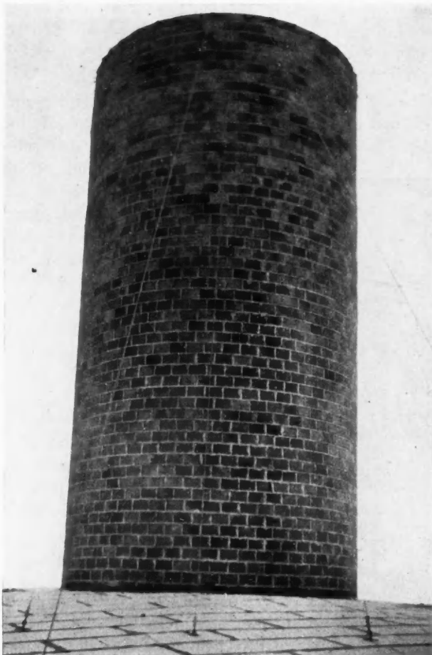
This View Shows Supporting Cables from Roof to Top of Silo.
