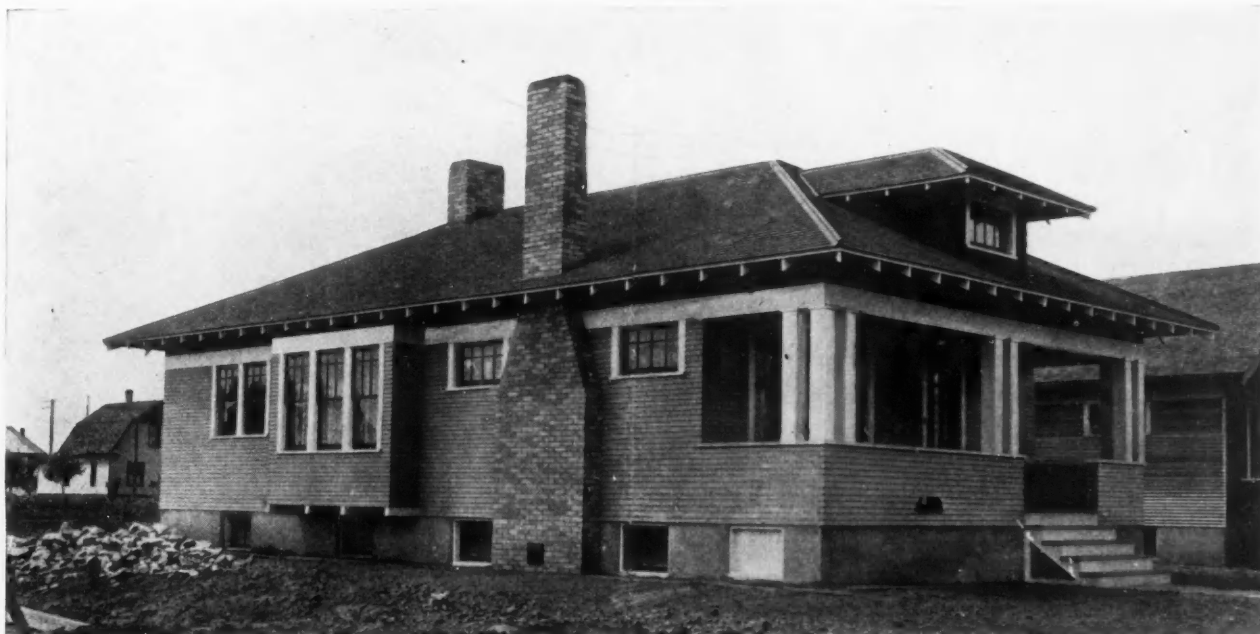
Perspective View of the Type of Bungalow Which G. A. Ensinger, Contractor and Builder, Has Found Popular in Bozeman, Mont.
