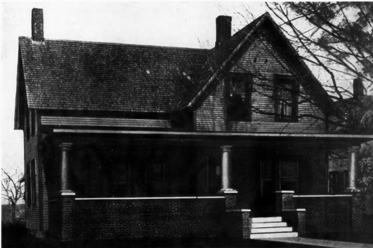
A Modern Face Brick Porch Entirely Across the Front of the House Shown Above Completely Transforms Its Appearance and Adds to the Comfort and Value of the Home.
