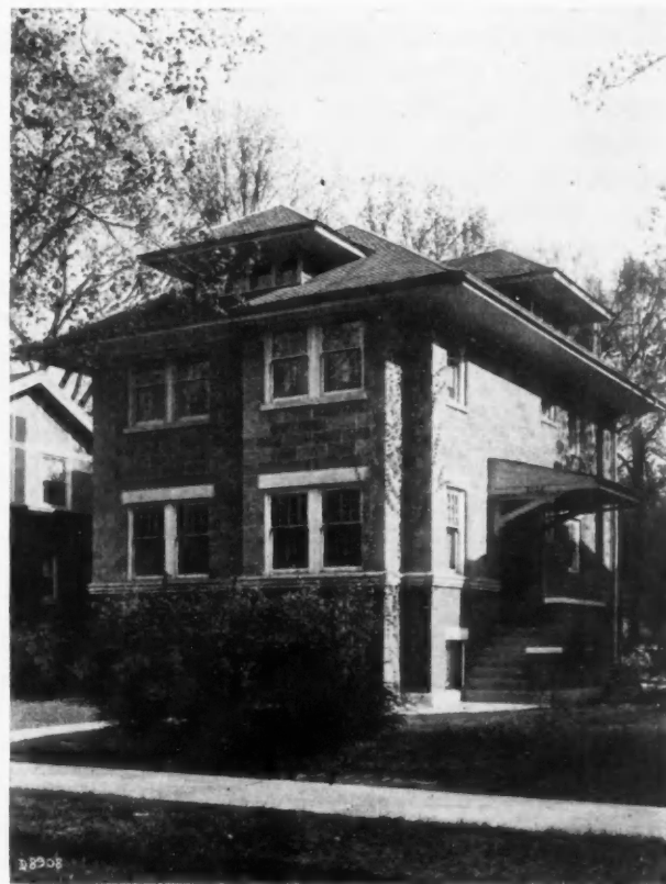
A Beautiful Small Residence Built of Concrete Blocks.
