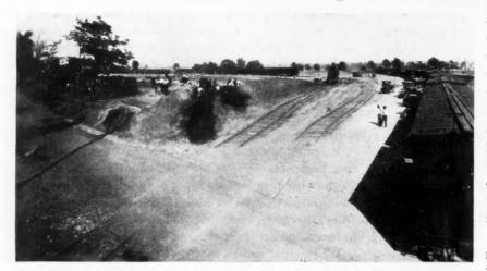
Railroad Tracks Are Run Directly Into the Cantonment so That Building Materials Are Unloaded From the Cars Right on the Building Site.
