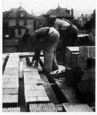
Placing Hollow Tile on 2 by 10-Inch Plank Centering. Note That Solid Centering Is Not Required.
