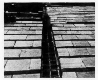
Combination Fireproof Floors Ready for 4-Inch Concrete Joists and 2-Inch Concrete Top Coat to be Poured. Note Bearing Partition of 10-Inch Tile Laid on End. A Layer of Building Paper Will Keep Concrete From Running Down.
