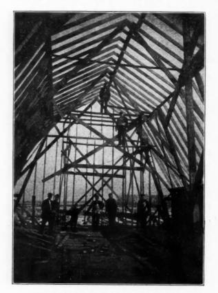
Fig. 2. Method of Framing Roof Timbers.
