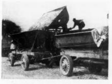
Materials Are Shoveled From the Car Into the Loader and Only a Few Seco Required to Load the Truck or Trailer.
