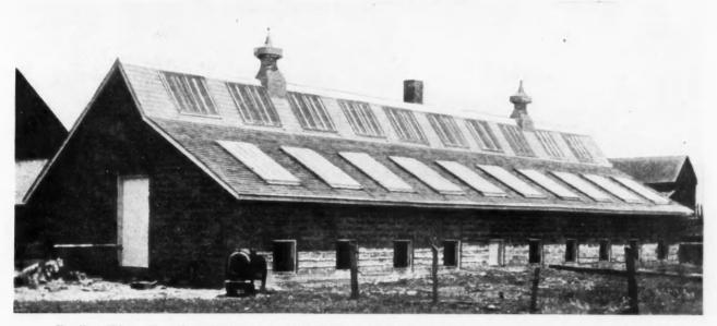
Excellent Winter Hog House Design of Concrete Blocks With Roof Windows and an Efficient System of Ventilation.
