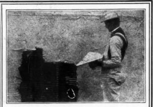
Plastering Rib Lath Note heavy scratch coat, due entirely to stiffness of Rib Lath
