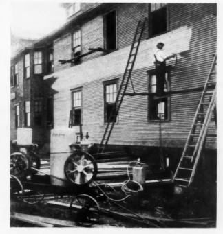
By the Use the Use of This Portable Equipment, Paint Is Forced Thru the Tubing and Sprayed on the Wall by Compressed Air.
