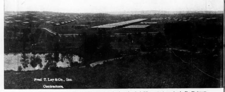
Panorama of Cantonment at Ayer, Mass., on July 31st, Forty-five days after the building contract was signed. The Workmen's Barracks-Temporary Quarters to House the Construction Gang-are in the middle distance. Note telephone lines from Construction Offices.
