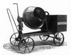
discharge any amount of concrete. The voke supporting the drum is of semisteel, molded in the form of an I-beam section with the metal distributed to give the greatest strength without unnecessary weight. Heavy
