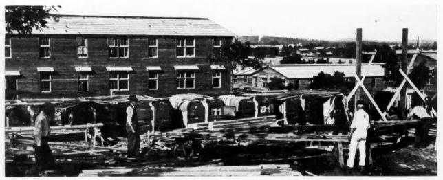
Boilers Have Been Erected in Open Complete, and Afterwards Have a Building Built Around Them. One Such Heating Plant Central for Each Unit or Regiment.
