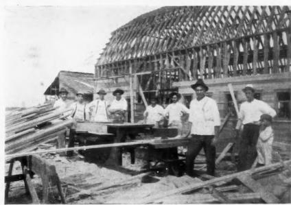
Contractor Ebert has a 4 h.p. Gasoline Engine and Woodworking Machine that He Takes Onto the Job. He Believes in Using Ali Labor-saving Equipment, Including Steel Scaffold Brackets.
