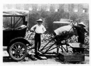
Auto Power Plant Operating Barrel Concrete Mixer.
