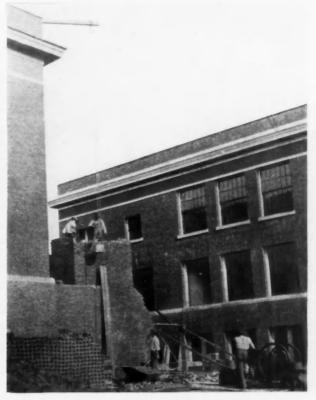
Reversible hoist used to great advantage by Contractor G. L. Smith, Waterloo, Ia., in constructing large brick chimney.
