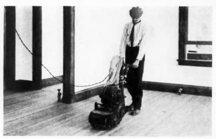
H. V. Demarest, Nyack, N. Y., saves time and labor, and makes money, using an electric power floor surfacer. One man and this machine surfaced a set of floors at a total cost of \$43.30, that would have cost for hand scraping at least \$475.00. Figure the gain yourself.
