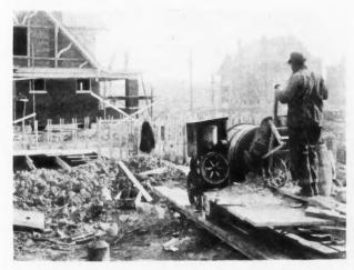
Concrete mixers have been perfected for builders' use. Note how convenient this loading platform is for charging the mixer by wheelbarrow. The mixer is often placed to discharge directly into the forms.
