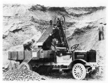
Sand and gravel can no longer be shipped in open cars. The contractors' answer to this rule of the Priority Board is to make more use of the neighborhood gravel pit. Here is a power loader and screen, loading a motor truck with torpedo sand. Materials from the local pit are OK, if cleaned and graded.
