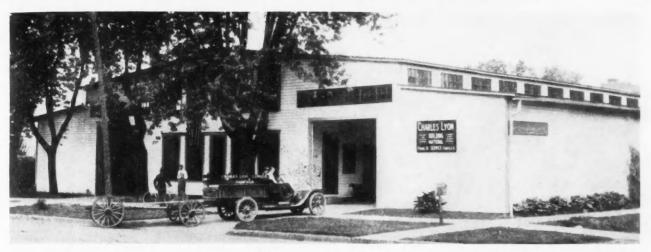
The Charles Lyon "Shed" Is a Low Monitor Roof, Double Driveway Warehouse, With Office and Display Rooms In the Middle at the Front. The Business-like Appearance of this Building Does Credit to Its Location on a Main Street of Fairfield, Iowa.
