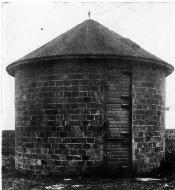
A Permanent Ice House on an Iowa Farm. Similar Buildings Are Used for Granaries, Root Storage, Etc.
