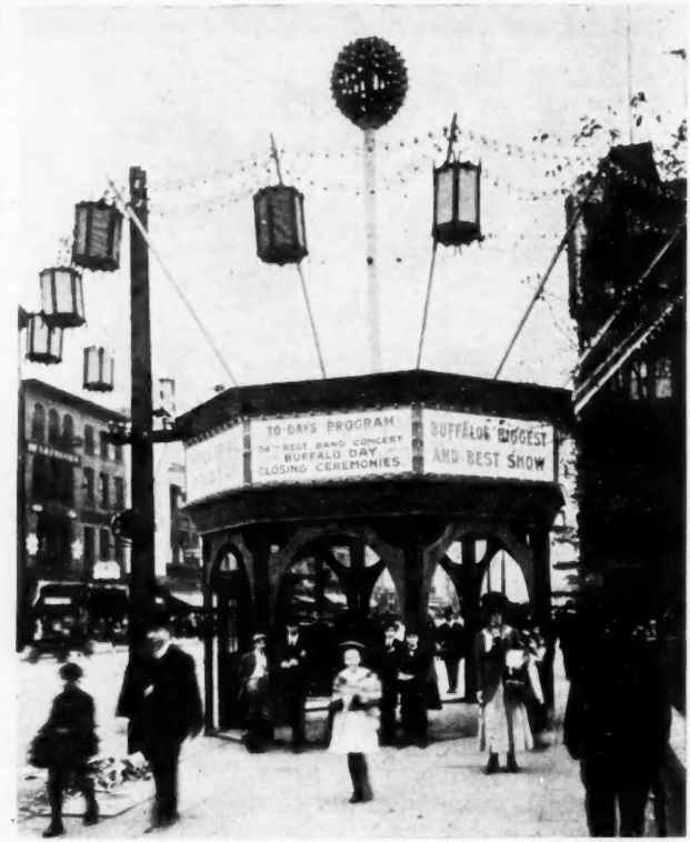
Wallboard Is Used for the Sign Panels of This Bandstand.
