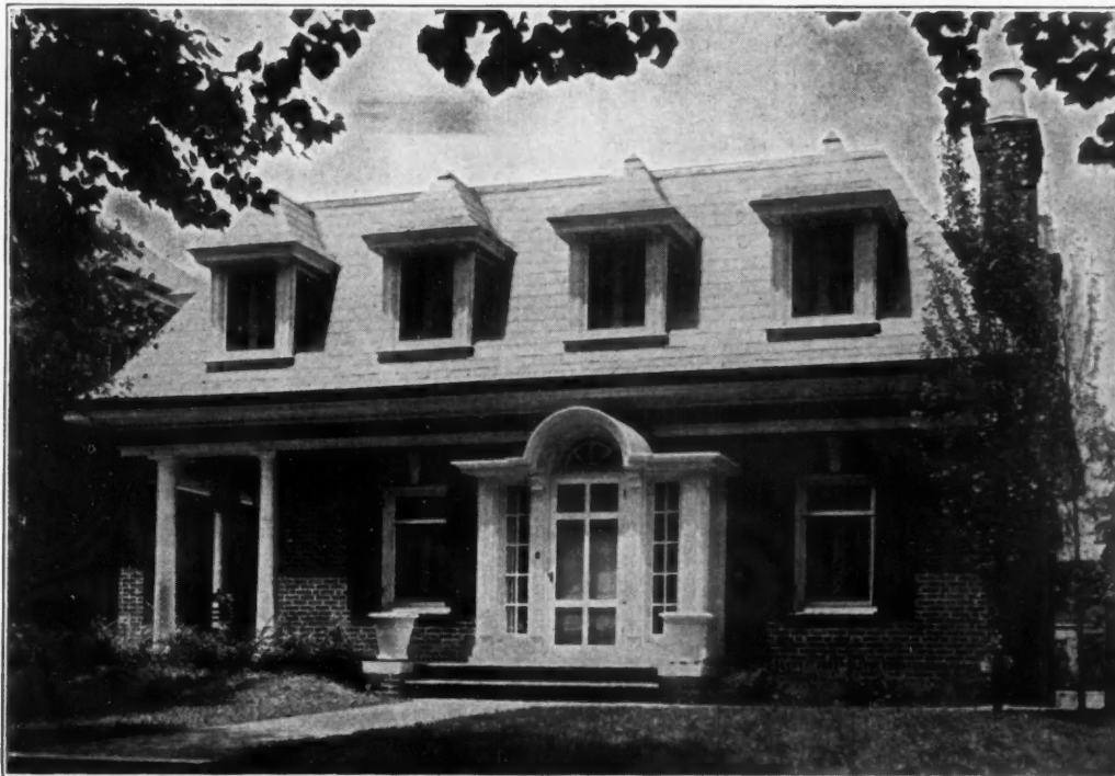
Maritz & Henderson, Architects
