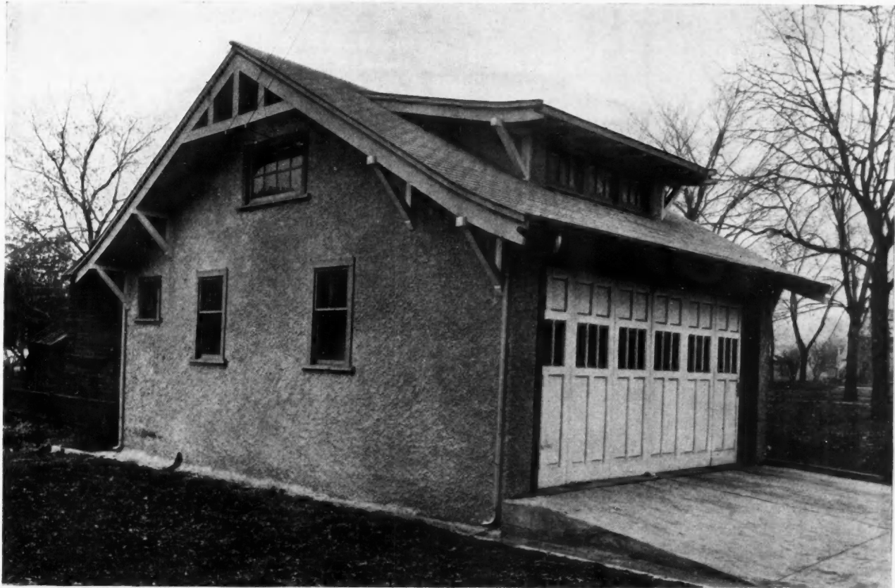
A Very Pretty Two-Car Garage of Hollow Tile, Stuccoed. The Doors Are Hung in Two Groups of Three Panels Each, Arranged to Slide Back Around the Corner Inside.
