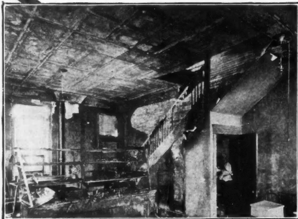
Rear section of store just after the fire. Note failure of plaster on walls.
