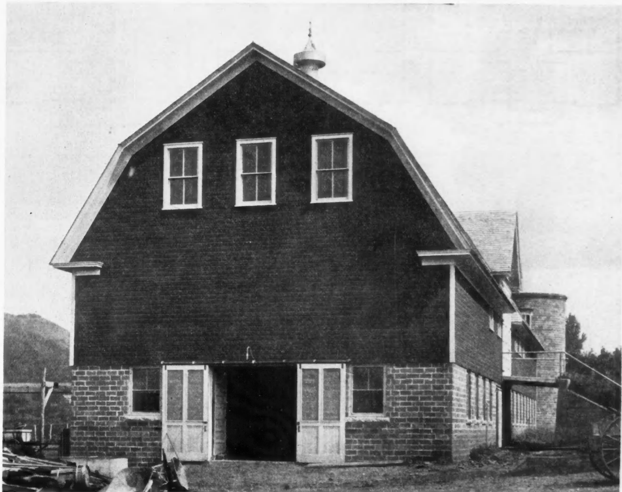
Tile Basement Bridge Barn at Briar Comb Farm, Winona County, Minnesota. The Stable Floor Plan Shown Above Provides for Thirty-eight Cows in a Barn 86 Feet Long.
