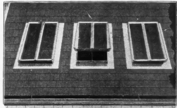
Sheet Metal Frames Are Self-Flashing.
