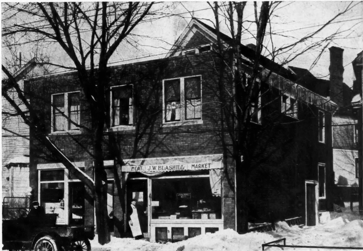
A Face Brick Veneer Front and Modern Show Windows Have Completed the Transformation of the Old Dwelling Into this Modern Store Building with Flats Above.
