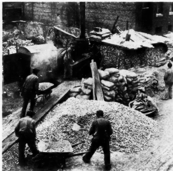
Concreting in Zero Weather at Ann and Lake Streets, Chicago.
