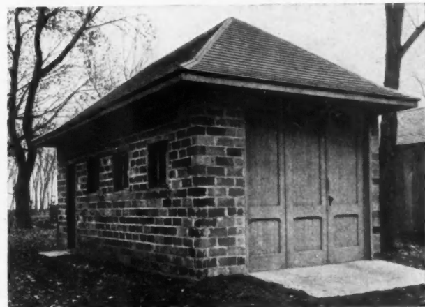
Photograph and Floor Plan of One-Car Tile Garage. The Variety of Coloring in the Tiles Makes a Pretty Wall.
