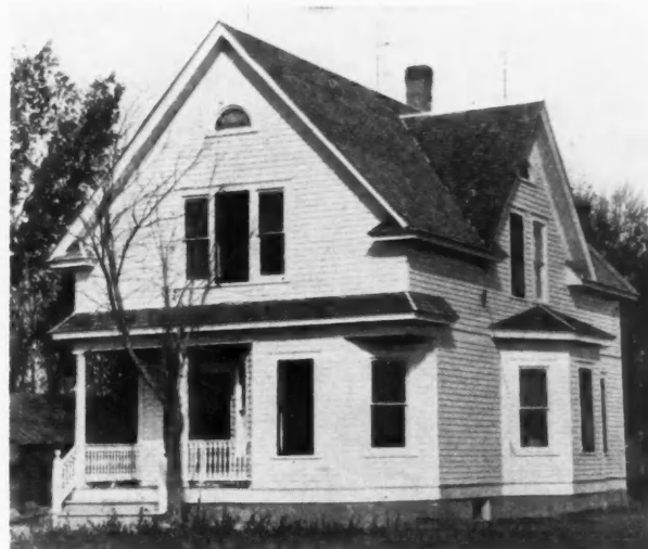
Modern Dwelling, Size 22 by 36, 14-Foot Studs Built at Walnut Grove, Minn., by Contractor Kregel.
