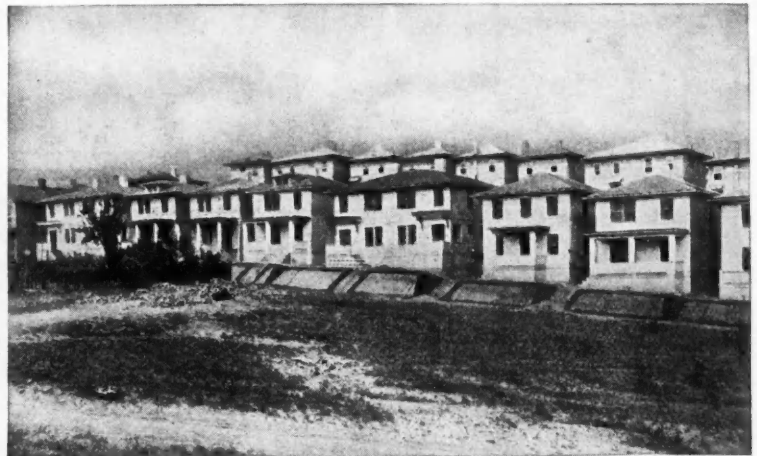
A Street of Concrete Homes Built at Donora, Pa.
