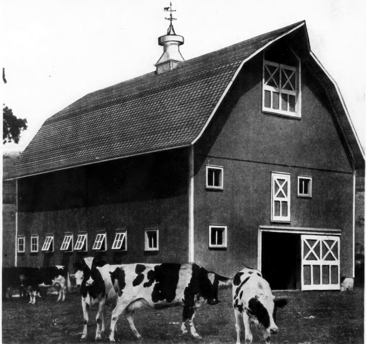
Barn for Twenty Cows Arranged to Face Out, so as to Drive Thru. Size of Barn Is 52½ by 32 Feet.
