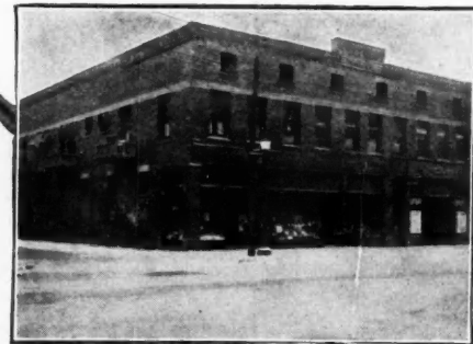
The Wild Building, Canton, Ohio. Fire originated in the rear of Nelson's Millinery Store—read Mr. Nelson's letter below:
