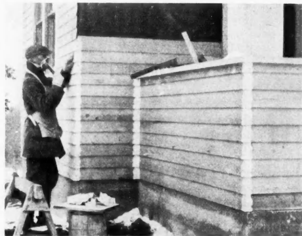
Metal Corners for Both Outside and Inside Corners Make a Neat Finish.
