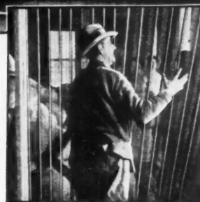
Self-Sentering partition Bower's Sanitarium, Lancaster, Pa.
