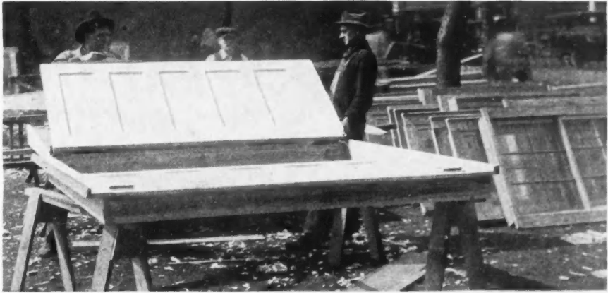
"Close Up" of the Manner in Which the "Fine Work" on the Doors and Windows Was Done in the Workyard so as not to Clutter up the Work of Construction. Gangs of Men Were Put at This Work at Seven, and by Ten had the Doors and Windows in Their Frames so that Each Unit Could be Carried to the Building and Quickly Nailed in Place.
