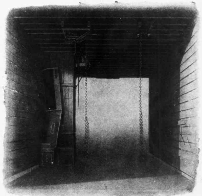
View Looking Thru Driveway, Showing Boot Folded up Out of the Way, and Hoisting Chains Let Down from the Ceiling to Slip Over the Front Wheel Hubs to Tilt the Wagon. Either the Platform Jack or the Ceiling Jack is Operated by the Same Power That Runs the Cup Elevator.
