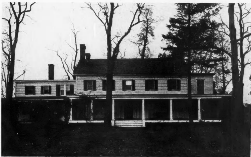
Residence of Maj. F. B. Barrett; Riverside Drive, Red Bank, New Jersey. Covered With 50 Squares Wide Space Asphalt Shingles Laid Over Old Wood Shingles.
