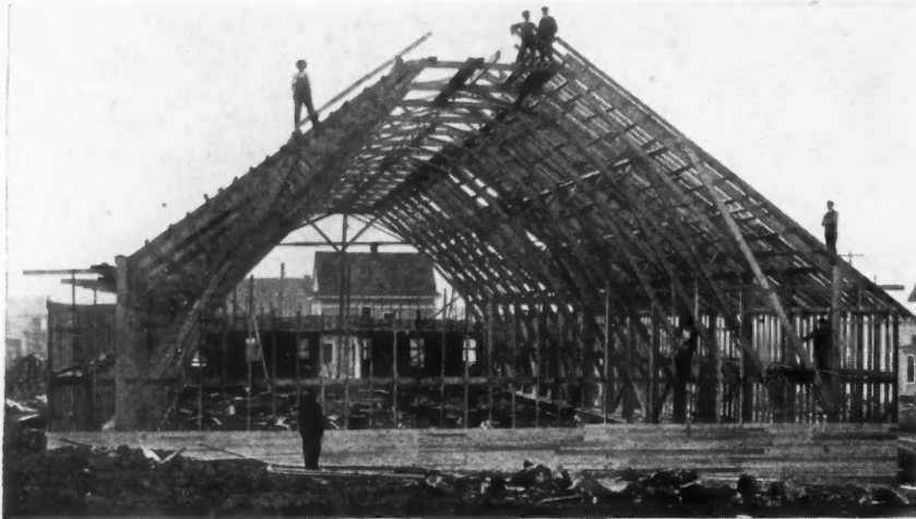
Frame Work for Skating Rink, 76 by 200 feet, at Campbellton, N. B.
