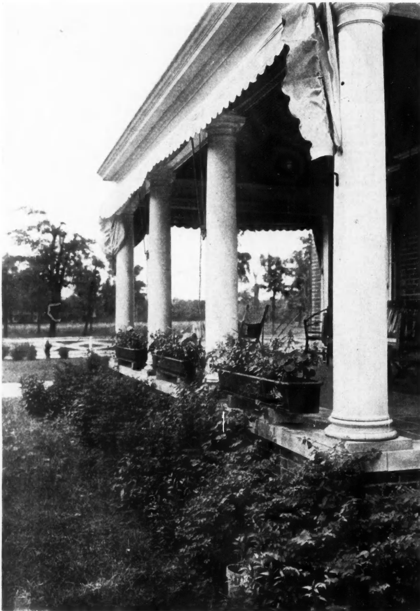
Comfortable Farm Home Porch in Illinois.
