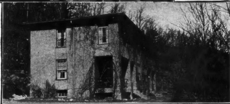
Twin House at Tuxedo Park, N. J. Built in 1907 with Metal Lumber and sided with Stucco on Berger's Expanded Metal Lath. ONE PHOTO WAS TAKEN IN 1907, THE OTHER IN 1918, COMPARE THEM.
