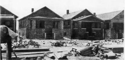
Four-Room Cottages of Tile Construction at Gary, Ind., Erected by W. L. Plew & Company. The Same Floor Plan as Shown on the Left is Used for All. Variety of Exterior is Gained by Having One Stuccoed, Another Faced with Brick, and a Third of Matt-Face Tile, etc.
