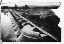
Multiple Arch Reinforced Concrete Dam, near San Diego, Cal.
