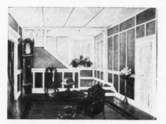
See complete plans and blue prints of typical Wall Board cottage, shown in the Industrial Housing Section opposite Page 34 of this issue. This Cottage uses Wall Board for Exterior Lining to take the place of Sheathing and also for Interior Finish of Entire House.
