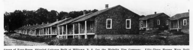
Group of Four-Room, Shingled Cottages Built at Milltown, N. J., for the Michelin Tire Company. Fifty-Three Houses Were Built Complete in 56 Working Days, by the John W. Ferguson Company, at \$1,125 Each.
