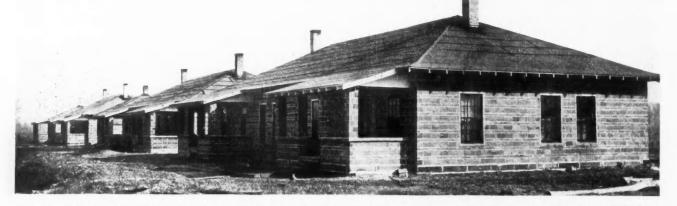
Row of Double Houses at Brazil, Ind., for the Employes of the Clay Products Company. Using Their Own Material—and It Is a Logical One of the Construction of Workingmen's Homes—these Houses are of Tile Construction.
