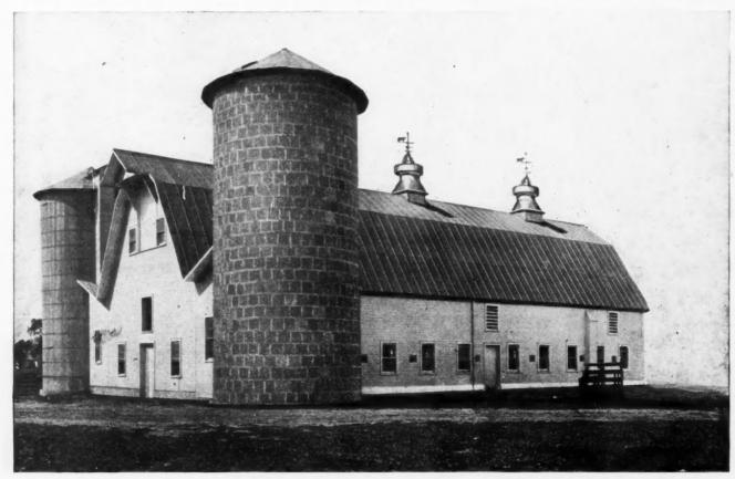
Photograph of Double-Silo Barn with Sheet Metal Roof. Size Is 36 by 64 Feet, Arranged to Stable Thirty-two Cows. Complete Plans for This Modern Dairy Barn Are Presented in the Blueprint Supplement Immediately Following.
