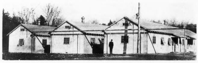
Where Company Dormitories or Bunk-Houses Are Wanted for the Unmarried Men, They Can Be Designed to Present an Architectural Appearance and the Interior Laid Out for Comfort and Efficiency Without Running Into Extravagant Expense. This Group of Three Double Dormitories, Each Measuring 100 by 21 Feet, Is Heated from the Central Steam Plant.
