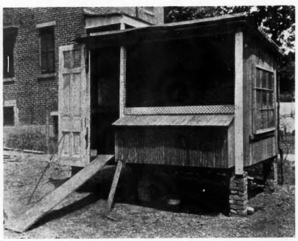
A Good Type of Open-Front Poultry House for a Small Flock. The Front Can be Closed with a Muslin Curtain on Cold Nights. The House Is Set on Brick Piers so as Not to Afford a Refuge for Rats. Notice the Nests Built Out on the Front of the House Where the Eggs Can be Reached by Raising the Hinged Cover.
