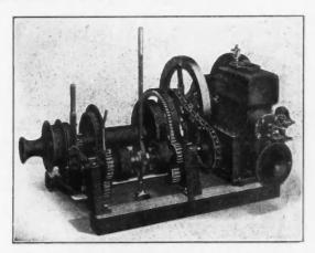
"American" No. 4 Hoist with Self-Contained Gasoline Engine. It can be made also with Electric Motor Built in, or arranged for Belt Drive.
