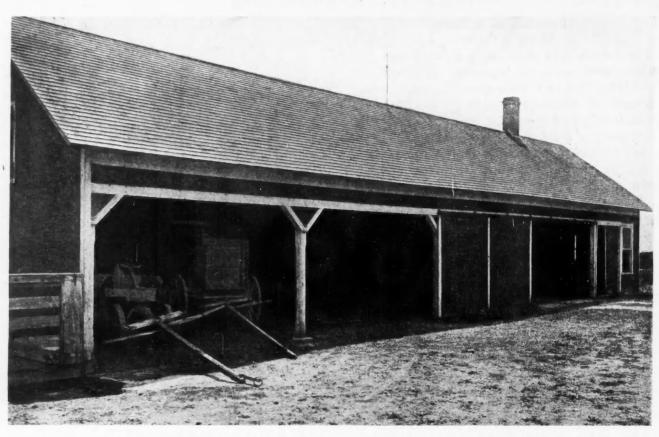
Here Is a Practical, Money-Saving Farm Building, Combining Implement Shed, Garage and Repair Shop. It Is 16 Feet Wide by 66½ Feet Long, Height 10 Feet to the Plates. The Space up Under the Roof Is Floored Over, Making a Dry Storage Space for Hand Tools, Farmer's Lumber Supply, Etc. The Shop in the Far End Is Equipped with Forge, so That the Farmer Can Take Care of a Good Deal of His Own Blacksmithing and Repair Work.
