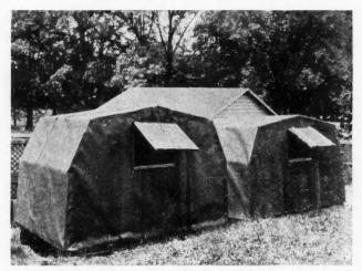
Rear View of Piano-Box Houses Shown Above. The Openings at the Rear Are Provided for Ventilation and Coolness in the Hot Weather. Windows Could be Used Instead of Solid Shutters and Would Make the Houses Lighter When Closed.
