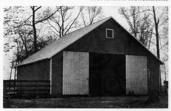
Inexpensive Implement or Carriage Shed, Size 28 by 30 Feet. It Should Have a Well Drained, Hard Packed Earth or Gravel Floor, and be Built Weather-Tight All Around.
