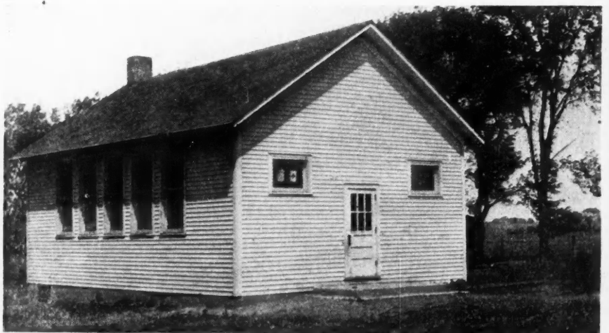
An Old School House Remodeled to Conform to the New Lighting Requirements.
