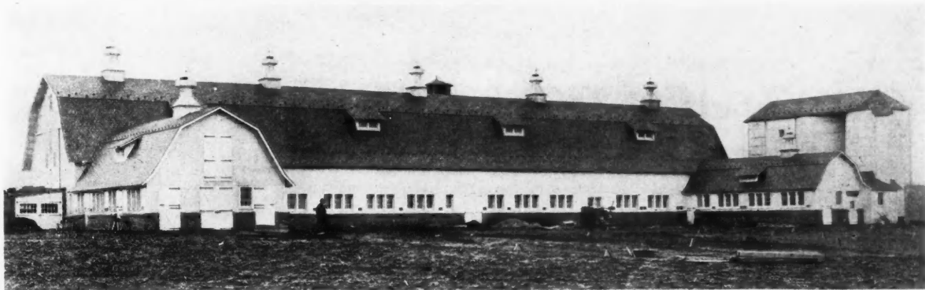
New Dairy Barn on Friends' Hospital Dairy Farm at Trevoze, Pa. Designed by James Manufacturing Company, and Built by William D. Bubeck, Carpenter and Builder, of Somerton, Pa.
