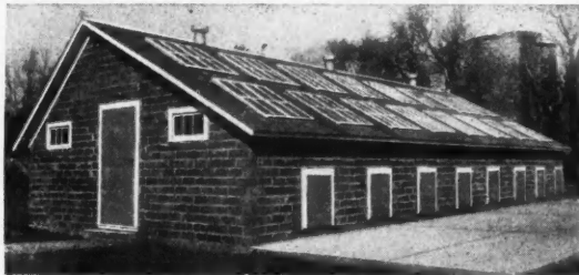
Hog House on Avondale Farm near Mason City, Iowa
