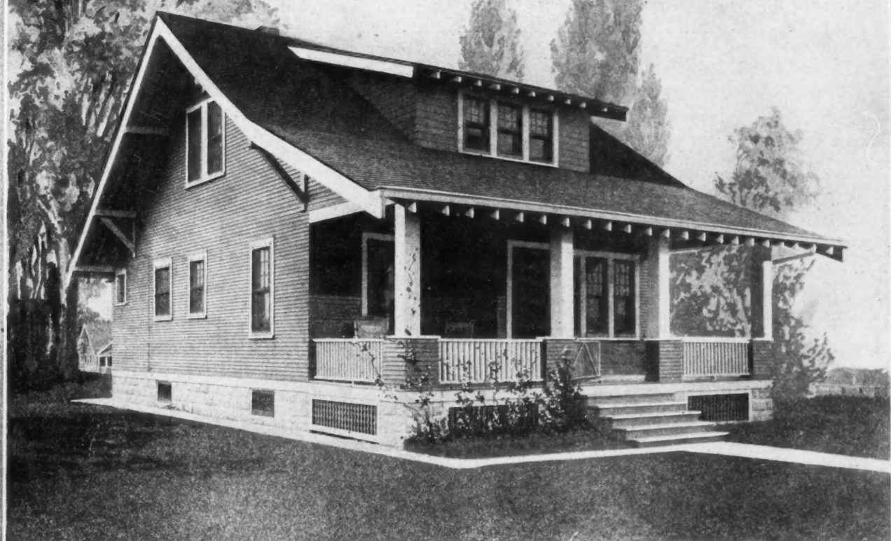
A PRACTICAL BUNGALOW OF SEVEN ROOMS. This design has the true western sweep with wide cornice, brackets and exposed rafters. Size, 28 by 28 feet. This plan shows four well arranged rooms on the main floor and three bedrooms and a large bathroom upstairs. The story-and-a-half style is well liked both for good looks and economy.
