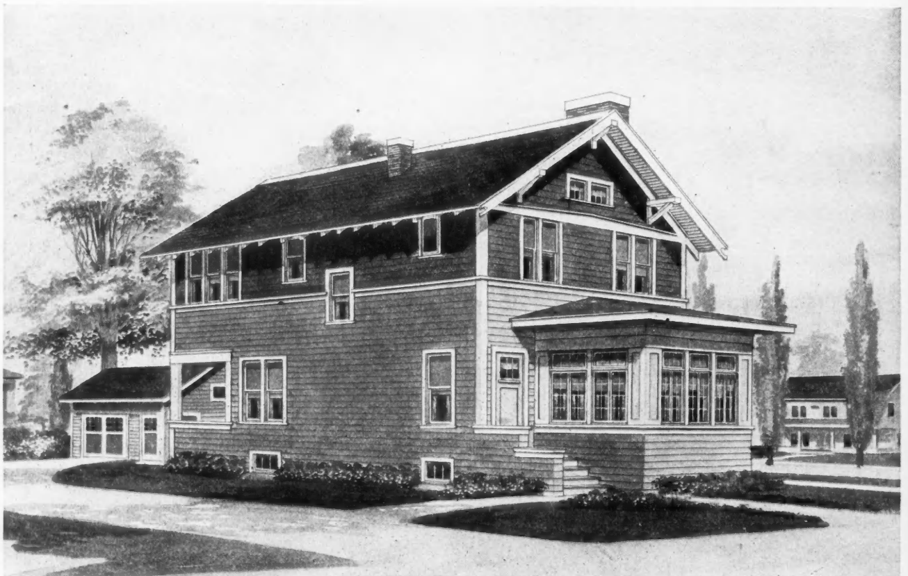
Narrow Lot Residence of Seven Rooms, Showing All Frame Construction. Alternate Exteriors in Brick and in Hollow Tile Stuccoed Appear on the Opposite Blue Print Page, and Working Plans for This House Are Presented.
