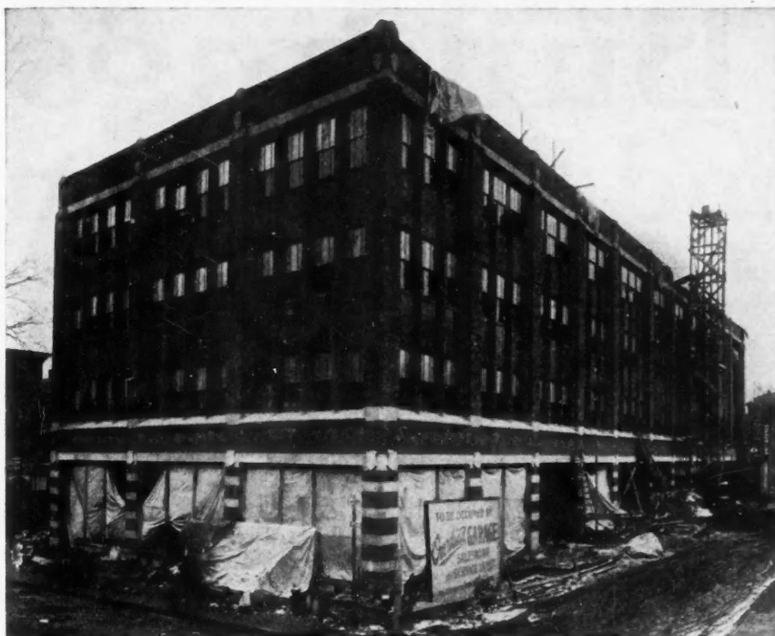
Exterior Completed on February 26th.
