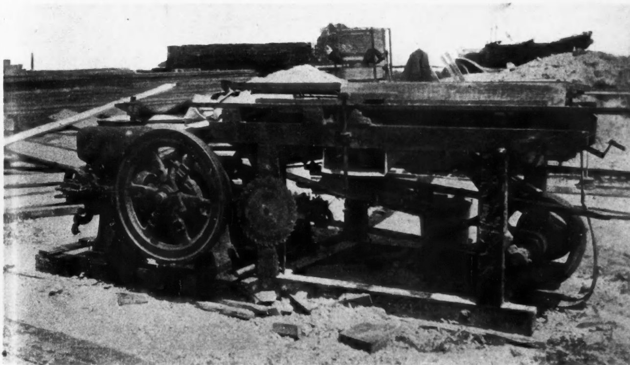
Power Saw Rig Built by Contractor Herman Erler, Rosemount, Minn., and a Great Labor-Saver on His Barn Building Work.
