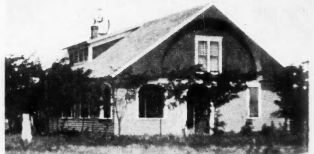
Bungalow Type of Farmhouse Built by J. J. Chlumsky, Near Timken, Kansas.
