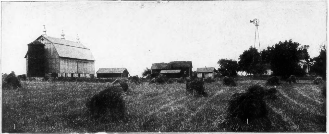
The Dairy Farm of Ben Thelan, Caledonia, Wis., whose barn is equipped with a complete ventilating system, which takes off excessive moisture and combustible gases.
