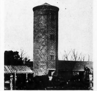
Vitrified Tile Silo of the Modern Type, Showing Tile Feed Chute and Masonry Roof.
