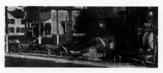
Mechanical Conveyor Taking Sand and Gravel to Paving Mixer.
