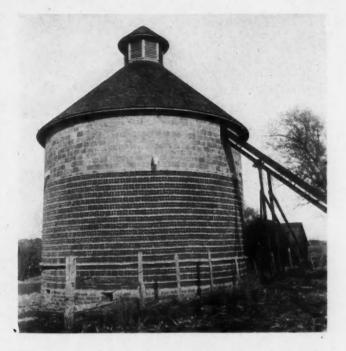
Circular Corn Crib and Granary of Vitrifled Clay Tile. The Tile for the Lower, or Crib, Section Have Pierced Holes for Ventilator.
