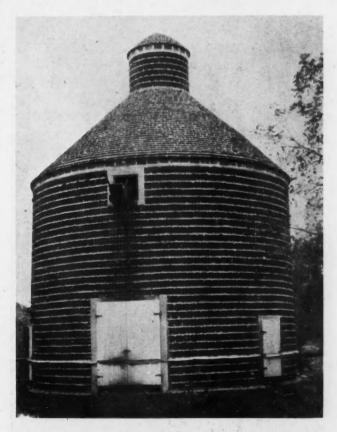
Circular Corn Crib of Vitrified Clay Tile, the Tile Being Laid with a Slope Downward and Outward. Three-fourths of the Wall Surface Is Open, Providing Perfect Ventilation. The Cone Spreader Distributes the Day's Husking Evenly.
