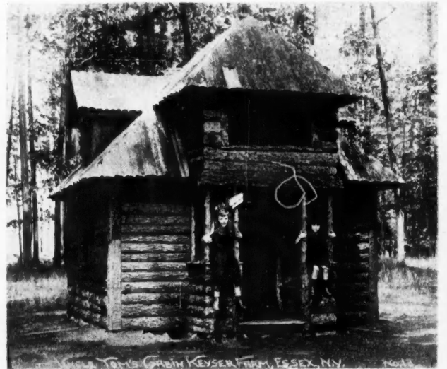
J. E. Murphy, Carpenter and Builder, Essex, N. Y., Built This Log Cabin Playhouse.
