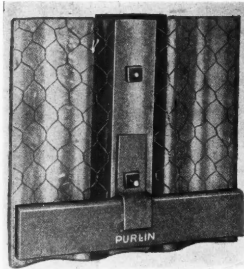
Iron Supporting Clip Fastens the Glass to the Purlins.
