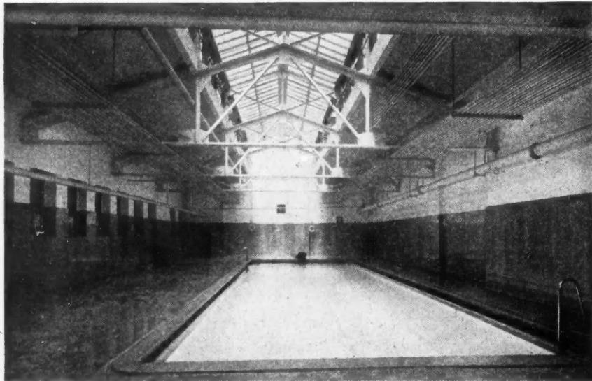
Interior View of Natatorium of the J. Sterling Morton High School, Cicero, Ill. The pool is regulation size, 24 by 60 feet, with distance markings, spring boards and ladders. Arrangement of heating system is especially noticeable, all pipes being overhead. All steel and metal work is white. The terrazzo floor has proper pitch to shed water into gutter outside pool curb. A filtration system is used and temperature of water is thermostatically controlled.
