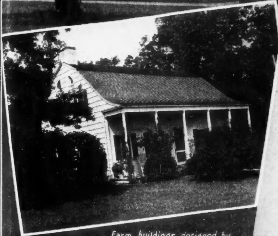
Farm buildings designed by ALFRED HOPKINS
