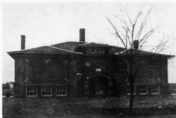
Houston School, Caldwell, Idaho, Erected by W. A. McGee & Son, of Specially Designed Buff and Brown Rough Faced Concrete Brick.
