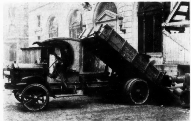
Smith Hauser & McIsaac, Inc., New York City. Contractors Use "White" Trucks with Special Dump Bodies to Deliver Materials to the Building Job. The Driver Seems to Like the Ease with Which He Can Dump the Load.
