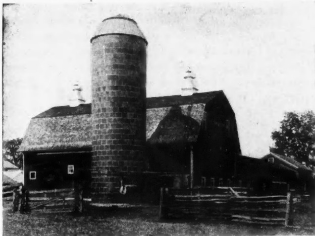
Vitrified Tile Silo on the Farm of J. M. Preston, Washington, Mich.
