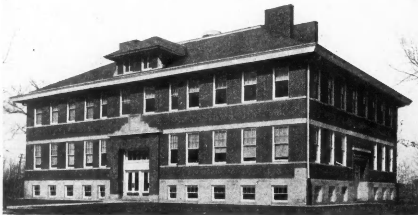
A Conservative and Economical School Building, the Central Grade and High School Building, North Chicago, Ill. Two stories and basement of stone and brick, with slate roof. Ashby, Ashby & Schulze, Chicago, architects.
