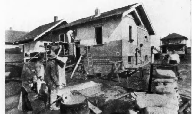
Stucco and Plaster Have a Strong Affinity for the Rough Surface of an Insulating Board Used as a Wall Base in This Building. The Strength of the Bond Is 200 Pounds to the Square Foot.
