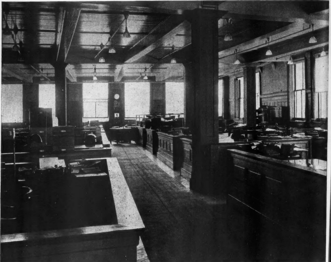
Compromise Between Private and General Offices. The Solid Partitions Give the Privacy, While the Large Open Space Allows Plenty of Light and Air, and the Whole Office Appears More Spacious.
