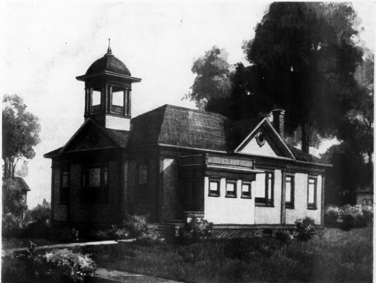
A Beautiful Village Church to Seat 354. Well Arranged Inside and Exterior Appearance Satisfactory. This Type of Public Building Is in Demand This Year.
