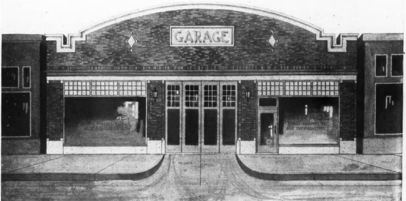
Front Elevation of a Public Garage of Brick and Terra Cotta. The Dimensions Are 50 by 100 Feet, Which Provides Space for a Good Many Autos, While There Is Room for a Supply Salesroom. The Building Is Fireproof Thruout and Is Especially Attractive.
