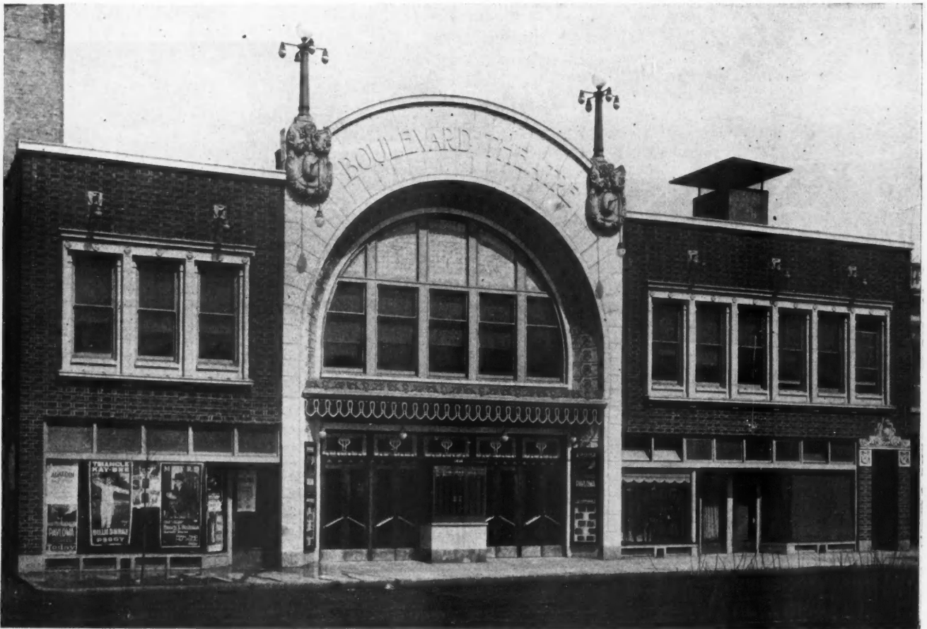
The Popularity of the "Movies" Has Brought Thousands of Good Jobs to Builders. Here Is One of Hollow Tile with Brick Veneer, the Type of Fireproof Construction That Is in Demand.
