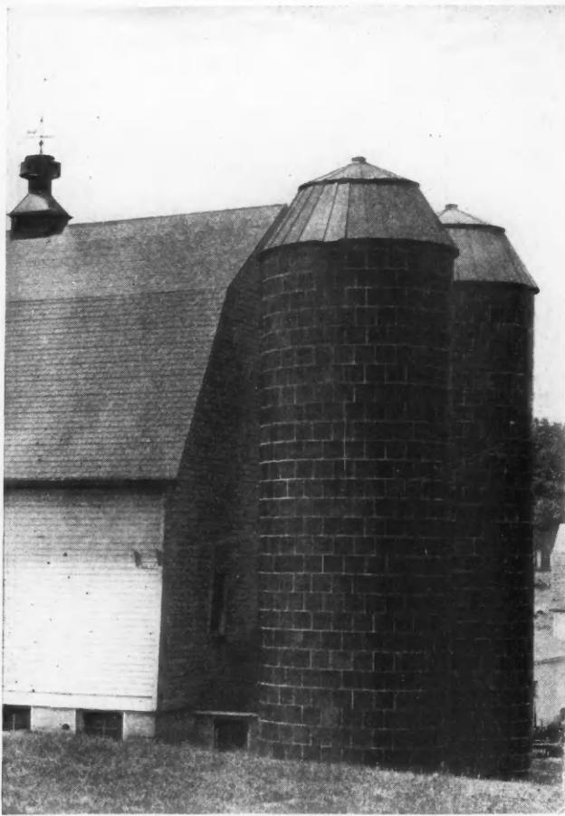
A Fine Pair of Hollow Tile Silos on the Farm of R. S. Olds, Grosse Point, Mich. These Silos Are 12 by 40 Feet.
