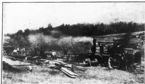
At Work in the Wood Lot.
