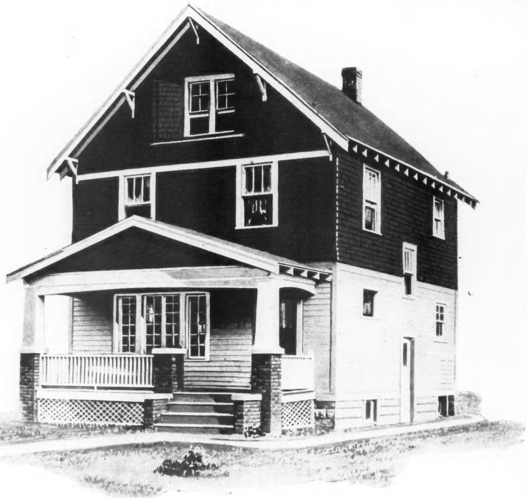
SIX-ROOM FRAME HOUSE. This Design Is Typical of the Homes Built at Firestone Park, Akron, O., a Large Industrial Housing Project that Was Begun Several Years Ago. The House Is of Frame Construction Set on a Concrete Foundation. Its Dimensions Are 22 by 26 Feet, and It Contains Six Well-Arranged Rooms and Bath.
