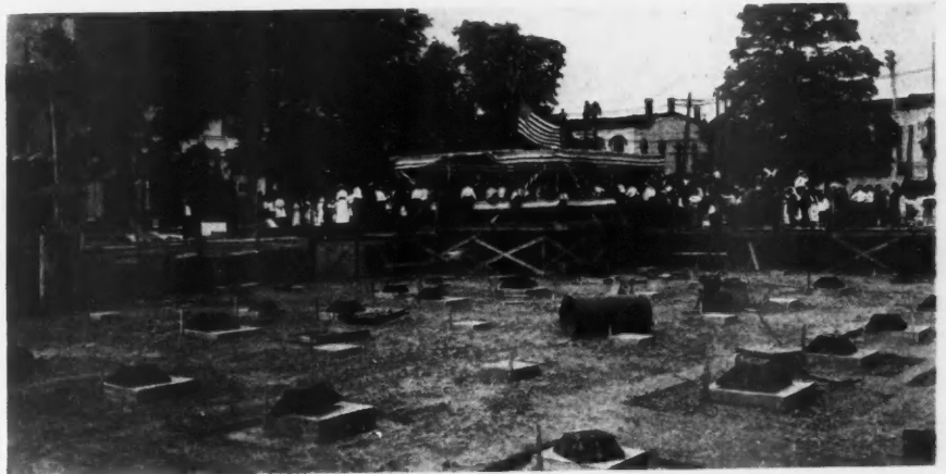
The Concrete Footings That Support the Madison County Court House, Edwardsville, Ill. The Photograph Shows the Ceremony Attending the Laying of the Corner Stone.
