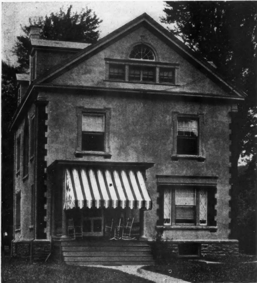
The Brick House After It Had Been Overcoated with Stucco. Note the Corners Where the Brick Have Been Retained as Exterior Trim.
