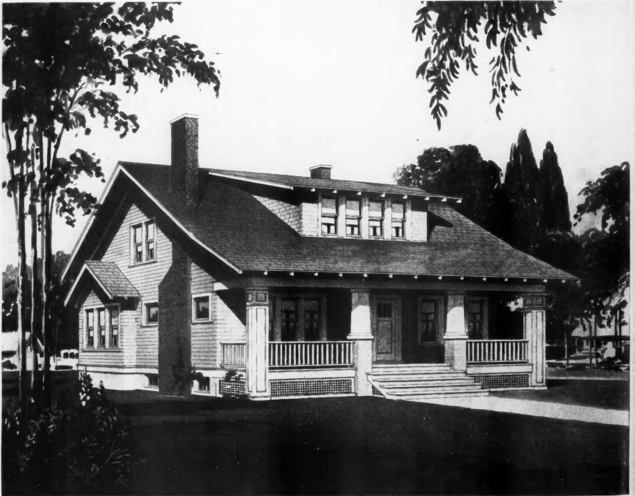
SEVEN-ROOM BUNGALOW TYPE RESIDENCE. This Story-and-a-Half House is a Beauty and of the Sort that is in Great Demand. Its Dimensions are 36 by 28 Feet. The House contains Seven Good Rooms, Four on the First Floor and Three on the Second.
