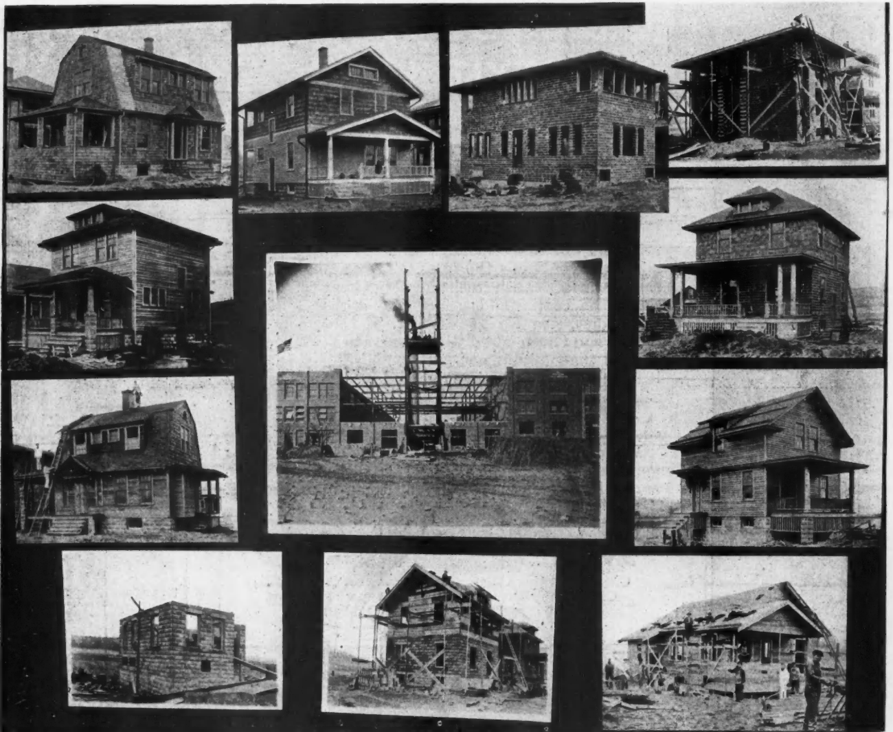
INDUSTRIAL HOUSING PROJECT, FORT MADISON, IOWA. Beginning at the Top, Left to Right—Six-Room Dutch Colonial; Six Rooms of Frame and Shingle Construction; Hollow Tile to Be Covered with Gray Stucco; Hollow Tile to Be Covered with White Stucco; Six-Room Frame House; Hollow Tile to Be Covered with Shingles on Upper Floor. Center Picture Shows Office Section of Tire Plant, Sprinkling Tank Tower, and First and Second Units of the Plant. Five-Room Dutch Colonial and Five-Room Frame House. Bottom Row—Six-Room Home of Brown Rough Face Cement Block with Stucco on Second Story; Five-Room Bungalow and Panel Face Concrete Block House of Five Rooms.
