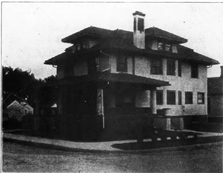
The Stucco on This Home Was Applied When the Temperature Was 16 Degrees Below Zero and After Four Years Shows No Cracks and Is in Perfect Condition. The Home Is Owned by Charles Petry, Marshall, Mo. F. H. Knelsley, of Marshall, Was the Architect.
