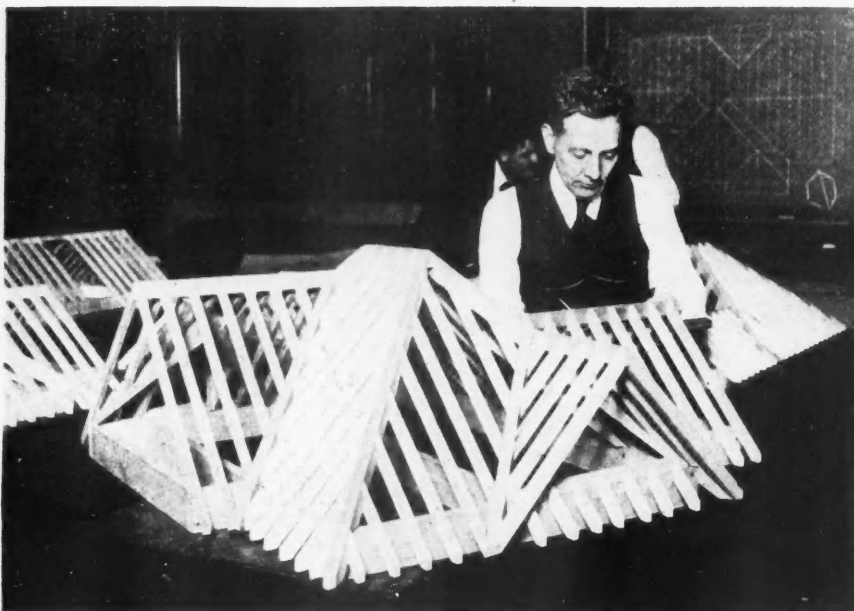
Fig. 1. A Model Roof Laid Out with a Steel Square at the Pratt Institute. The Diagram of the Roof Frame Is Shown on the Blackboard.
