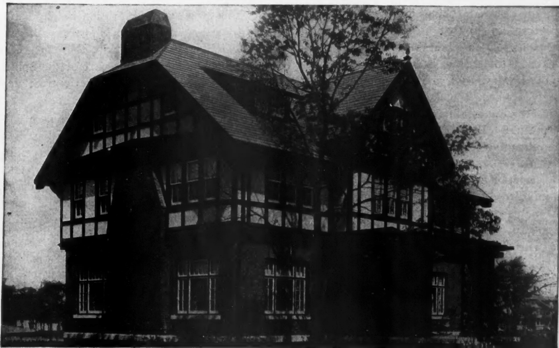
Roof covered with Ambler Asbestos Shingles (Century Brand)—American method. Upper sidewalls covered with Ambler Asbestos Building Lumber—Half-timber effect.
