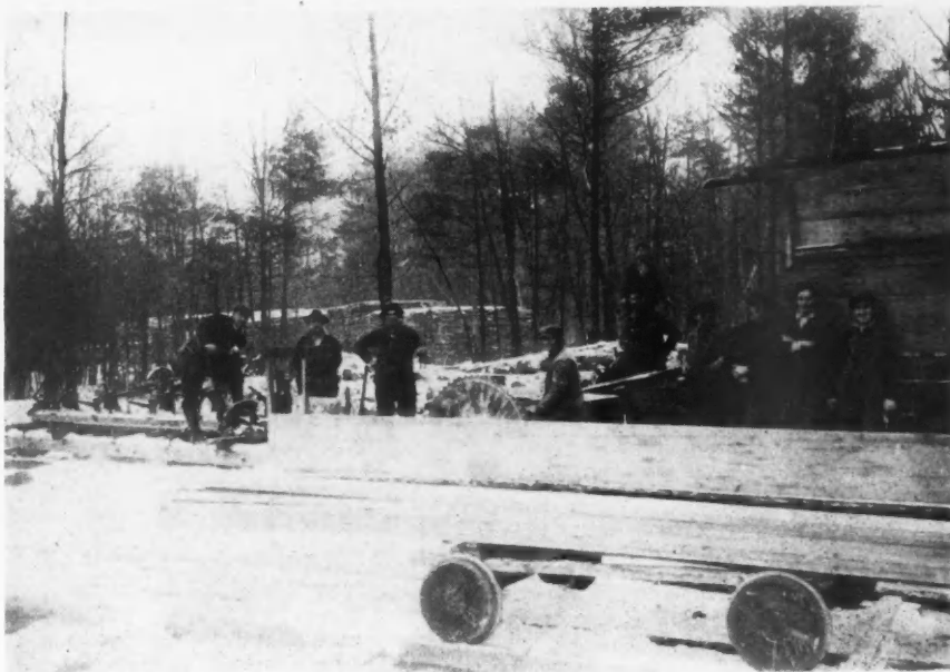
A Close-Up View of the Portable Saw Mill. Wooden Tracks Are Laid Where There is Much Timber to Be Cut and Sawed and the Lumber Is Carried to the Pile.
