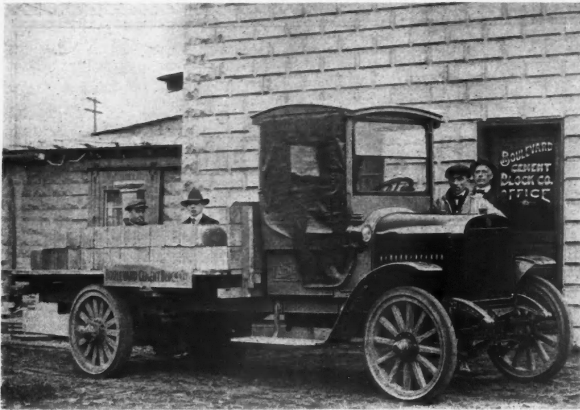
The Boulevard Cement Block Co. Has a Special Body on Its "Acme" Truck for Hauling the Concrete Blocks It Makes.
