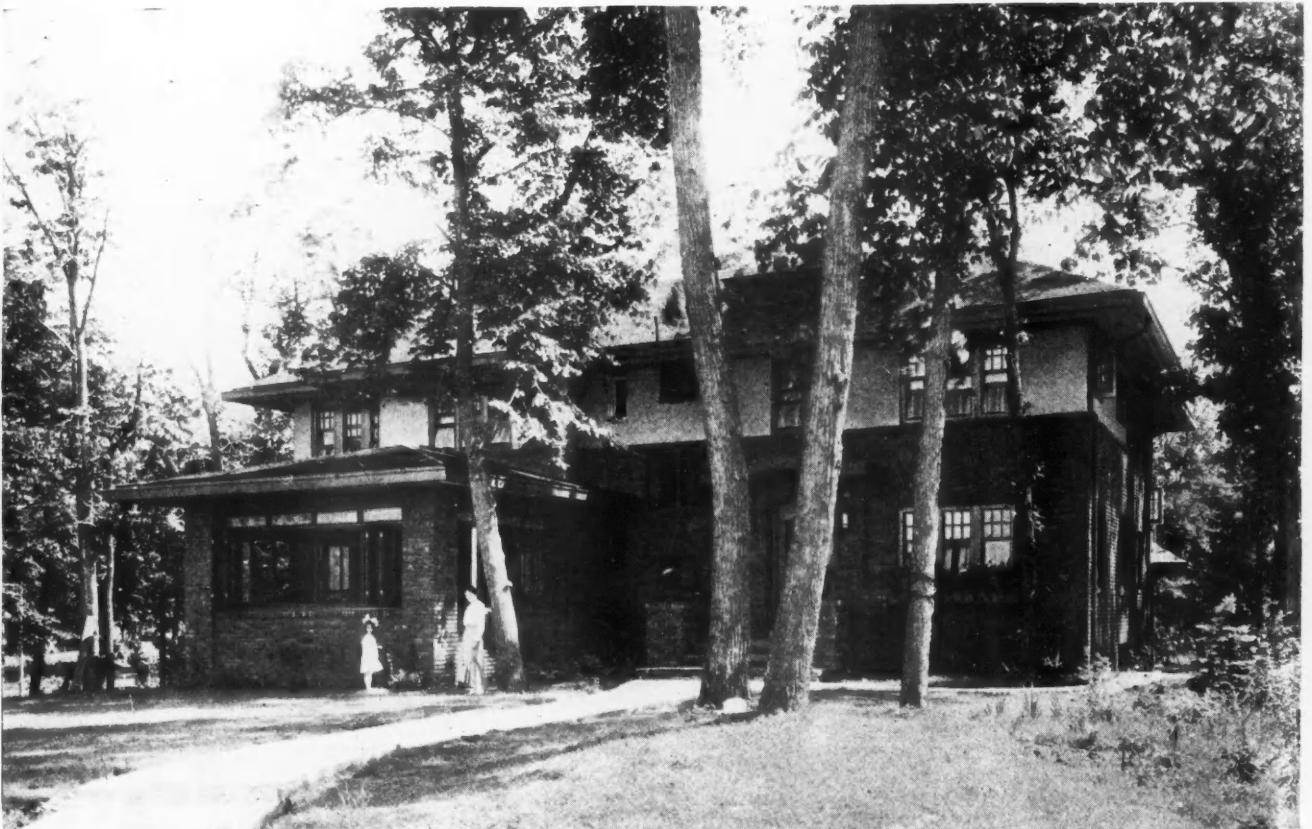
A FINE EXAMPLE OF THE USE OF FACE BRICK. Note How Effective the Exterior of this House Has Been Made Through the Use of Face Brick, With a Strip of Stucco Under the Roof Projection. For Large or Small Houses Face Brick Over Solid Brick, Hollow Tile or Frame Construction Makes an Attractive Home.
