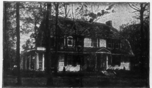
Stained with Cabot's Creosote Stain C. M. Hart, Architect, Bay Shore, N. Y.
