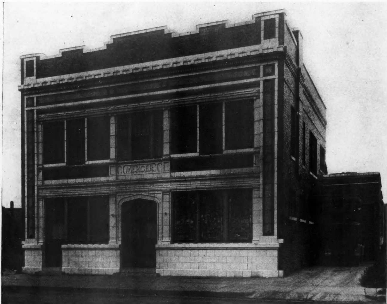
Two-Story Modern Business Building with Basement. Size 50 by 125 Feet, Brick and Terra Cotta Construction. Building Contains Complete Undertaking Establishment on First Floor, Consisting of Salesroom, Chapel and Garage, and Has One Apartment on the Floor Above. The Morgue and Embalming Room Are in the Basement. The Garage Is Large, for the Automobiles and Undertaker's Needs.
