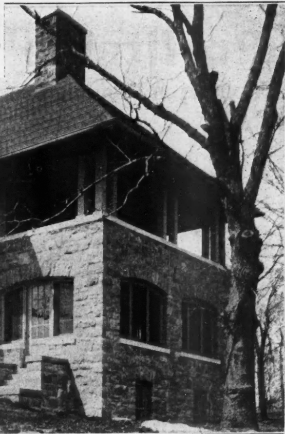
Residence of Prof. Geo. B. Pegram; built in 1913. Berlov Metal Lumber was used in floors and bearing partitions. William B. Claflin, the architect, member American Society of Civil Engineers, after an inspection, reports:
