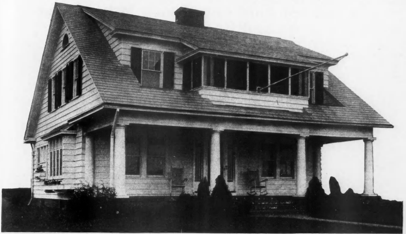
MODERN SEVEN-ROOM FARM HOME. Here is an exceptionally good farm home building design. The house is 23 by 36 feet and contains seven rooms. The living and dining rooms, den and kitchen are on the first floor, and three bedrooms and bath on the second. The arrangement of the rooms is shown by the plans on page 115. The basement plan shows the location of the pipeless furnace and the modern laundry equipment, which go far toward making life on the farm more worth the living.
