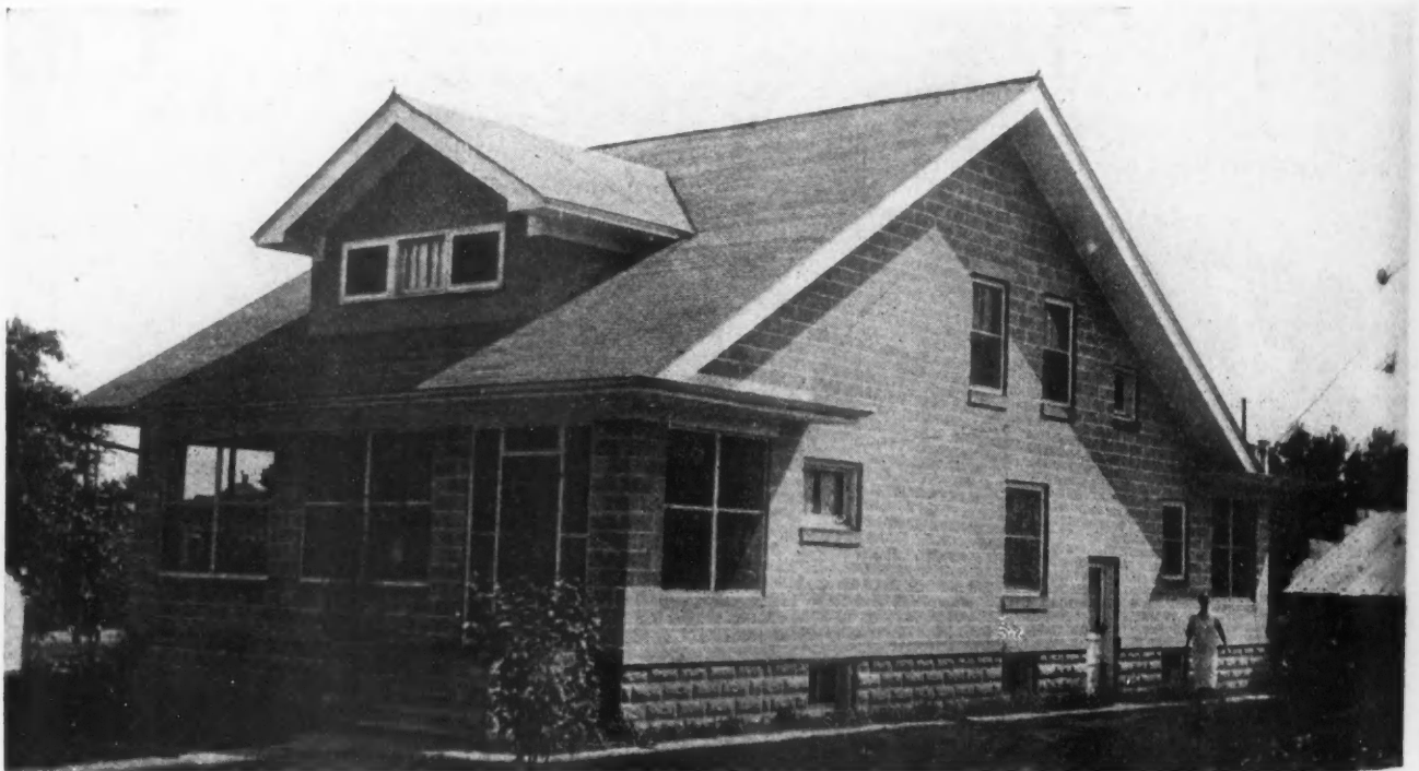
A COZY SEVEN-ROOM HOUSE OF CONCRETE BLOCK CONSTRUCTION. This building with its large comfortable screened porch is 26 by 32 feet.
