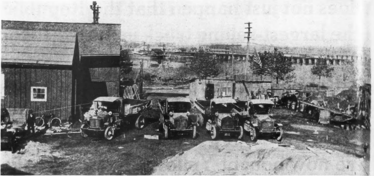
Four of the Six "Pierce-Arrow" Trucks of E. C. Humphrey, Contractor, Hackensack, N. J. Using Six Trucks, Mr. Humphrey Hauled More Than 500 Tons of Material a Day for 200 Days, Making a Record for Speed on Road Construction Work.
