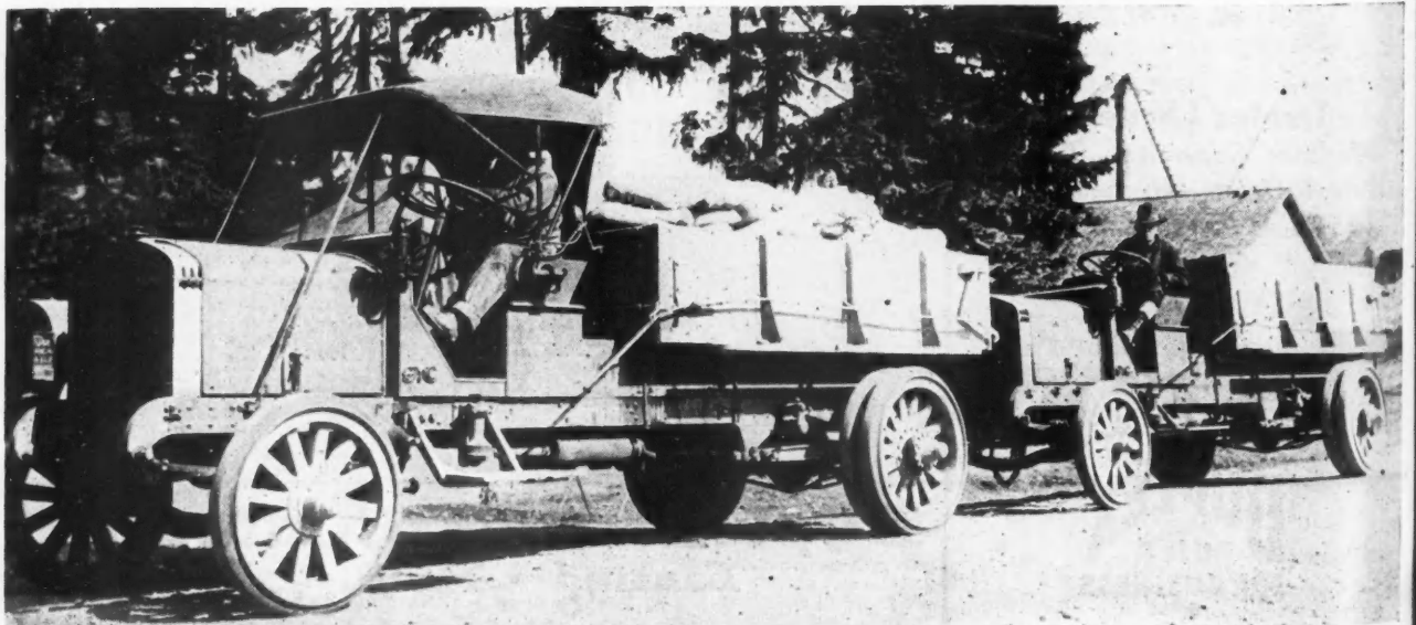
Hauling Cement to the Rural Building Job. Here Are Two "GMC" Trucks Carrying Large Loads of Heavy Cement Over Country Roads.
