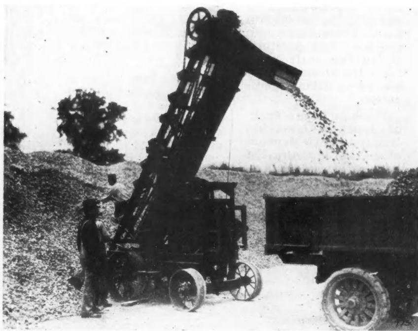
Portable Power Bucket Wagon Loader, Which Puts Materials on the Truck Speedily and Economically. The Endless Belt Carrying the Buckets and the Gas Engine That Provides the Power Are Mounted on a Four-Wheel Truck, Which Can Be Moved to Any Part of the Yard.
