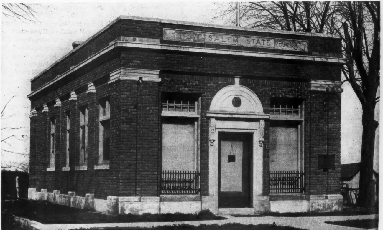
A Good Small Town Bank Design. It Is 55 Feet Long and 20 Feet Wide and of Brick and Terra Cotta Construction. An Impressive Building That Will Reflect Credit on Its Surroundings.
