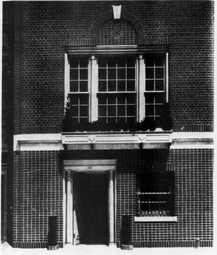
No Small Part of the Beauty of This Brickwork Was Derived from the Mortar. The Mortar Is of the Best Quality and the Joints Carefully Painted.
