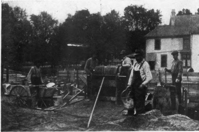
Practical Hand-Propelled Concrete Mixer. This Machine Plows the Mixture Instead of Churning It in Revolving Drum.
