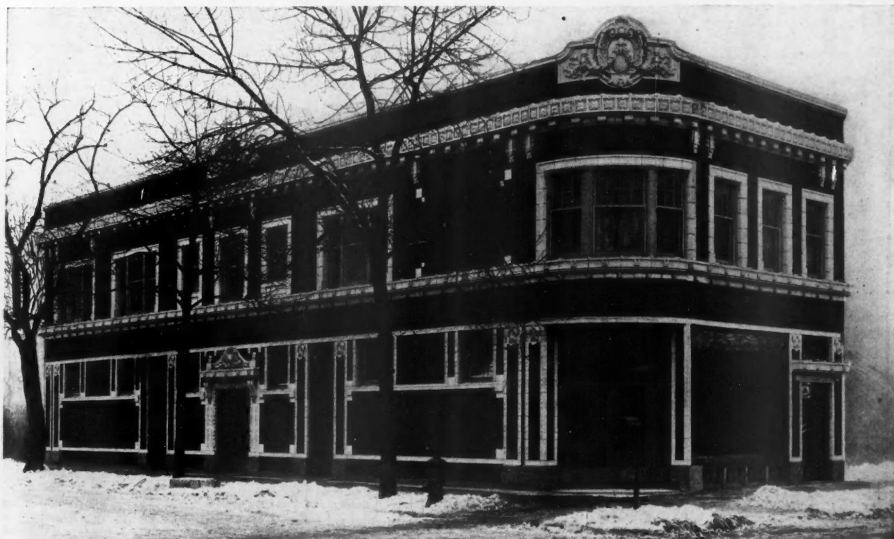
Corner Store and Apartment Building of Brick and Terra Cotta Construction. An Ideal Building for a Corner Lot, Size 96 Feet 6 Inches by 30 Feet. The First Floor Consists of a Store, 28 by 46 Feet, and Stock Room, While the Upper Floor is Divided Into Two Five-Room Apartments.
