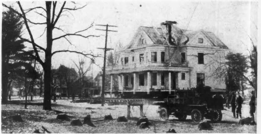
Moving a House by Truck. The Truck Is Anchored to a Stump.
