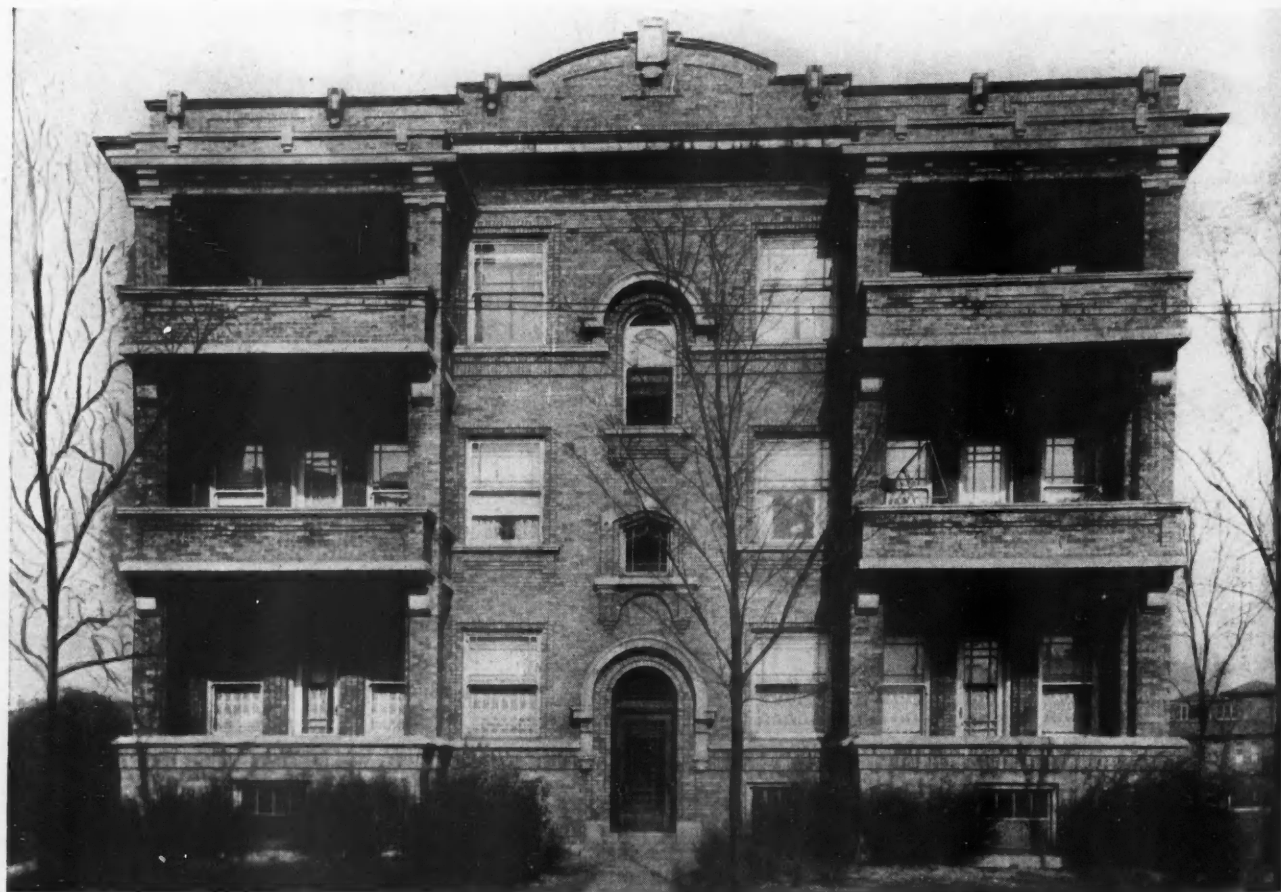
Three-Story Six-Apartment Building of Brick and Stone Construction. This Building, 56 by 60 Feet, Is Built on Substantial Lines and Emphasizes Comfort in Its All-Season Porch and Five Large Rooms. The Living Room Contains a Space-Saving Bed.
