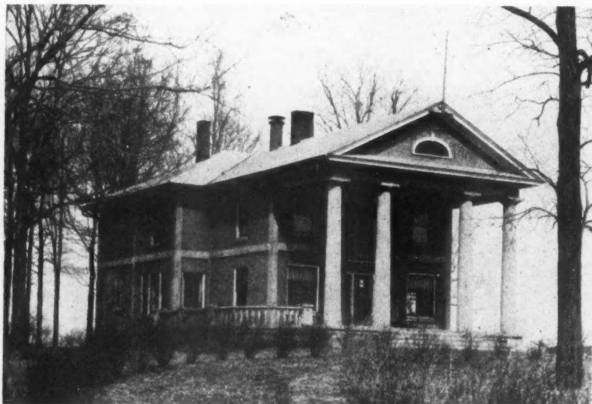
An Unusually Attractive Farm Residence and Office, of Monolithic Concrete, Built of Beam, Column and Curtain Wall Construction, Same System as Is Used in Construction of Modern Fireproof Industrial Buildings.
