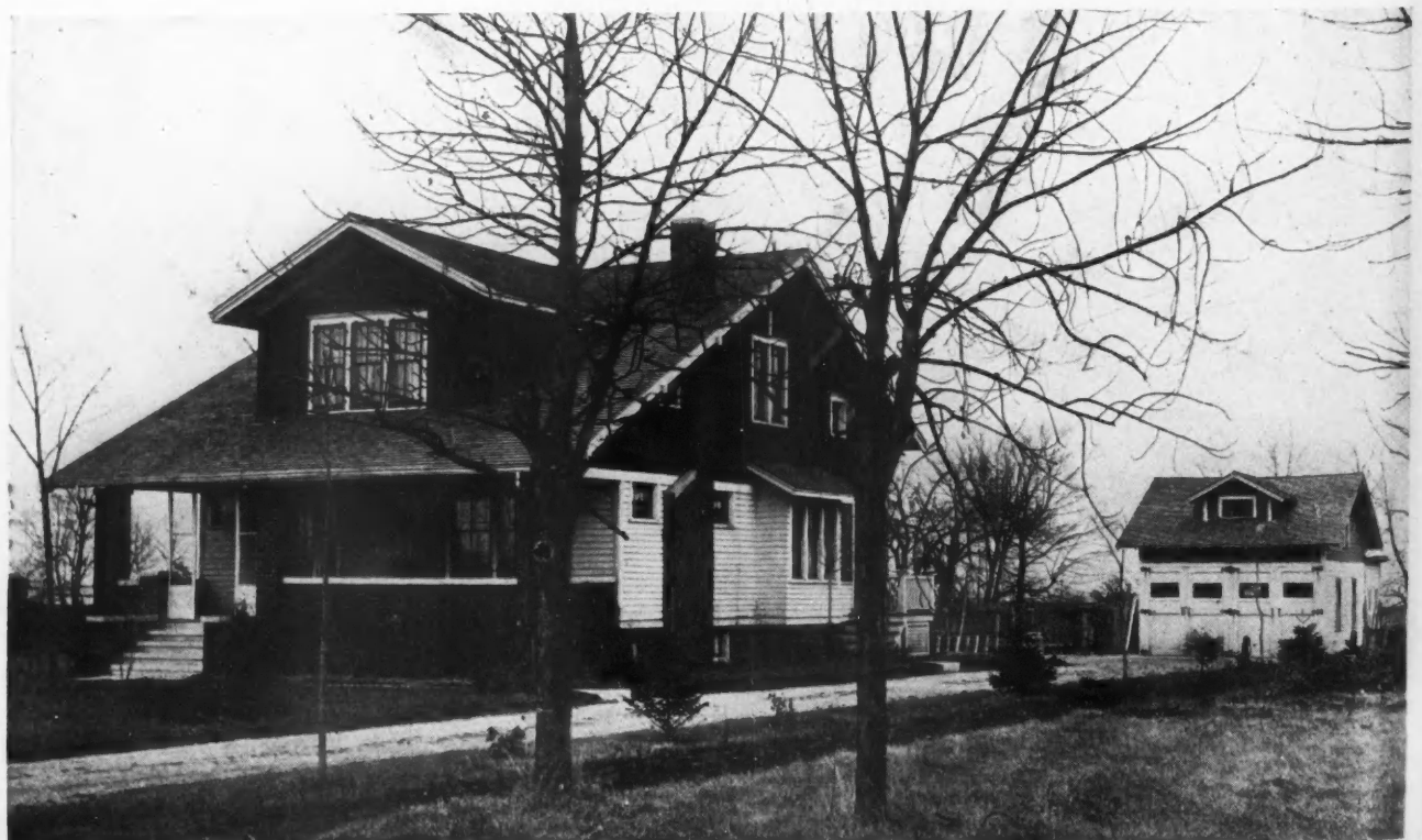
This Pretty Home Contains Eight Rooms and Bath, Altho Its Dimensions Are 40 by 24 Feet. The Large Porch, with Brick Pillars, Is a Good Feature.
