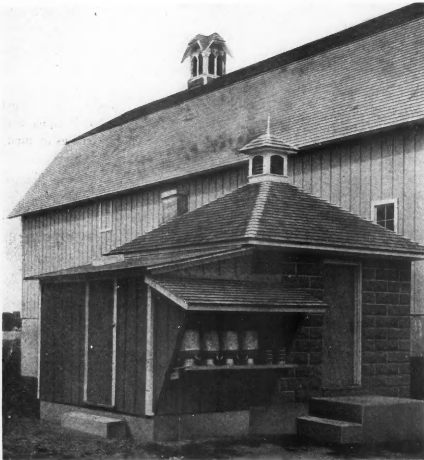
A Concrete-Block Milk House with Frame Addition for Boiler Room and Can Rack. This House Is Built Near the Dairy Barn. The Size, Including Addition, Is 19 by 14 Feet.
