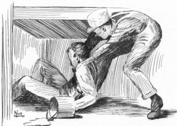
The Elevator Lowered Suddenly, Striking One of the Painters.
