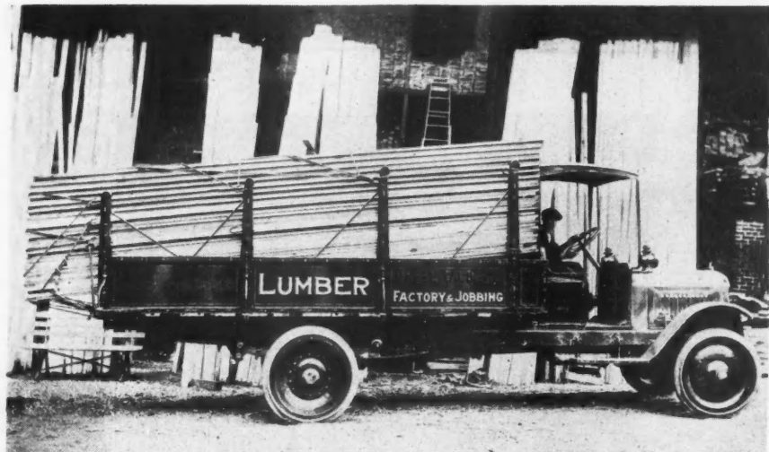
The "Republic" Truck of James E. Tague & Co., Lumber Dealers, Loaded, Ready to Start for the Building Job. This Truck Carries More Than Three Times the Capacity of a Wagon and Has a Speed of 15 Miles an Hour When Loaded. It Is Easy to See Why Motor Trucks Are an Essential Part of the Equipment of Successful Lumber Dealers.
