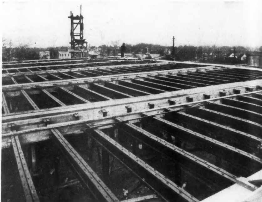
Metal Joists Set Into Concrete, Fireproof Floor Construction Used in Office Buildings, Factories and Other Similar Structures.
