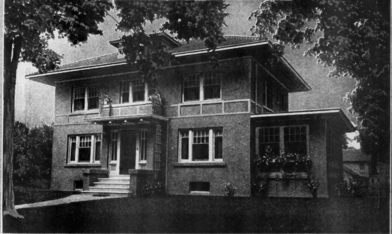
R ECTANGULAR STUCCO HOUSE WITH HIP ROOF. The design of this house is an example of the excellence of the square-type house especially in regard to the convenient arrangement of rooms. The exterior is very neat in appearance and is well "set off" by the wide box cornice and hip roof of tile. In the interior, the living room and adjoining sun porch form the center of attraction. Every requirement of careful design is met in the second floor arrangement. The house is 36 feet 6 inches by 30 feet.
