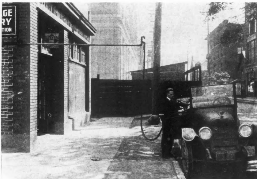
Unique Method of Piping Gasoline to Curb in Front of Garage. The Gasoline Pipe Is Hinged at the Corner of the Building and Swings to the Side of the Building When Not in Use. It Is of a Height That Permits Unobstructed Use of the Sidewalk.
