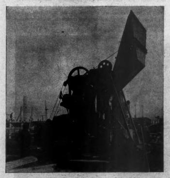
This Paying Mixer Poured the Footings of the Columns in the New Cadillac Plant Frected in Detroit. It Was Used in a Variety of Ways in the Construction Work.
