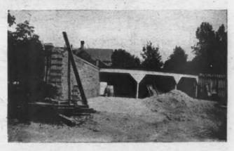
Builders' Supply Yard Equipped with Concrete Platform for Mixing Concrete to Be Worked Up in Spare Time Into Concrete Block.
