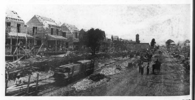
Whole Row in Course of Construction. This Picture Shows How Lumber and Material Were Hauled to Scene of Operations on Nartow Gauge. Speedy Hauling Prevented Many Delays.
