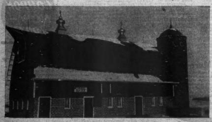
Combination Hollow Tile and Frame Barn with Gothic Root and Hollow Tile Sile Built by W. A. Krengel, Lamberton, Minn.
