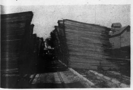
Lumber Yard with Concrete Supports for Piles and Combination Trackway for Jard Trucks and Push Carts. The Rails Are Set on Concrete Slabs Which Are Wide Baugh to Serve as Wagon Wheel Track.
