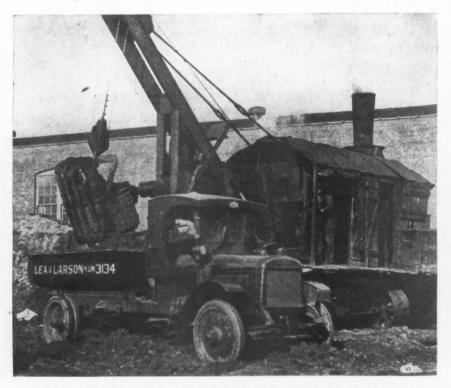
A 3½-Ton "Republic" Truck Doing Its Bit in Excavating Work. Heavy Trucks Have Been Instrumental in Speeding Up Building Work and Cutting Down Costs Because of Their Carrying Capacities and Speed.
