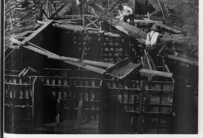
Placing Plants All Set for Foundations. Each Machine Takes Care of Two Buildings. Batch Cars Hauled Mixed Concrete to the Placing Plants from the Unloading Yard.
