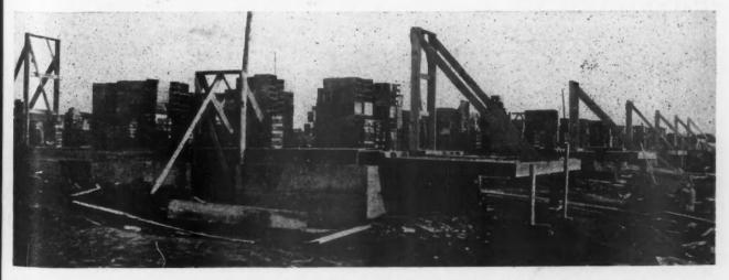
The Carpenters Have Just Finished the Flooring and Have Moved on to Make Room for the Masons to Set the Walls. The Work Schedule Was an Important Factor in Finishing the Job in Remarkably Short Time.
