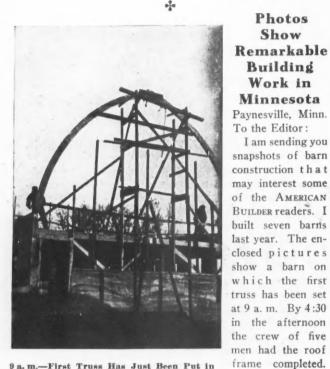
a. m.—First Truss Has Just Been Put in Place by E. A. Opitz, Paynesville, Minn. concrete block barn with the roof starting on the joists. It has a large haymow.
