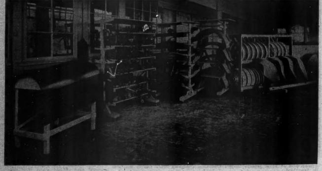
is for Drying Parts After Painting. All Racks Are Equipped with Bollers to Allow Them to Be Taken to Any Part of the Building.
