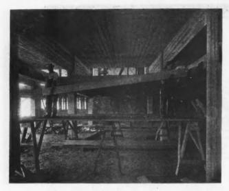
Putting a Beam in Place on Joist Hangers. This Type of Construction Is Used Where Overhead Trackage Is Needed.
