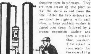
Workman Installing New Spud for Connecting Gas Water Heaters. This Spud Is Fitted Without Disturbing Old Pipes.
