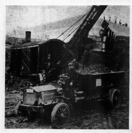
Excavating Is One of the Important Jobs in Building. This Five-Ton "Packard" Is One of the Big Reasons for the Efficiency of the Ariss Constructing Co., Ashland, Calif.
