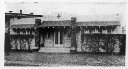
Railroad Foreman's Office and Quarters Built by Standard System of Precast Concrete Units. A Stucco Finish Has Been Applied in the Same Way as in Any Class o Construction.
