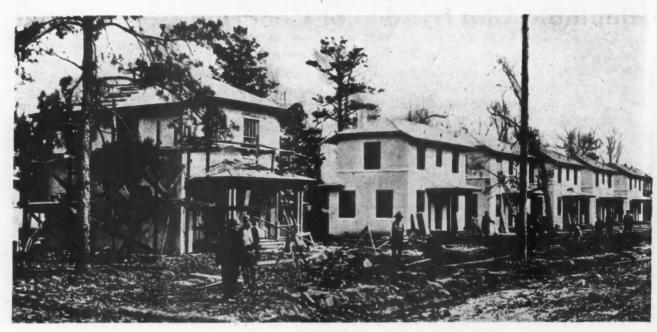
Industrial Housing Group at Baytown, Texas, Built of Precast System. The Units Were Cast on the Site of the Building. By Standardizing the Construction, the Baytown Refinery Co. Effected a Considerable Saving in Costs.
