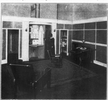
This Revolving Device Contains Four Rooms Which Can Be Brought Into Position When Needed. The Housewife is Just Swinging the Kitchen Into Place. Only One Room and Bath Are Needed with This Space-Saving Appliance.
