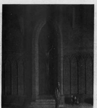
Crucifix Built of Composition Material. It Stands 17½ Feet High. The Head Relief Is 14 Inches. Two Tons of Clay Were Used in Building Molds for It.
