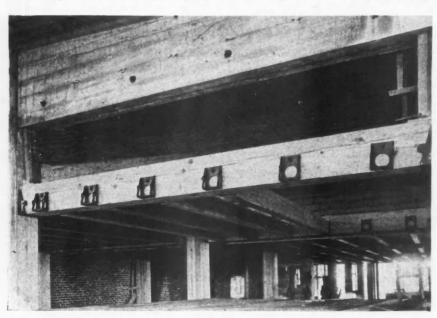
This Picture Shows a New Use for Joist Hangers. They Have Been Fastened to the Concrete Columns and Support the Cross Joist to Which Other Beams Are Attached by Means of Hangers.
