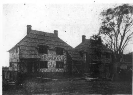
Row of Houses Under Construction in New Toronto, Canada. They Were Built in Series of Ten. Excavations Were Made at the Same Time for Ten Basements. The Walls Are Tile with Brick or Stucco Finish.
