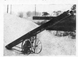
Engine Operating Belt Conveyor at Gravel Pile. This Equipment Is Portable and Can Be Moved from Place to Place Quickly.
