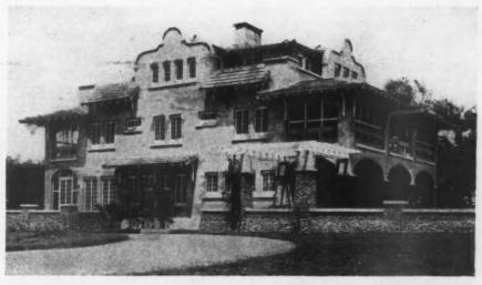
Residence in Houston, Texas, Built from Unit System. The Walls in This Type of Construction Are Precast Concrete Channels Cast in Lengths Equal to the Height of the Floor for Which They Are Used.
