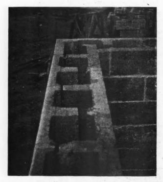
Figure 8. System Illustrating Use of Special Length Corner Block.
