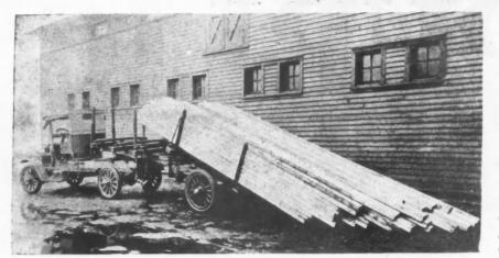
Jack-Knife "Trailmobile" Just as the Load of Lumber Has Been Rolled Past the Center of Gravity and Is Tipped Off.
