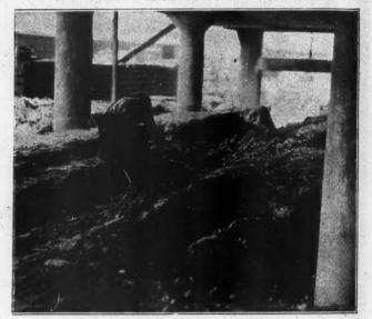
Man Guiding the Digging Slip Under the Building. The Entire Basement Was Excavated After the Building Had Been Constructed.
