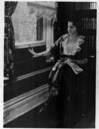
The Fresh Air Enters the Room But Is Deflected Upward so There Is no Trace of Draft When a Person Sits Next to the Window. The Arrangement Also Prevents Rain from Coming Thru.
