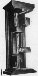
Cross Section of Double Window Showing Weather-strip in Position. Note Part-ing Rail or Bead, Z-Bar and Meeting Rail
