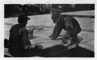
Laying Concrete Slabs on Roof. This Material Is Porous Concrete and Is Designed for Use as Sheathing and Siding. It Acts as Insulation Because of the Small Air Holes Which It Encloses.
