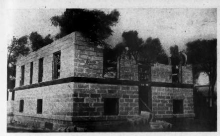
Figure 4. Dwelling of Concrete Stucco or Foundation Block to the Surface of Which Portland Cement Stucco will Be Applied.
