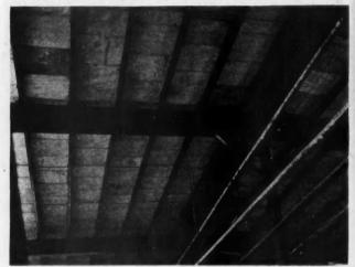
Underside of Roof Over Which Concrete Slabs Have Been Laid as Sheathing. This Material Can Carry Fairly Heavy Loads. Nails Can Be Driven Thru This Material to Wood Studs.
