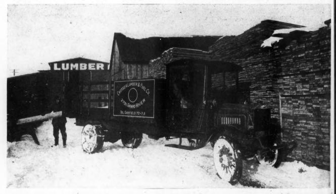
Winter Brings With It Rough and Slippery Roads. Crotser Lumber and Fuel Co., Detroit, Mich., Have Found a Solution for Hauling Lumber Under These Conditions. They Use This 5-Ton "Service" and Several Others All Thru the Severe Weather. Chains Eliminate Sliding While Power Conquers All Rough Roads.
