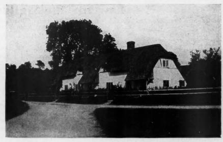
Typical Stucco Cottage Found in Many Sections of England. This Material Is Gradually Replacing Stone Because of the Difficulty Connected with Quarrying and the Scarcity of Labor. This Thatch Roof Is Made of Wheat Straw or Reeds.
