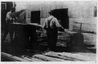
One Machine of the Type Shown Here Will Perform Many Operations, Such as Jointing, Grinding, Mitreing, Rabbeting and and Dadoing. Many Lumber Dealers Are Installing Saw Rigs in Their Yards.
