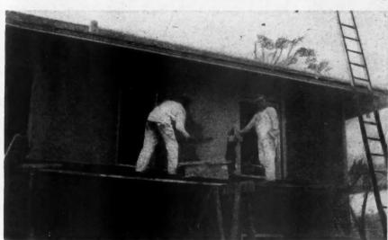
Figure 5. Applying Portland Cement Stucco to Concrete Block Surface.
