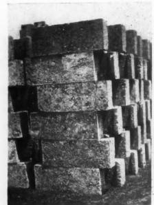
Figure 1. Pile of Stucco or Foundation Block, Showing the Uniformly Rough Texture Produced by Using a Standard Concrete Mixture Thruout the Block Without Fucing.
