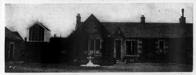
Stone Workman's Cottage at Ayrshire, Scotland. Durability Is One of the First Considerations of the Builder. Climate Determines the Thickness of the Walls. Note the Shingle Roof Which Is Rapidly Displacing the Thatch Formerly So Popular
