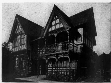
Half Timber Type of House at Largs, Scotland. In This Construction Heavy Timbers Are Framed Together and the Panels Filled with Brick, Then Coated with Stucce. Note the Sharp Gables
