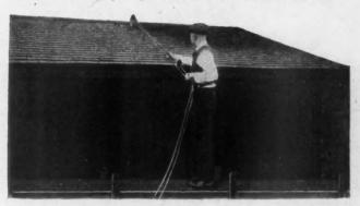
Applying Paint on a Roof. By Adding Sections Scaffolds and Ladders Can be Eliminated in the Painting Job. This Machine Will Apply Waterproofing Material.
