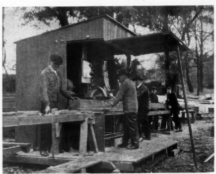
Efficient Methods Now Call for the Cutting of Rough Lumber on the Scene of the Building Activity. Here a Handy Woodworker is Doing the Work of Many Men. Another Cog in the Great Labor-Saving Process.
