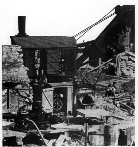
Machinery on the Job. We Need no Stronger Testimony Than Is Presented Here as to the Merits of Modern Machinery and Equipment on the Building Job. There Are the Mixer, the Gas Engine, the Pump, and Steam Derrick, All Cutting Labor Cost and Speeding Up the Work.
