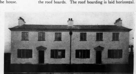
Steel Framed House Finished and Ready for Occupancy. This Is the So-called Semi-Detached House, Containing Four Apartments. The Floors Are Concrete with Oak Covering.
