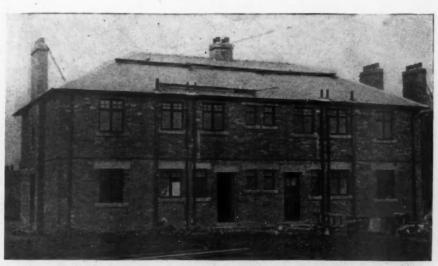
Back View of Foursome Brick House. The Two Tenants on Ground Floor Use Front and Back Doors, While the Tenants for the Upper Floor Enter by the Door in the Ends of the House.
