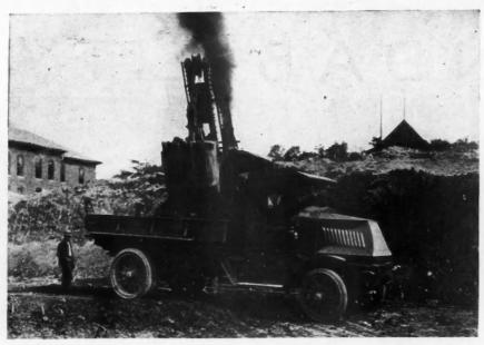
Dempster Construction Company Found This 3½-Ton "Mack" Truck Could Keep Up with a Steam Shovel Despite the Heavy Grade. It Also Used a Short Cut Which Was Impassable for Horses.
