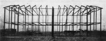
Steel Framed House, Showing Steel Framing for Walls and Roof. The Upright Frames Are T-Irons, the Roof Angle Irons. The End Gables Are Trimmed for Brick Chimneys.
