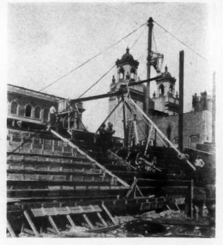
Another Unique Type of Hoisting Bucket Operated on a Single Mast. Here They Are Pouring Concrete for a New Baseball Grandstand.
