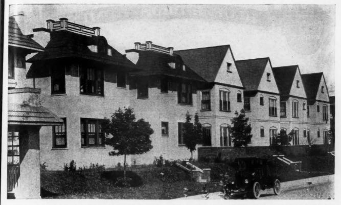
Fig 3. Street of Attractive Homes Showing Various Types of Composition Roofs. The Second House To the Left Has Been Covered with Shingles Thatched Style, Also the Third House, While on the Next Two, the Gabled Roofs Have Been Covered with Asphalt Shingles of Even Color. It Makes a Very Pleasing Variety of Roofs.
