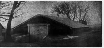
Concrete Vegetable Storage Cellar, a Handy Building on the Farm for Storing Produce. This Building Is 30 Feet Wide, 48 Feet Long and 7 Feet High. It Is Built of Concrete and Insulated in an Unusual Way.
