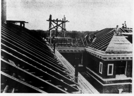
Steel Lumber Used as Structural Support in Permanent Roof Construction. This Is a Hip Roof With Steel Joists Used as Roof Rafters.
