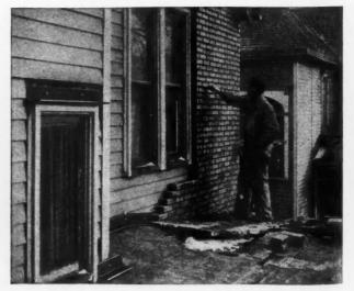
Veneering Above Kitchen Roof. Steel Angles Angles Angles Angles the Sheathing and Attached To the Study So Weight of the Brickwork Comes on the Roof. Are
