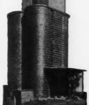
For twenty years NATCO Glazed Bin Tile has given the utmost satisfaction in the construction of practically every type of bin used for the storage of grain, coal or other ma-terial. Such bins have proven absolutely fire - safe. They never need painting or repairs. One unit is used throughout. The steel air spaces in each unit effectively prevent and keep cold and moisture from penetrating through the walls. Deep and wide channels
