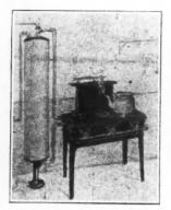
Boiler Connected with New Stove Top Water Heater. This Device Heats the Water in the Boiler While the Meals Are Being Cooked and Without Much Extra Fuel Consumption.
