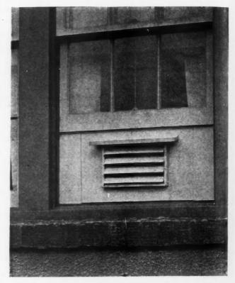
View of the Window Cooling Device from Outside Showing Shutter Arrangement and Adjustable Panel in Which It Is Set. This Presents a Neat Outside Appearance in Keeping With the Finest Home or Apartment — No Projecting Box as With the Ordinary Window Cooler.
