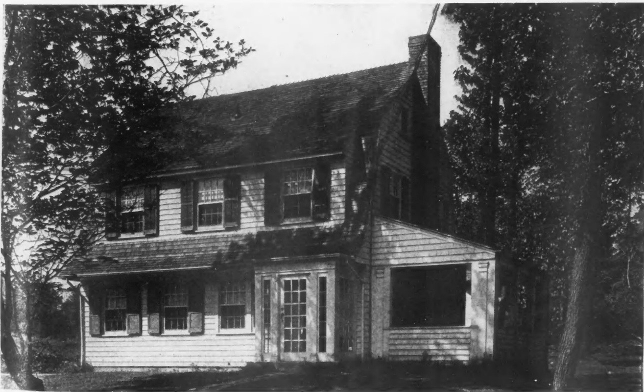
Well Designed Dutch Colonial Residence of Six Rooms. The Side Walls are 4-Inch Studs Sheathed and Shingled. Simplicity of Design Has Made This House Economical to Build. Owner, F. Halderman, Tenafly, N. J.; Architects, R. C. Hunter & Co., New York City.
