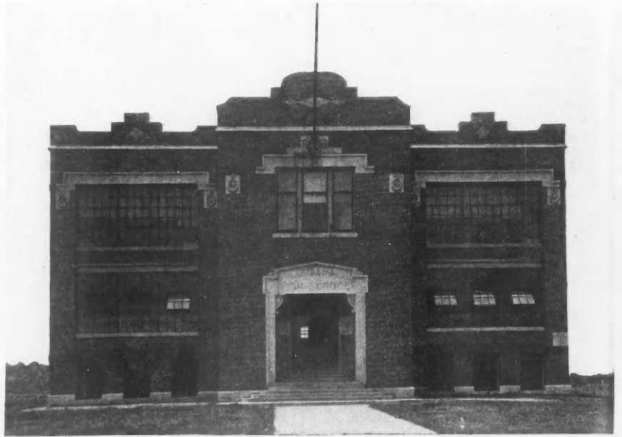
Steel Sash with Pivoted Ventilators Make This Urbana, Ind., School Quite Attractive and as Modern as Schools in Larger Cities.
