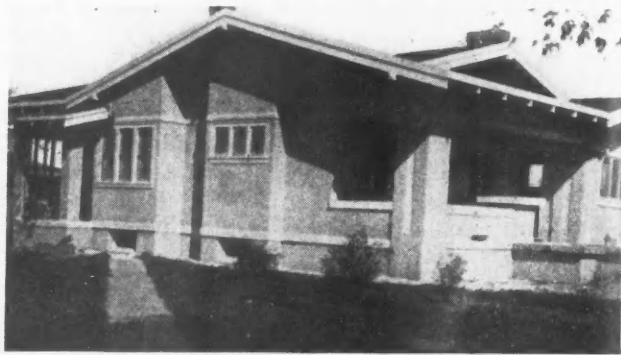
This Modern Home Has Running Water, Electric Light and Many Other Features Which Are Advocated by the American Builder. Erick Olson Was the Contractor.
