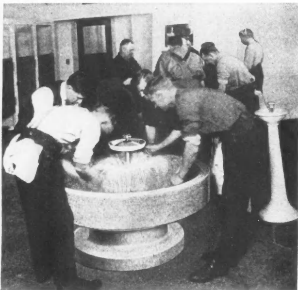
New Wash Fountain Designed To Improve Sanitary Conditions in Factories, Schools, Public Buildings, etc. It Also Saves Considerable Space.
