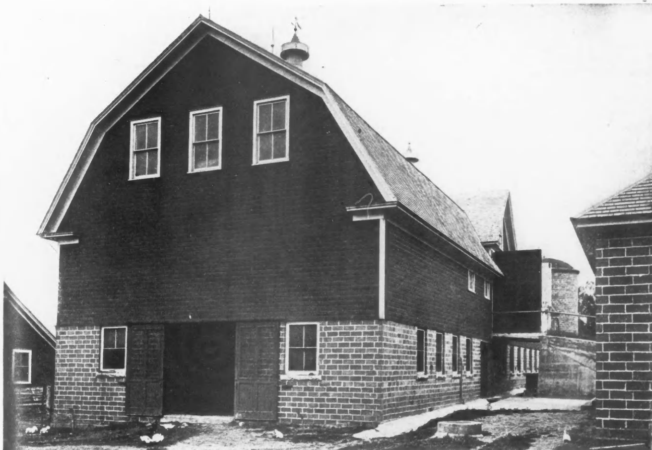
View of Modern Dairy Barn, 36 by 110 Feet, with Concrete Approach to Upper Hay Mow. This Barn Has Stalls for Forty-Four Cows, Calf and Bull Pens, Record Office, and Large Feeding Room with Two 10-Foot Diameter Brick Silos.
