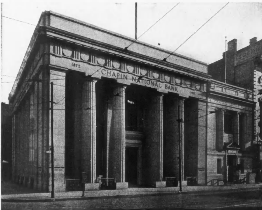
Details of This Massive Bank Design Are Well Executed in Concrete Stone. Note Span of Central Lintel. Stone by Emerson & Norris, Boston; Mowbray & Ufinger, Architects, New York; Fred T. Ley & Co., Boston, Contractors.
