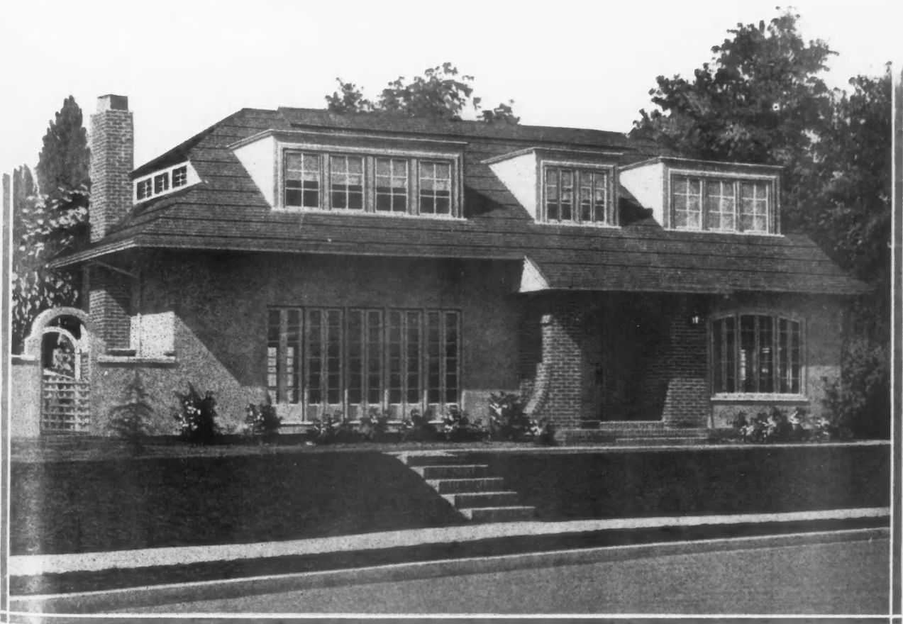
"SUNSHINE" HOME. Easily the outstanding feature of this beautiful compactly constructed house is the abundance of window space. Upstairs and down, each room has many windows, admitting plenty of health-giving sunlight. It is built of tile coated with stucco and a few added touches around the entrance in special texture brick. The roof presents a very pleasing appearance, made up as it is in the thatched effect with composition shingles. The large living room at one end is a veritable storehouse of cheer and brightness as a formidable row of French doors in front and walls make it a room of glass. A large fireplace is located in the side wall. There are three rooms on the lower floor and three above. While giving an impression of bigness this house is not extra large in size, being 46 feet wide and 35 feet deep.
