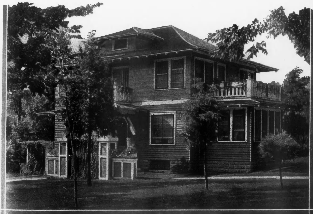
CONSERVATIVE, WELL-DESIGNED FAMILY HOME. For the larger family this type of house is appropriate. This is a two-story frame house of eight rooms, five of which are bedrooms, which insures facilities for a large family. The foundation is rock-faced concrete block and frame siding is used up the second floor with shingles above to the cornice. The roof is modified hip with one attic dormer. Variation from the usual style of the square house is found in the projecting sun parlor with balcony above. The main entrance is on the side opening into the large living room. A bedroom with toilet off the living room is convenient for guest room. There is also a breakfast nook adjoining the kitchen. The main bedrooms, four in number, are on the upper floor. Little space has been sacrificed for large, unwieldy closets. Size of house, 28 by 36 feet.
