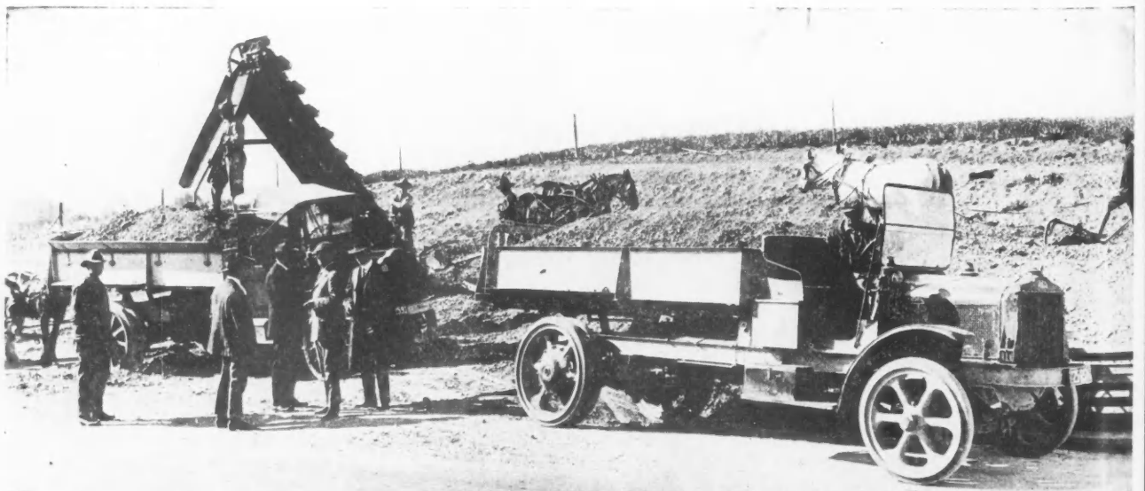
Two 5-Ton "Whites" on the Job. They Helped Build Eight Miles of Fine Road in San Luis Obispo County, California, in Five Months They Averaged Six Trips Daily Carrying 5½ to 6 Yards of Gravel.
