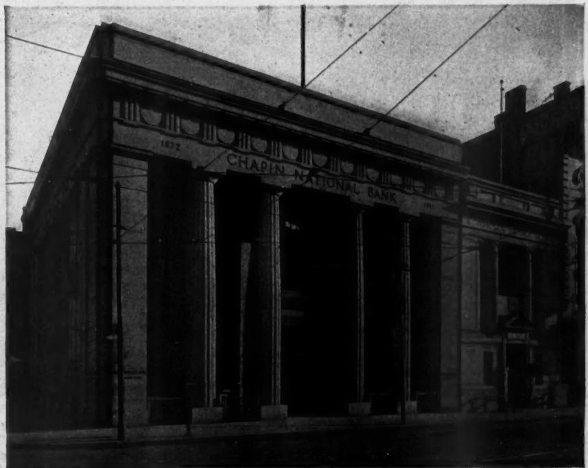
Details of This Massive Bank Design Are Well Executed in Concrete Stone. Note Span of Central Lintel. Stone by Emerson & Norris, Boston; Mawbray & Uffinger, Architects, New York; Fred T. Ley & Co., Boston, Contractors.
