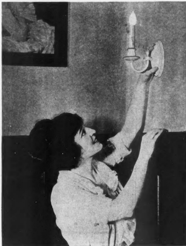
Handy Type of Wall Bracket Which Can Be Put in Place Quickly Provided Small Outlets Have Been Placed in Wall by Contractor. A Small Room Should Have at Least Three of These Convenience Outlets.
