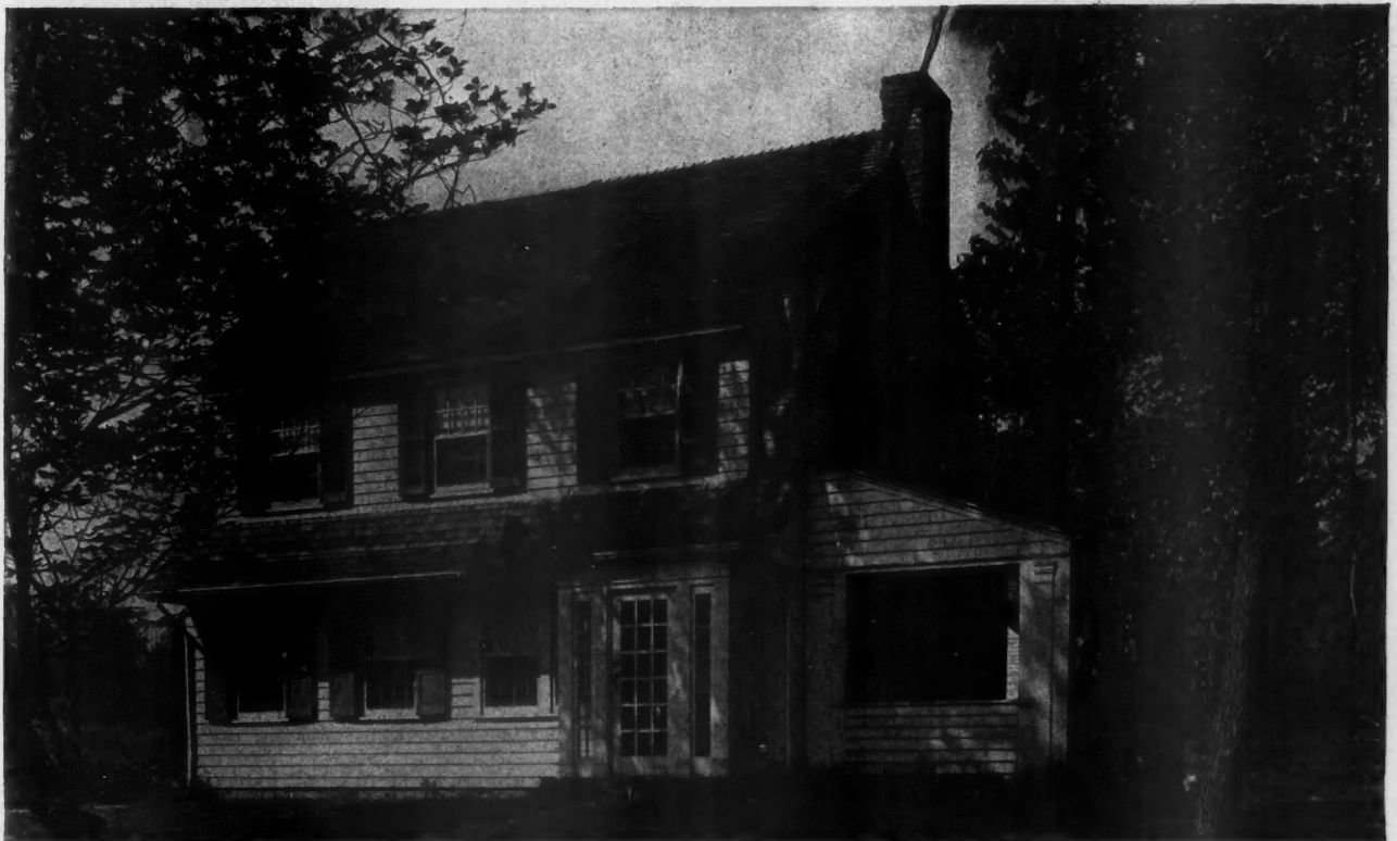
Well Designed Dutch Colonial Residence of Six Rooms. The Side Walls are 4-Inch Studs Sheathed and Shingled. Simplicity of Design Has Made This House Economical to Build. Owner, F. Halderman, Tenafly, N. J.; Architects, R. C. Hunter & Co., New York City.
