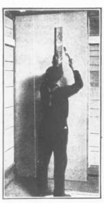
Panel Is Nailed at Top. A Piece of 2 by 4 Is Laid Over Studs and Struck with Heavy Hammer Blows. Fasteners Clinch Into Back of Board.
