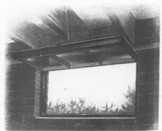
Window As It Appears Open with Chain Holding in Position-Note Level Instead of Sloping Sill
