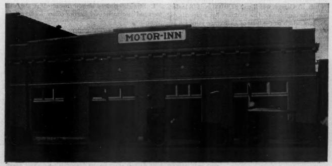
Motor Inn Garage, Detroit, Minn., Built of Concrete Brick. This Type of Fireproof Structure Is Designed to Cut Fire Bisk and Insurance Rates, and Remove Menace of Public Parking.
