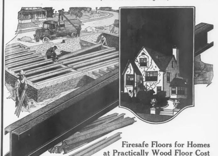
HINK of it! The same type of floor that has long been used in skyscrapers, at little more than the cost of combustible wood floors, is now made possible by the use of National Steel Joists.
