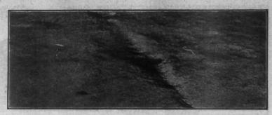
The Rut in This Floor Is at a Joint or "Seam" in the Concrete. Very Often When These Joints Are Not Well Bonded, a Line of Weakness or Soft Spot May Develop. Such a Line of Weakness, if Traversed Daily by Heavily-Laden, Metal-Wheeled Trucks, Will Wear Into Holes. When Trucks Begin to Bump Into Such Holes, Not Only Do the Rutted Sections Wear Faster, but the Entire Surrounding Surface as Well.
