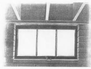
Another Type Basement Steel Sash, Showing Permanent Lock Attacked.
