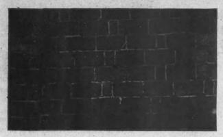
bond, three stretchers being followed by a header, the header on the next course centering over the space between the headers below. This particular wall was standing upon sloping ground and the courses followed this natural slope instead of being laid horizontal and the wall stepped off at the top, the usual practice here. The wall is about seven feet high and eight inches thick, with buttresses about every twelve feet. The buttresses, by the way, were perpendicular.
