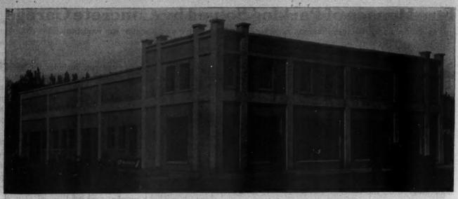
Public Garage at Eliendale, N. D., W. E. Hart, Owner, Built of Reinforced Concrete J. W. Finkle & Son, Contractors. It Has a Stucco Coating and Is Designed to Be Fireproof. It Has a Shew Room With Offices Above.
