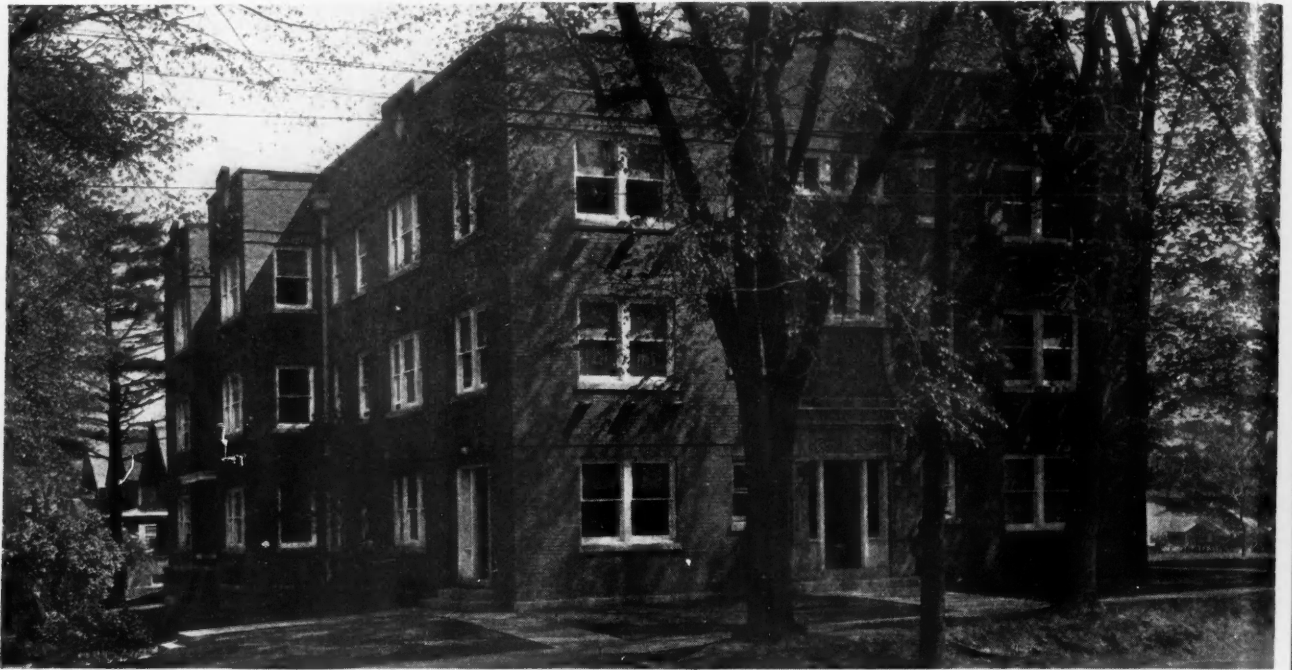
The Highland Apartments, Front and Side View, Showing Difference in Treatment from Court Type in Chicago. This Is Known as the Corridor Type, the Corridor Being on the Inside of the Building with Apartments Along Each Side. This Building Has 11 3-Room and 12 2-Room Apartments.
