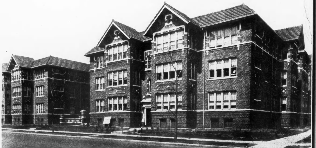
Typical Court Apartment Building. Example of the Architectural Motif Which Chicago Favors Today. The Court Provides Extra Lighting Advantages to All Apartments and Breaks Up the Cold, Unappealing Straight Front Elevation.
