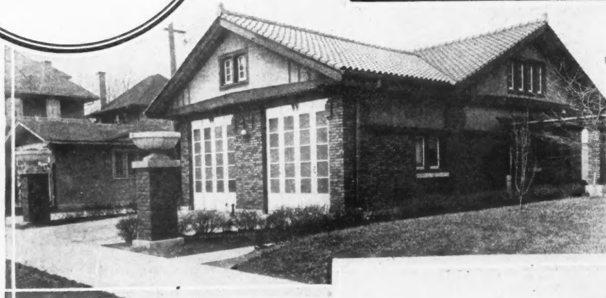
Two-Car Garage with Apartment for Chauffeur. It is Built of Brick and Stucco with Tile Roof and Has Folding Sliding Doors.
