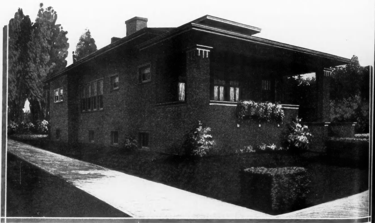
POPULAR CITY-STYLE BUNGALOW. Bungalows of four, five and six rooms are popular in the cities for the reason that they do not require large, and consequently expensive lots. The stucco bungalow design shown above is of this type. It is 20 by 50 feet, with an 8-foot front porch projection, and with the exception of the bay in the kitchen walls are unbroken lines. Five good rooms are shown on the floor plan. The living room is a feature because of its size and the fact that it has outside exposure on three sides. The two bedrooms are so located that they are separate from the other rooms, while the bathroom is between them. A basement extends under the whole house. This is a very desirable design for those who want a small house at a reasonable cost.
