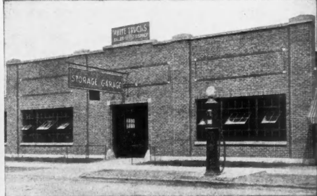
In Public Garages Standard units of Truscon Steel Sash in solid brick walls makes a fireproof building for the Lorenz Garage, Lansing, Mich.
