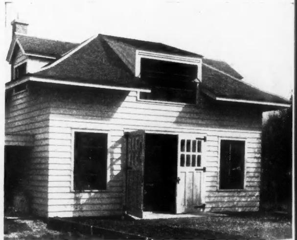
Private Garage Equipped with Steel Sash. This Type of Small Building Is Well Adapted for the Use of This Material.
