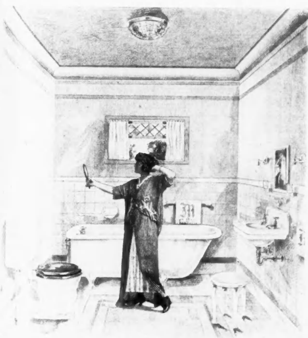
The Luxury of the Modern Bathroom Found in the Most Humble American Homes Is Largely Due to the Constantly Available Supply of Hot Water. This Is Possible Because of the Remarkable Development in Hot Water Heater Manufacture.
