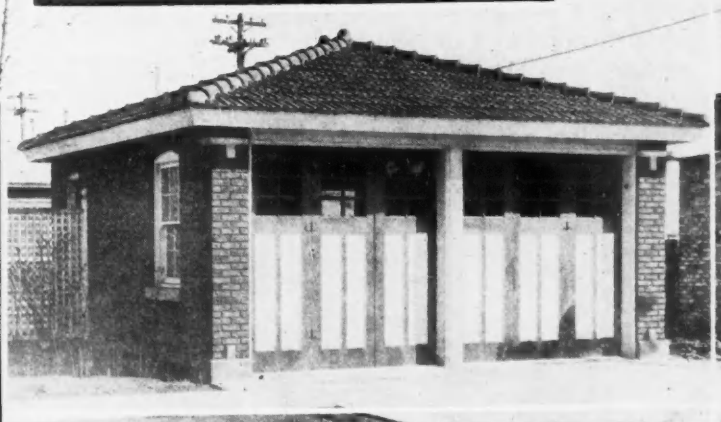
Garage Design That Is Practical and Attractive. Each Section Has a Three-Door Arrangement, the Inside Door Swinging on Hinges, the Other Two Folding and Sliding Back Against the Outside Wall.
