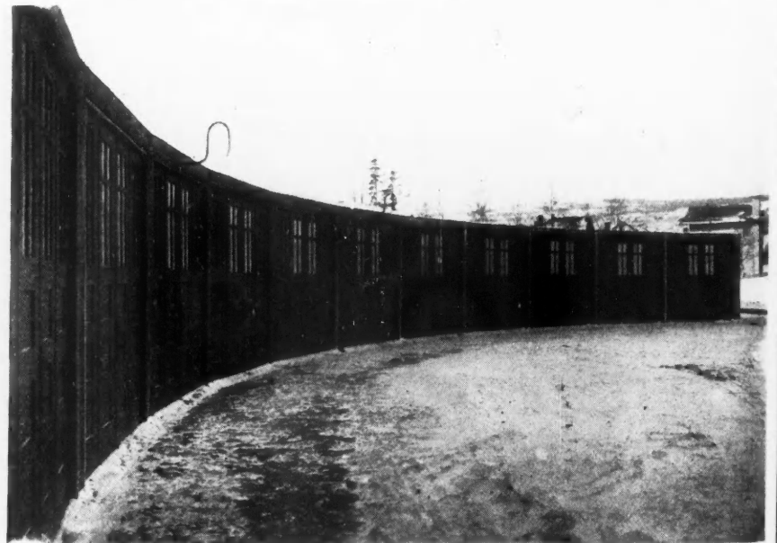
Figure 2. Circular Community Garage at Morgan Park, Duluth, Minn. It Is Built on the Principle of a Roundhouse and Is Now Entirely Concealed by Means of Terraces and Beautiful Landscaping. Concrete Block Were Used in the Walls.
