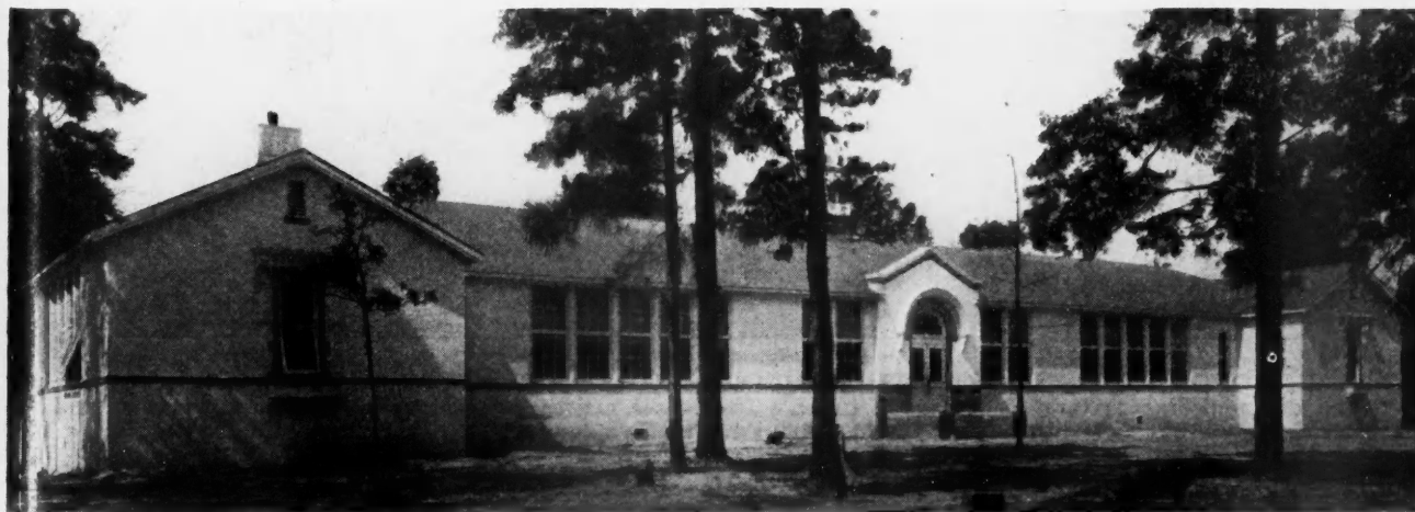
Junior High School at Mount Olive, Ala., Showing New Type of Individual Unit Building That Is Being Used in This Section. Plenty of Daylight Is One of the Outstanding Features and Additions Can Be Put on Quickly Without Much Expense.
