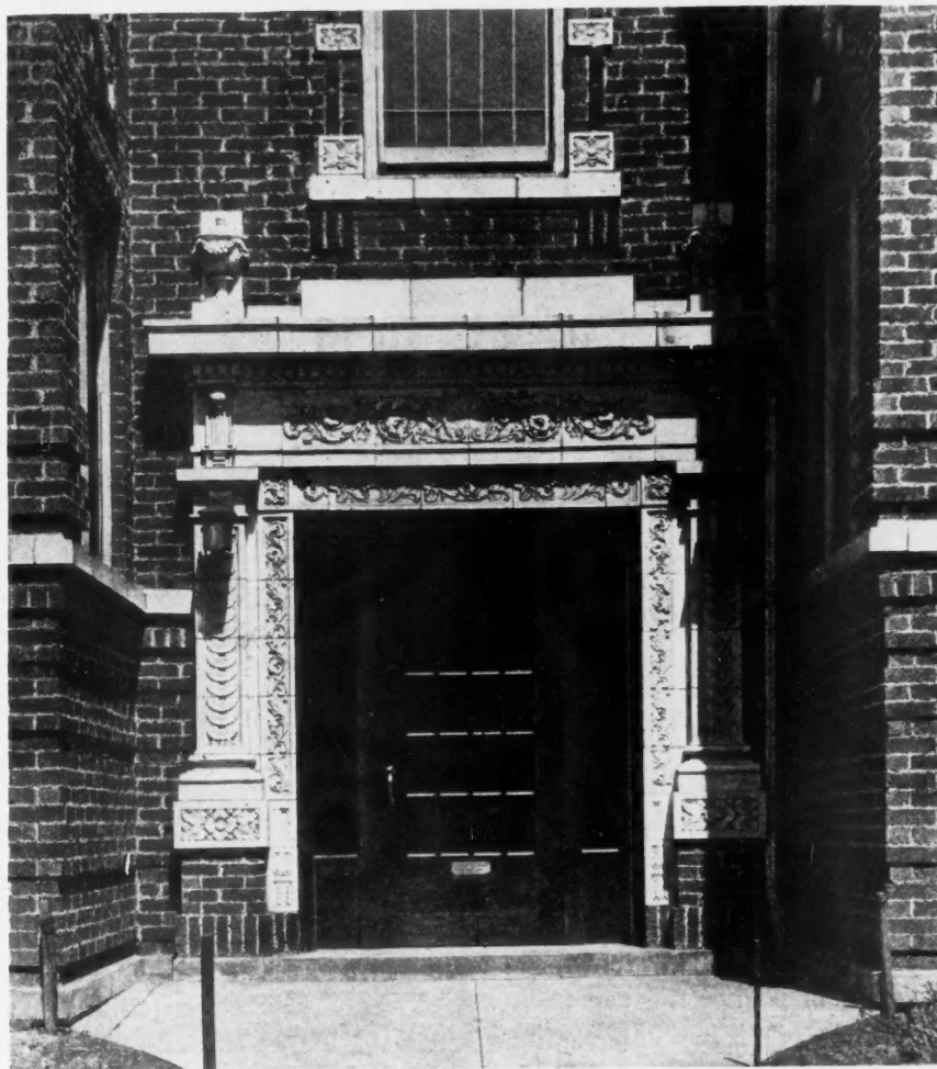
Detail of Entrance of Chicago Apartment Showing Terra Cotta Treatment on Main Entrance and Windows. The Single Door Is Simple but Dignified in Design and Opens Into Hallway Giving Access to Six Apartments.
