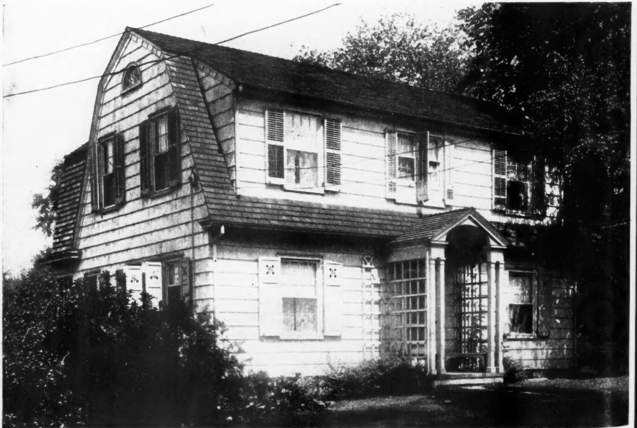
Simplicity of Treatment Makes This House Exceptionally Inviting and Charming. The Rooms are Comfortable and Efficiently Arranged. In the Rear of the House Adjoining the Living Room is a Large Living Porch. The House is 35 by 26 Feet.
