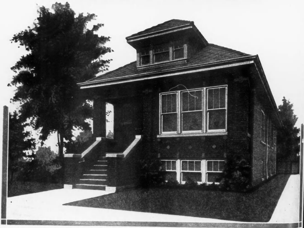
COMPACT, SUBSTANTIALLY BUILT BUNGALOW. This type of brick dwelling is quite popular in the large cities because of its practical arrangement, sturdy construction and economy in cost. It is solid brick on a concrete foundation, with concrete porch and steps and stone trim. The roof is covered with asbestos shingles. In keeping with the modern demand, this house has a sun parlor with triple windows on three sides. Abundant sunlight from this room as well as from two triple windows on each end of the living room, make that room exceptionally bright. For a small home the living room is a delightful surprise, 11 by 22 feet. No space has been given over to a vestibule. In addition to the living room and sun parlor, there is a good-sized dining room, 14 by 10 feet 9 inches, two bedrooms and kitchen. Bedrooms and bath have been grouped along one side of the house off a hall which also opens into the kitchen. The house is 24 by 50 feet.
