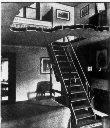
How Attic Can Be Used Without Using Up Space Below for Stairway. This Stairway Can Be Pushed Up Out of the Way When Not in Use.
