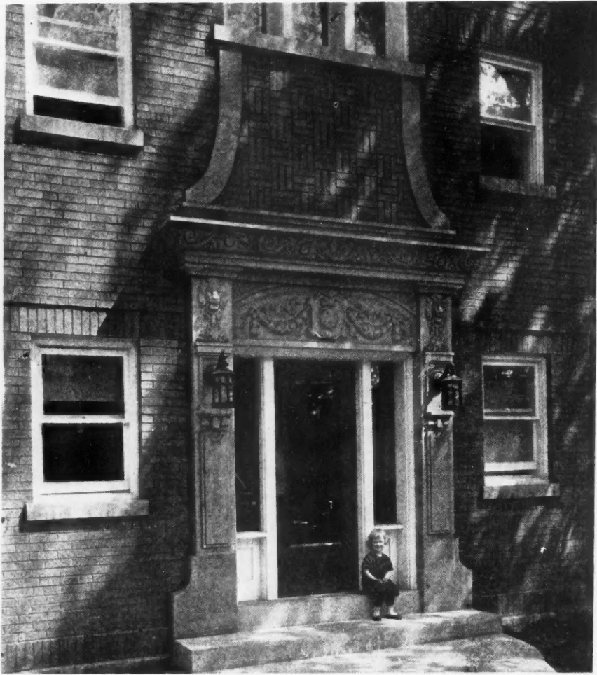
Front Entrance Detail of Rockford Apartments. Artistic Treatment Has Been Made of This Important Part of the Building. Bedford Stone Being Used with Special Paneled Brick Courses.
