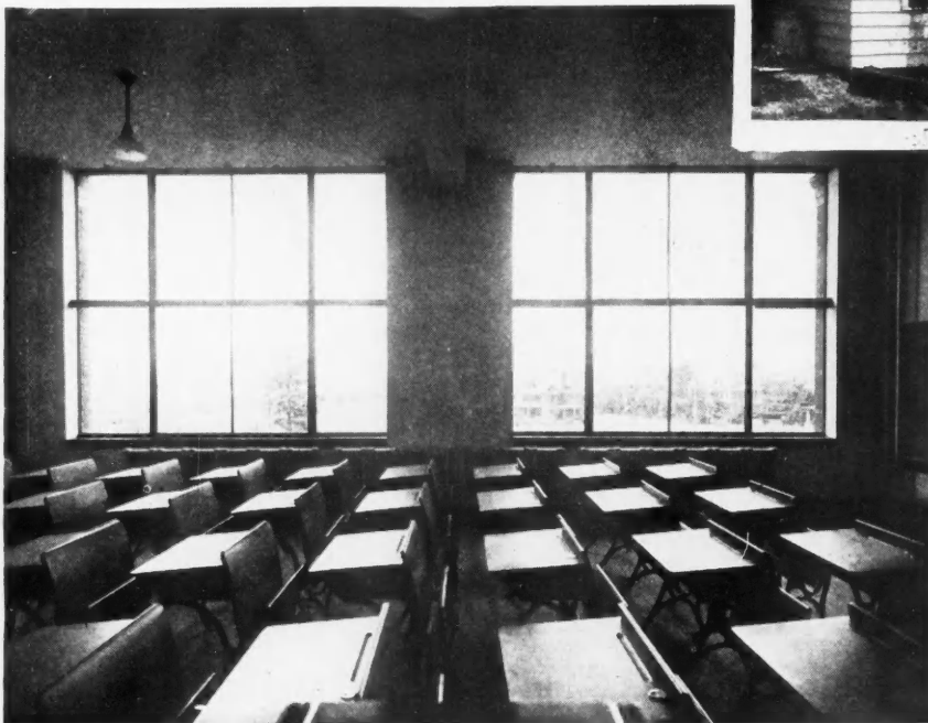
View of Room in Allentown, Pa., High School, Showing Variation in Steel Sash Design. In This Building the Double Hung Sash Type Is in Use.
