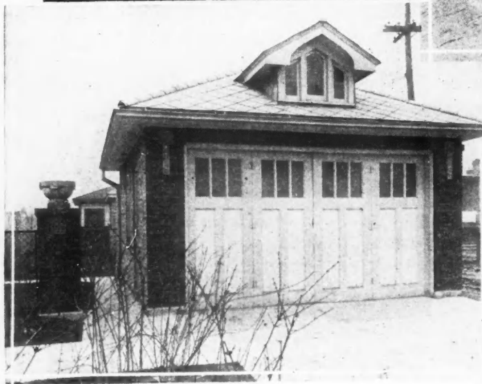
Asbestos Shingles and Roof Dormer Add Variety to This Garage Design. It Has a Hipped Roof and Four Folding Doors.
