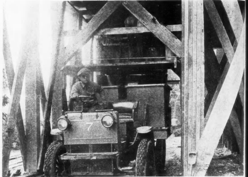
Fig. 1. Truck with Special Dual Dump Body in Position Under Gravel Hopper. This Truck Can Be Loaded Quickly and Accurately, as Each of the Compartments Holds a Specific Amount.
