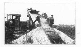
Fig. 2. Excavator and Loader on Gravel Pit Work.
