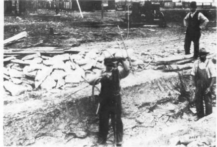
Power Operated Air Compressor Rig Successfully Drilling in Hard Rock at St. Paul, Minn.
