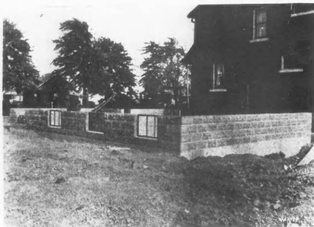
Steel Sash Windows Are Installed as the Wall Is Laid.
