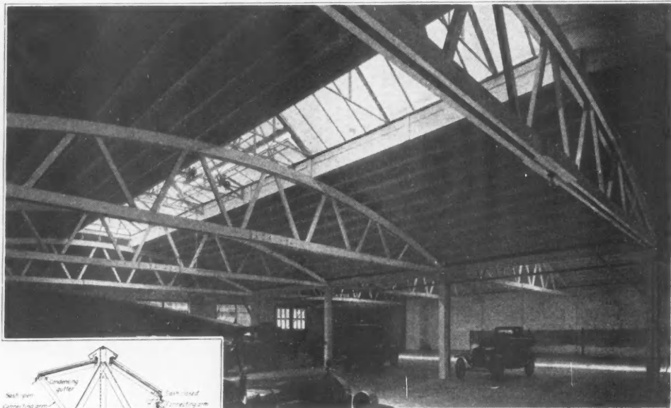
Interior of Garage, size 100 x 200, having 2 spans of 50'-0" McKeown Bowstring Trusses and 2 Blaski Ventilating Skylights, size 8' x 60'.
