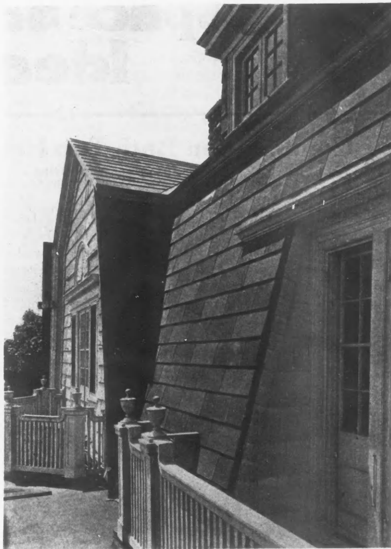
This Picture Shows Copper Shingles on the Home of Otto Myers, New Rochelle, N. Y.
