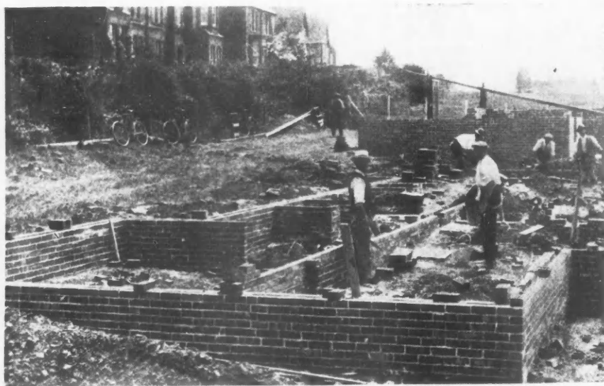
The Foundation for a Brick Home in England. Most of Them Are Built Without Basements.
