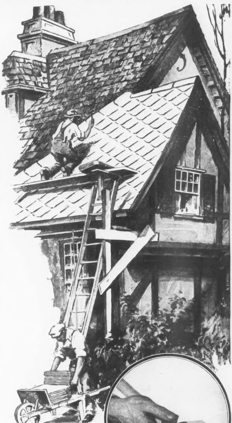
A lather's hatchet is the only tool required to lay Johns-Manville Asbestos Shingles.
