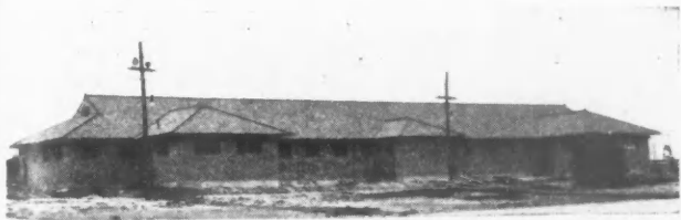
One of the Two Public Bath Houses Built to Endure.
