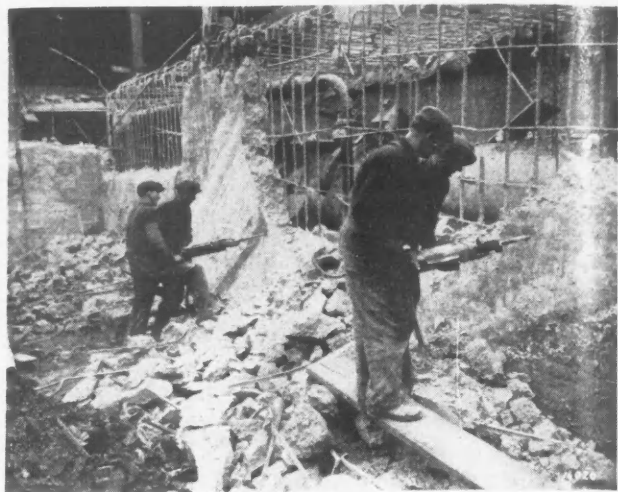
Paving Breakers Successfully Used to Demolish Heavy Vault Walls.
