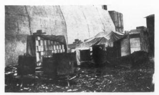
Tarpaulins and Salamanders Used in Heating Concrete Block to Be Laid During Cold Weather. Warm block lay easily and rapidly and protect the mortar against freezing.
