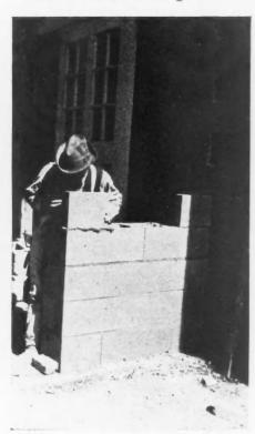
Laying Concrete Block at Temperature Around Freezing. Notice that the mason is not wearing his gloves.
