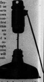
evice for Lowering and Dis-connecting Light Fixtures.
