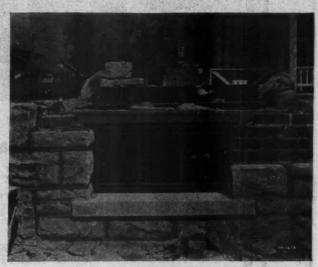
Closeup of Steel Cellar Sash in Stone and Brick Wall.
