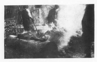
Iron Pipe Sections Being Used as Heaters for Sand and Gravel on the Work of the New Chicago Union Station. allow the contractor's gangs to be disorganized and incomes to cease.
