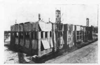
The Upper Tarpaulins on This Building Protect Newly Deposited Concrete. Those below trap heat used in hardening the second floor. Later these same tarpaulins will be used to protect the plastering.
