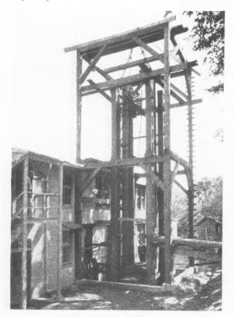
The Giant of All the Testing Machinery is Capable of Exerting a Force of 1,000,000 Pounds and is Used in Testing to Destruction Wooden Columns that are 30 Feet Long and a Foot Square.
