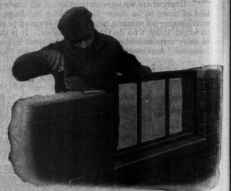
Mason Insets Anchor Clip in Channel Groove.
