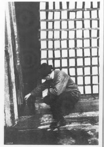
The National Timber Experts Have Invented a Valuable Water-Spray Kiln in which Humidity Can Be Controlled Artificially. The drying rate of the lumber is regulated by conditioning the air with sprays of water whose temperature is carefully regulated.
