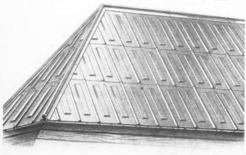
Portion of Roof Covered With Aluminum Laid Downward From the Ridge
