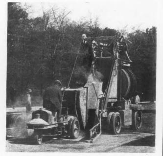
Milwaukee Firm Uses Rubber Tired Pavers Because They Transmit Few Shocks and Are Easier on the Pavement.
