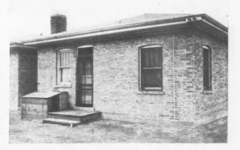
Rear Wall of a Garlow Showing 18 Ft., Built-in Steel Beam Construction. The brick beneath the beam is built into a panel which can be removed without disturbing the rest of the wall. This leaves a space for swinging the garage doors.
