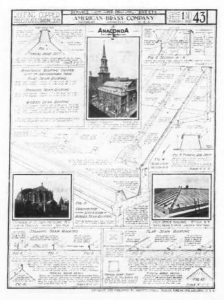
valuable and interesting to anyone interested in copper roofing. Service sheet No. 1 has excellent diagrams, photographs and scale drawings of flat seam roofing, standing seam roofing and ribbed seam roofing. There is also a great deal of other useful information about copper roofing. There is a table showing the recommended sizes and weights of copper for roofing and a list of standard specifications.
