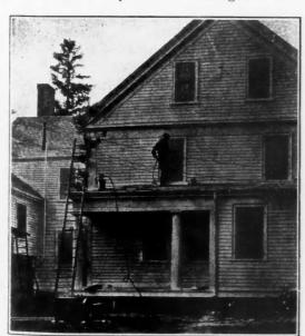
House Painting with Hand Brush Equipment and Enginedriven Air Compressor.
