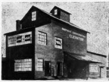
Good ventilation through big ventilators in Fenestra fire-proof steel windows helps to prevent dust explosions in grain elevators. It's a real advantage that may help you close the next elevator job that's up.
