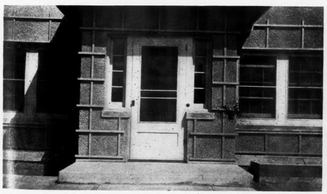
Detail of Front Entrance of Finished House, Showing Final Texture of Cement Stucco Finish. The wood lattice was added to soften the lines until shrubbery and vines have time to grow to do this work better.
