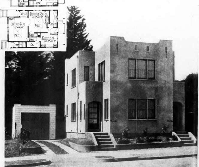
Photograph and Floor Plans of Two-flat Building of Mexican Design. Planned and built by Thomas N. Badger, Berkeley, California. Space-saving beds of the roller type are used.
