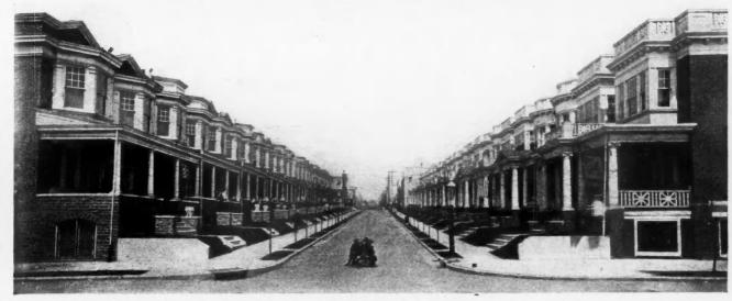
Residential Philadelphia Is Built Up Largely of Such Rows of Houses as the Above. Each unit is comparatively narrow and is lighted only from front and rear. Living room, dining room and kitchen are on the first floor with two or three bedrooms upstairs.
