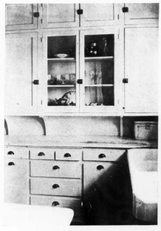
The Kitchen Is a Model of Neatness and Efficiency. All in white. This built-in cabinet goes clear to the ceiling, provides a well displayed section for best china and glassware, besides ample drawers and hinged compartments for cooking utensils and supplies.
