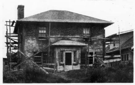
Concrete Block Residence After First Coat of Stucco Was Applied. The cement mortar joints between blocks are still discernible. With the final cost of cement stucco the wall presents a perfectly even tone that is permanent because the wall is of the same material thruout.
