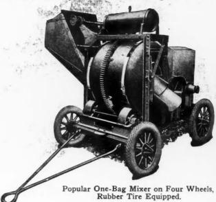
14 to 20 mile speed (while made for 4 to 5 miles), but the hard jolting and rattling soon works bolts loose, parts come out of alignment, battery and engine parts are harmed and the result is breakdowns and delays.
