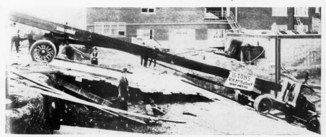
W. M. McMichael of Tulsa, a Hauling Contractor, Transported a Number of Massive Steel Beams from the Railway Cars to a New High School Site by Using a Regular 5½-Ton Dump Truck in Connection with a Trailer. In spite of twists and turns and steep inclines, the job was accomplished successfully and without mishap.
