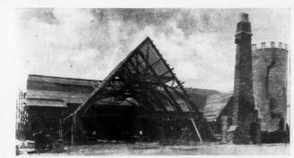
The New Riding Academy as It Appeared in Course of Construction. The chimney at the right was undamaged by the flames, and was incorporated in the newer structure.
