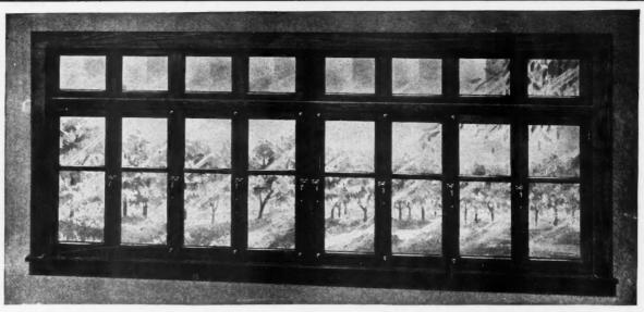
This AiR-Way installation consists of two series of four sash each. One series folds to the right; the other to the left. In this illustration all sash are tightly closed against the weather.
