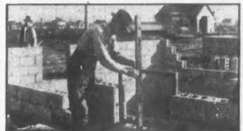
Plumb the window and build up the wall on either side.
