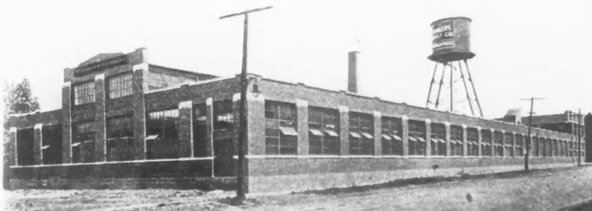
Under Certain Conditions of Site, Nature of Occupancy, Etc., the One Story Monitor Type Building Is Most Desirable.
