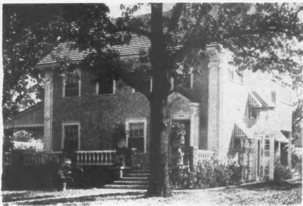
Residence of Mr. E. R. Mason, Des Moines, Iowa Architect, C. E. Cope Stucco on Sykes Expanded Cup Metal Lath
