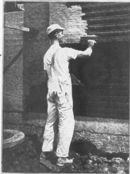
Applying scratch coat to E-Cod Fabric
