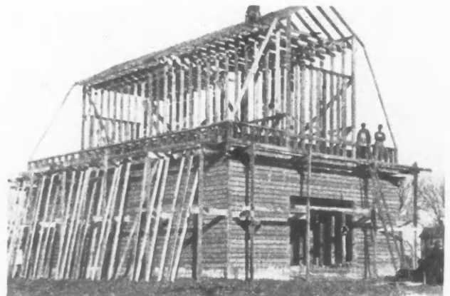
The Roof Structure Going Up on the Corncrib Which Was Designed by Mr. Burge from a Plan Memorized from American Builder.
