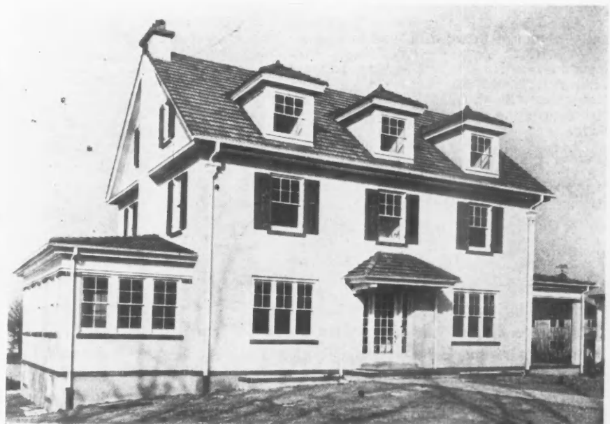
The Finished Residence as It Looked After Stucco Was Applied Over the Concrete Block as Shown in the Upper Photograph.
