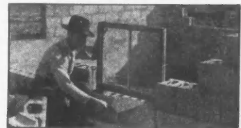
Set the Fenestra Window on the sill.
