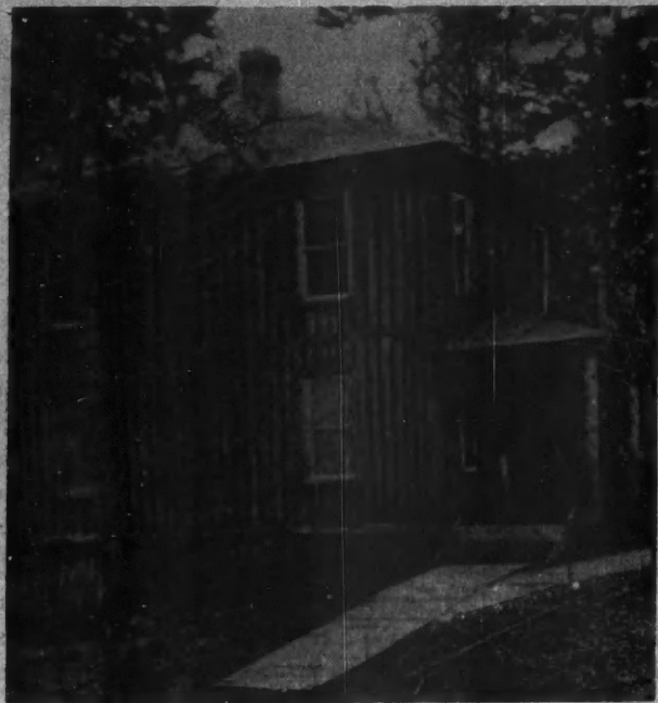
The Perpendicular Use of Logs Rising Up Two Stories, and it can be added to from time to time as one has the inclination.
