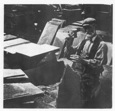
After the Slate Blocks Are Broken Across and the Preparatory Splitting Done, the Slabs Go to the Slate Splitter. Using a wide, flexible splitting chisel and a wooden mallet, he splits the slabs into slates of the desired thickness.
