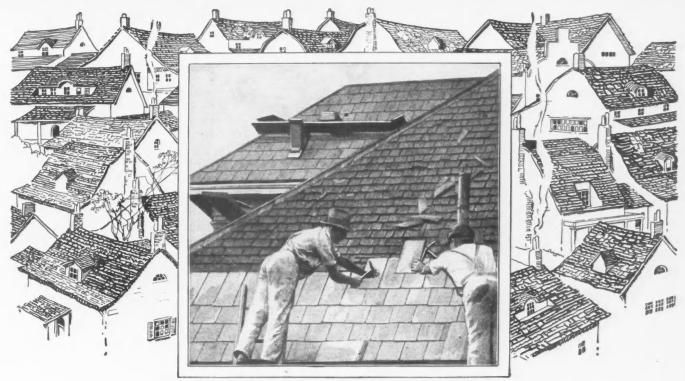
Laying Johns-Manville Rigid Asbestos Shingles right over the old roof
