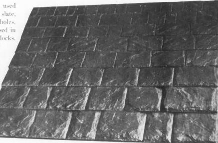
A Rustic Roof of Attractive Design, Made of Architectural Grade Slate. Not the least attractive part of a slate roof is this rugged, irregular, artistic effect. Properly manufactured roofing slate, laid according to established practice on uniform and strong supports of moderately steep pitch, provide a roof that will not leak.
