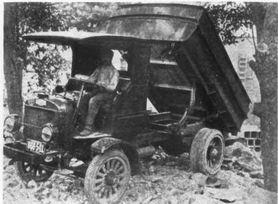
Contractors and Builders, and Especially Those Specializing in Road-Building Work, Find Substantial Advantage in Using Swinging, Adjustable Partitions in a Dump Truck Body, as Shown to Right.
