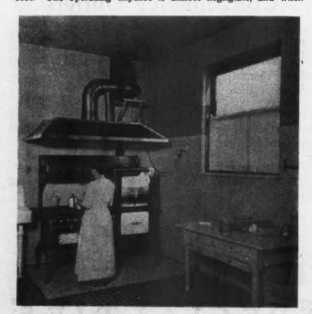
This Ventilator Is Built Into the Range Flue. Power is taken from a light socket or especial wiring can be provided.
