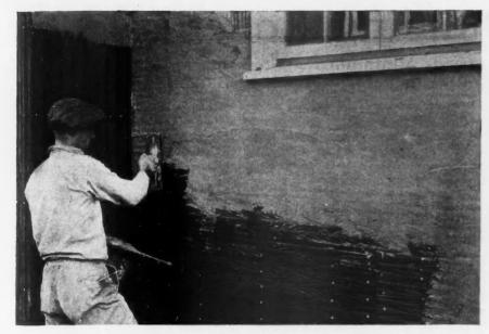
Strips of Carefully Selected Wood Are Pierced and Sliced by Special Machines and Backed with Waterproof Paper to Form This Expanded Wood Lath. The plastic mass oozes through and around, forming a perfect key.
