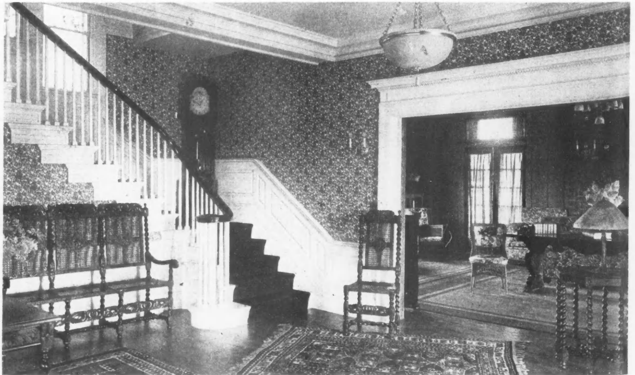
Stains Enhance the Beauty of Interiors, of Floors, of Staircases. This living room, visible from the hall, is panelled in oak and stained antique finish. Fumed, weathered, early English, Flanders, mission, silver gray, frosted, smoked, gray-green, Italian, Jacobean or Hungarian stains are others which lend character to an oak interior.
