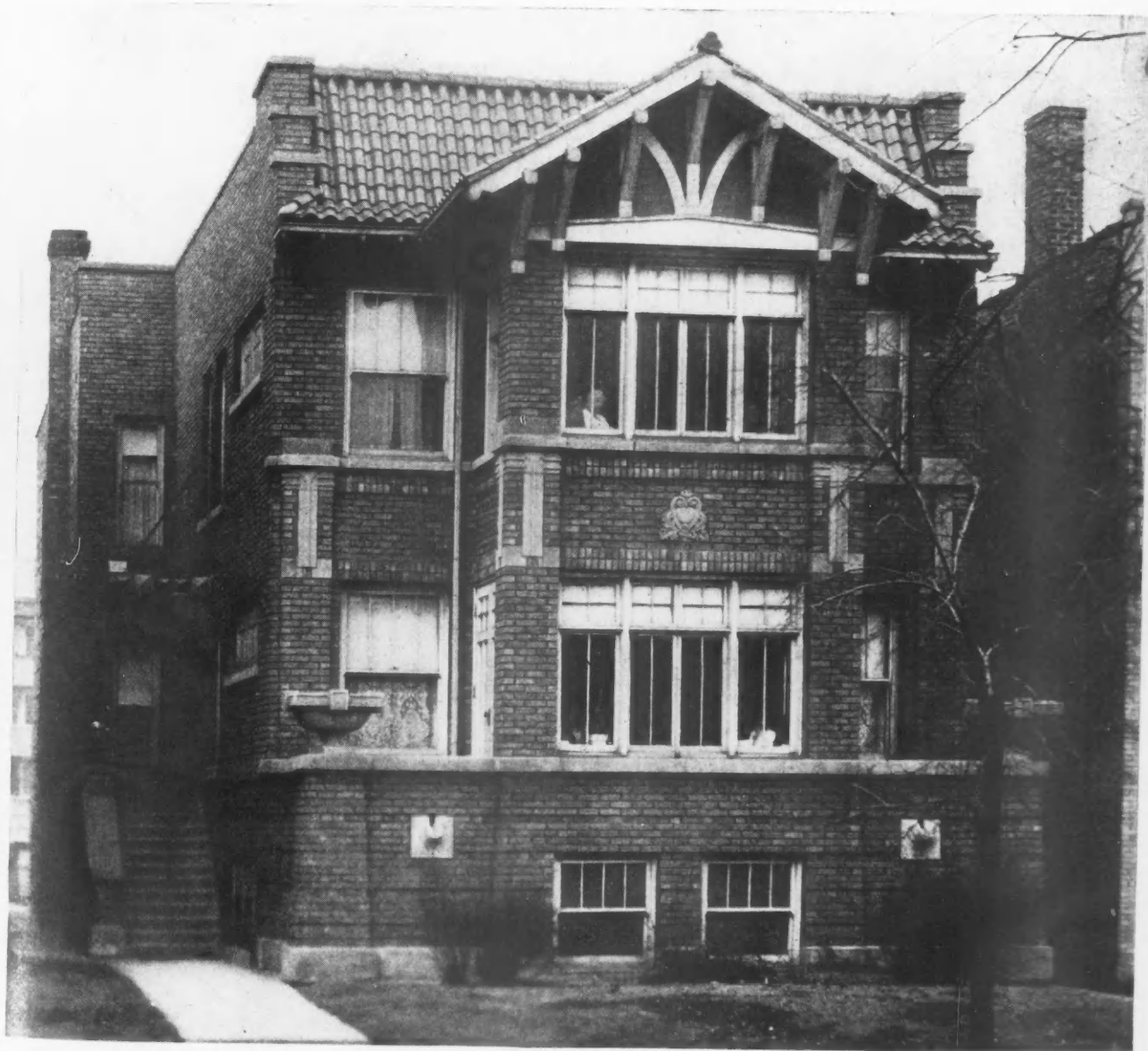
This Two-Apartment Is Designed for a Forty Foot Lot, and the Floor Plan Is Identical for Both Floors. The side entrance is a feature many appreciate, since it saves apartment room at the front of the structure.
