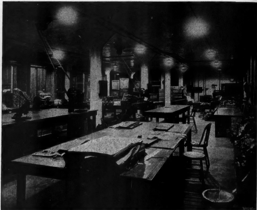
These Lights, Hung Close to the Ceiling, Furnish Ample Illumination for Close Work on the Tables in This Merchant Tailoring Establishment.
