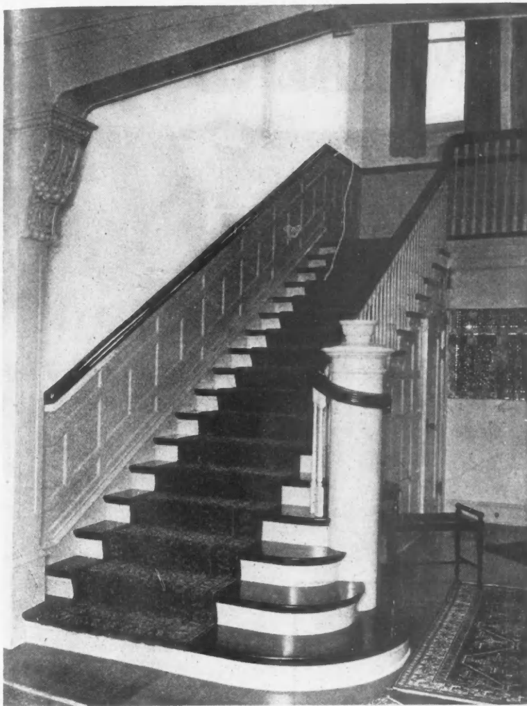
In This Attractive Hall the Panelling and All the Staircase Woodwork Is of Southern Pine, as Is Also the Floor.
