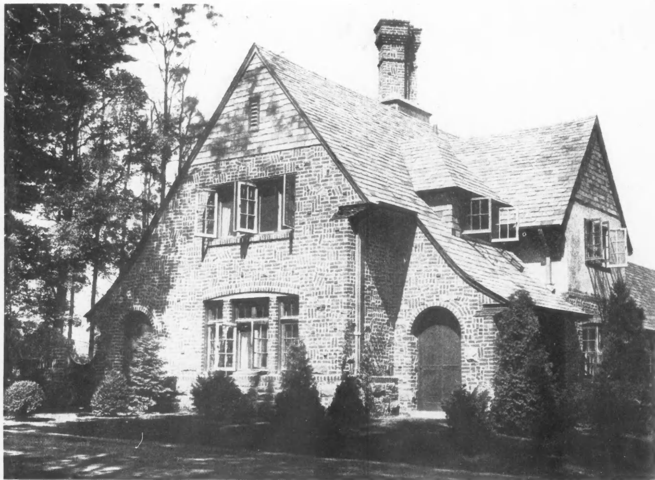
Note How the Jagged Blocks of Red Sandstone Are Combined with the Oddly Laid Brick of This Residence. The irregular slate roof and evergreen plantings and casement windows complete the illusion of quaintness. Donn Barber, of New York, was the Architect. Owner, George W. Hale, Esq., Oyster Bay, N. Y.
