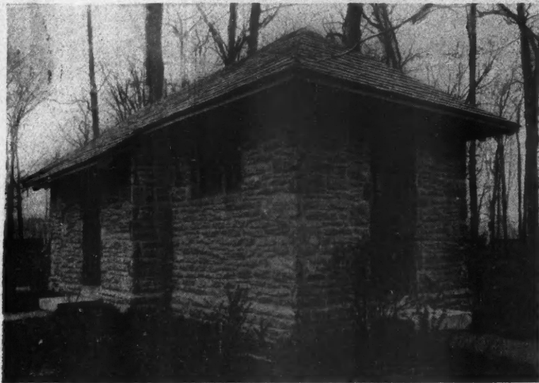
Convenience Station, Torresdale Park, Philadelphia, with Broken Ashlar Rubble Stone Walls. Designed by W. E. Roletter, City Architect's office.
