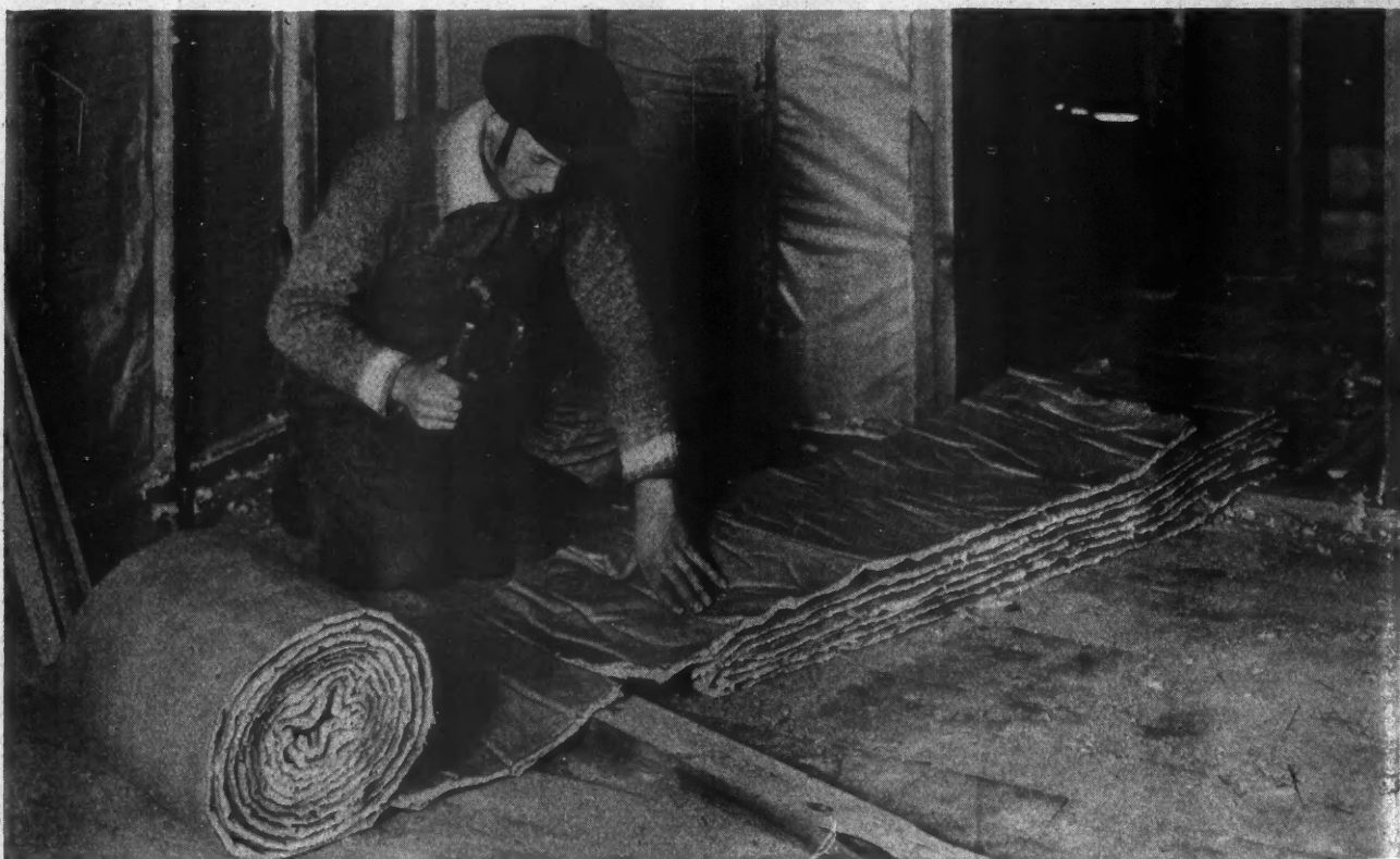
Insulating Material Takes Many Forms. One of the most effective and interesting withal is this type, evolved by a large producer of forest timber. It is really wood wool, fluffed; will not burn, and makes a snug blanket for wall or ceiling.
