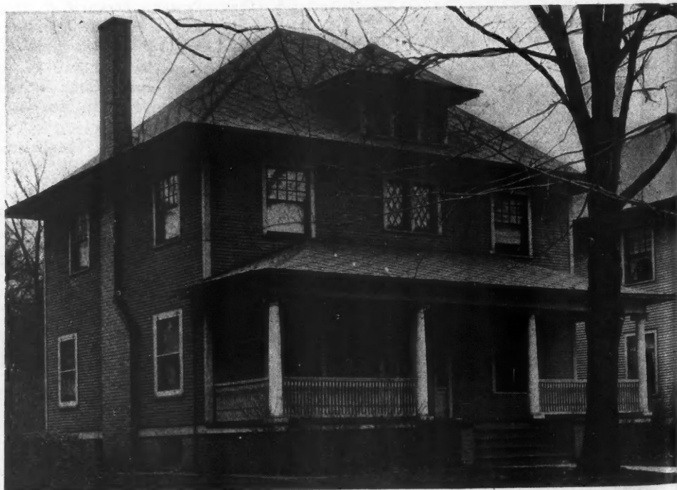
This Attractive Roof Is Composed of Hexagonal Shaped Asphalt Shingles That Interlock, Making Curling, Warping and Blowing Impossible.
