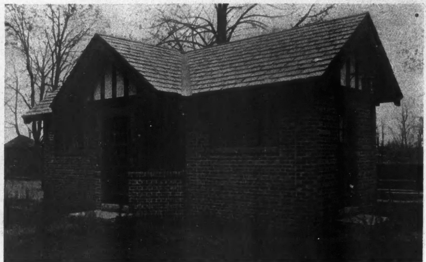
Convenience Station, Disston Park, Philadelphia. Combination brick and stucco timbered construction. Designed by W. E. Roletter, City Architect's office.
