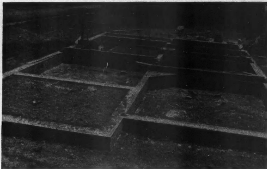
The Inside and Outside Walls, Up to Joists, of $5,000 Ideal Wall Brick Home. The dimensions are 30 feet by 50 feet over all. The walls are 8 inches thick.
