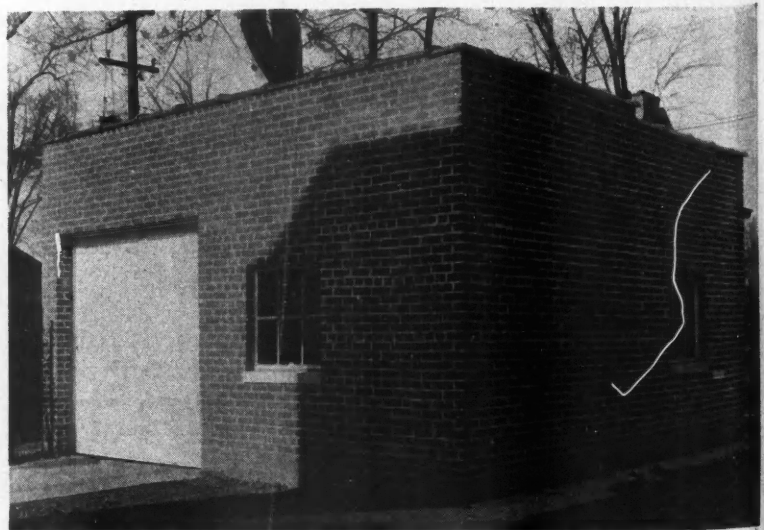
Steel Windows Help Make the Brick or Concrete Garage More Fire-Resistant. The steel sash unit is more easily handled if ventilator is wired shut when inserting. Arrange for inside glazing.
