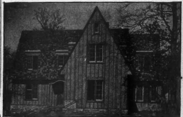
House near Chicago, showing its "underclothing" of Cabot's Quilt, with furring strips over the Quilt, on which the outside finish is laid. Roof also insulated. Leon B. Stanhope, Architect, Chicago
