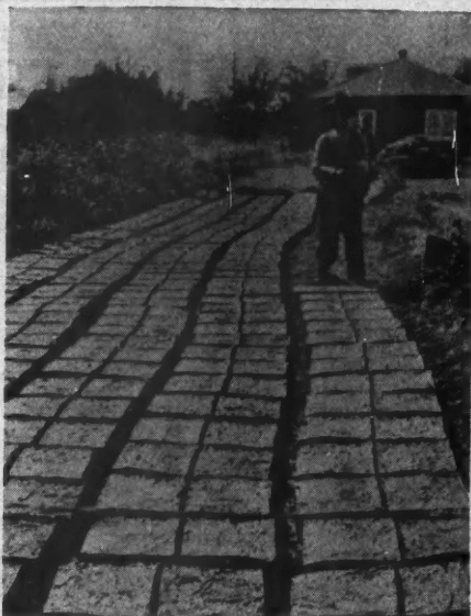
Adobe Bricks Being Cured in the Sun. Looks like some new-fangled pavement—or maybe fudge!
