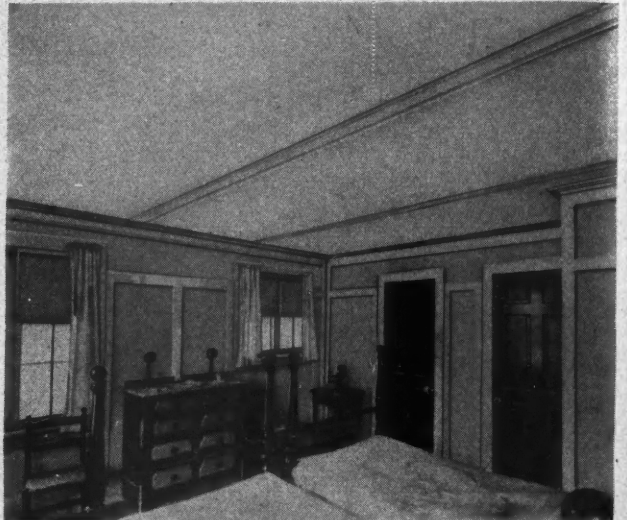
One of the Bedrooms in the Osborn Cottage Finished in Wide Panel Wallboard.
