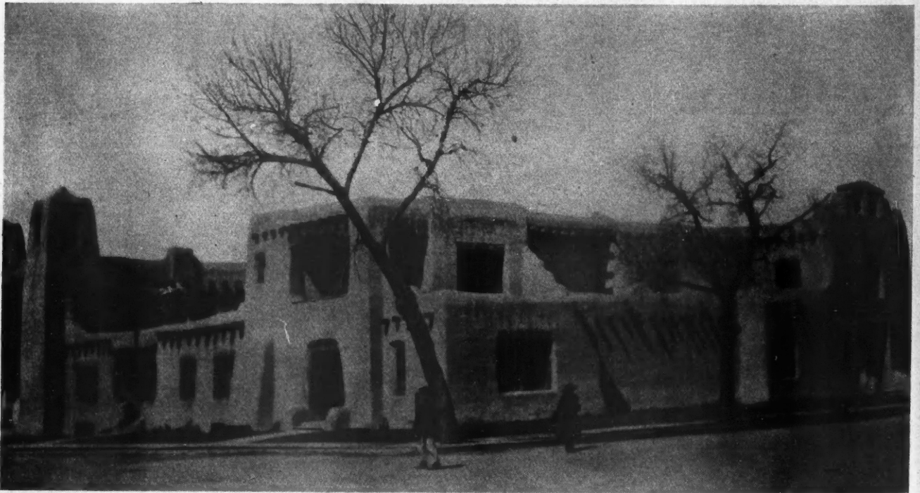
This Is the Old Museum, Santa Fe, N. M., a Building of Undefined Pueblo Architectural Design, and Constructed of Adobe Brick. Far from being a flimsy makeshift, adobe walls are well fitted for a museum. They are air-proof and fire-proof. Unusually heavy and strong they will withstand any wind short of a cyclone. They give a fine mellow texture to the walls, do they not?
