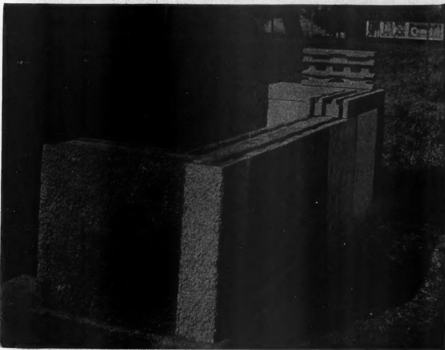
As Often as Three or Four Rows of the Blocks Were Laid, Grout Was Poured Into the Center Openings, Being Puddled Somewhat to Force It Into Horizontal as Well as Vertical Openings.
