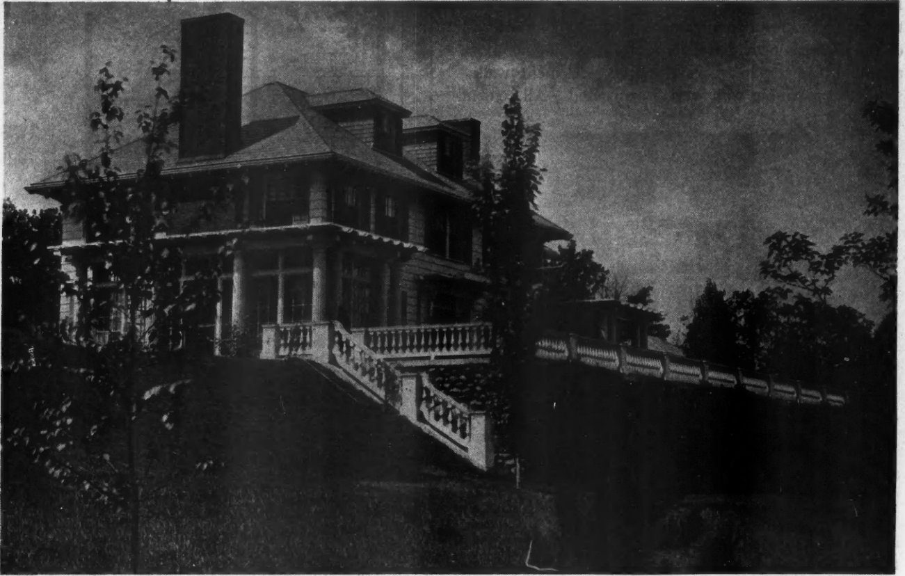
Turning a Defect of Location Into an Advantage. With cobbles picked from a nearby field a retaining wall was built, giving a broad terrace to the house.
