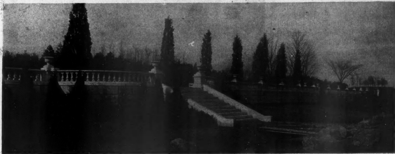
Making the Most of an Abrupt Slope. Comparatively little earth hauling was required for this retaining wall, but an imposing result was obtained.
