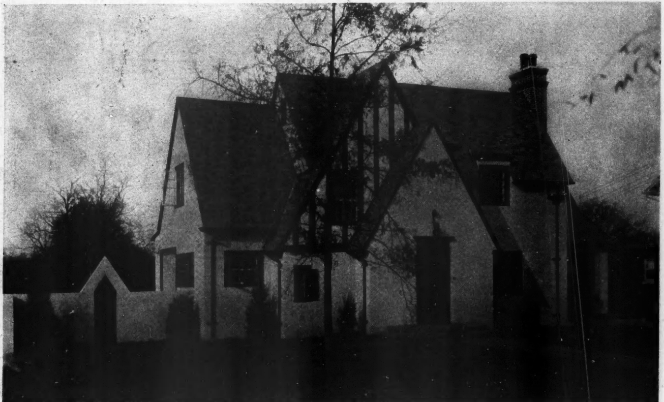
The Interesting Treatment of the Gables in this Home, with the Idea Developed Even in the Garden Wall, Forms a Motif of Unusual Interest. The one timbered gable makes an interesting contrast while the attractive, shuttered small window and the details of the entrance and door all do their part in adding attractiveness to the house.
