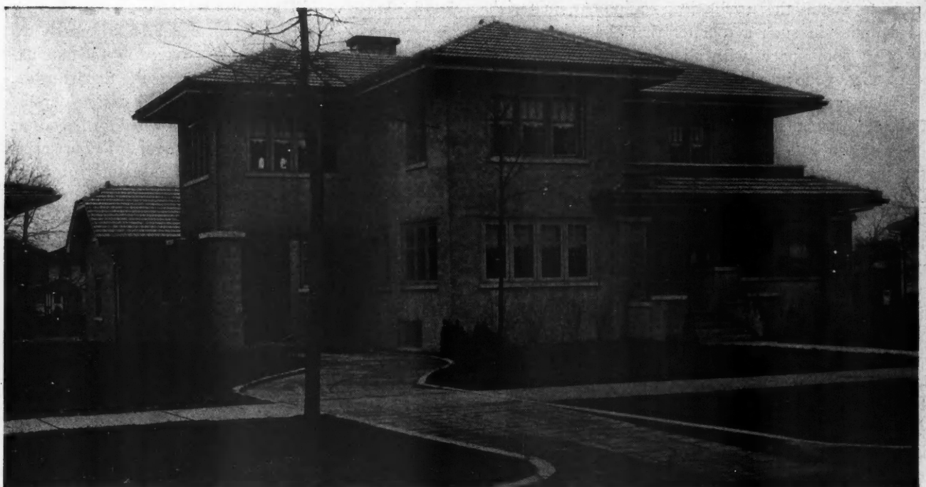
The Walls of This House Are of Concrete Block, Laid Dry Without Mortar, the Center Openings of the Block Filled with a Grout of Portland Cement, Sand and Water, and Later Stuccoed with Cement.
