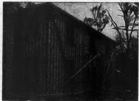
This shows a house insulated with Cabot's Quilt, ready to receive the outside finish. Russell S. Walcott, Archt., Chicago, Ill.
