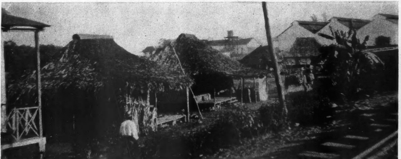
At San Jose De Guatemala We Found Nothing but a Few Native Huts and Warehouses as This Is the End of the Railroad. Thatched roofs and cane walls comprise the bulk of the material used in the construction of a native hut, which in some instances have wooden floors, but in the majority of cases have no floors at all. Babies, pigs, dogs, ducks and chickens all have equal rights in the houses, and to us it seems particularly dirty and filthy when compared with even the poorest of homes in the United States.
