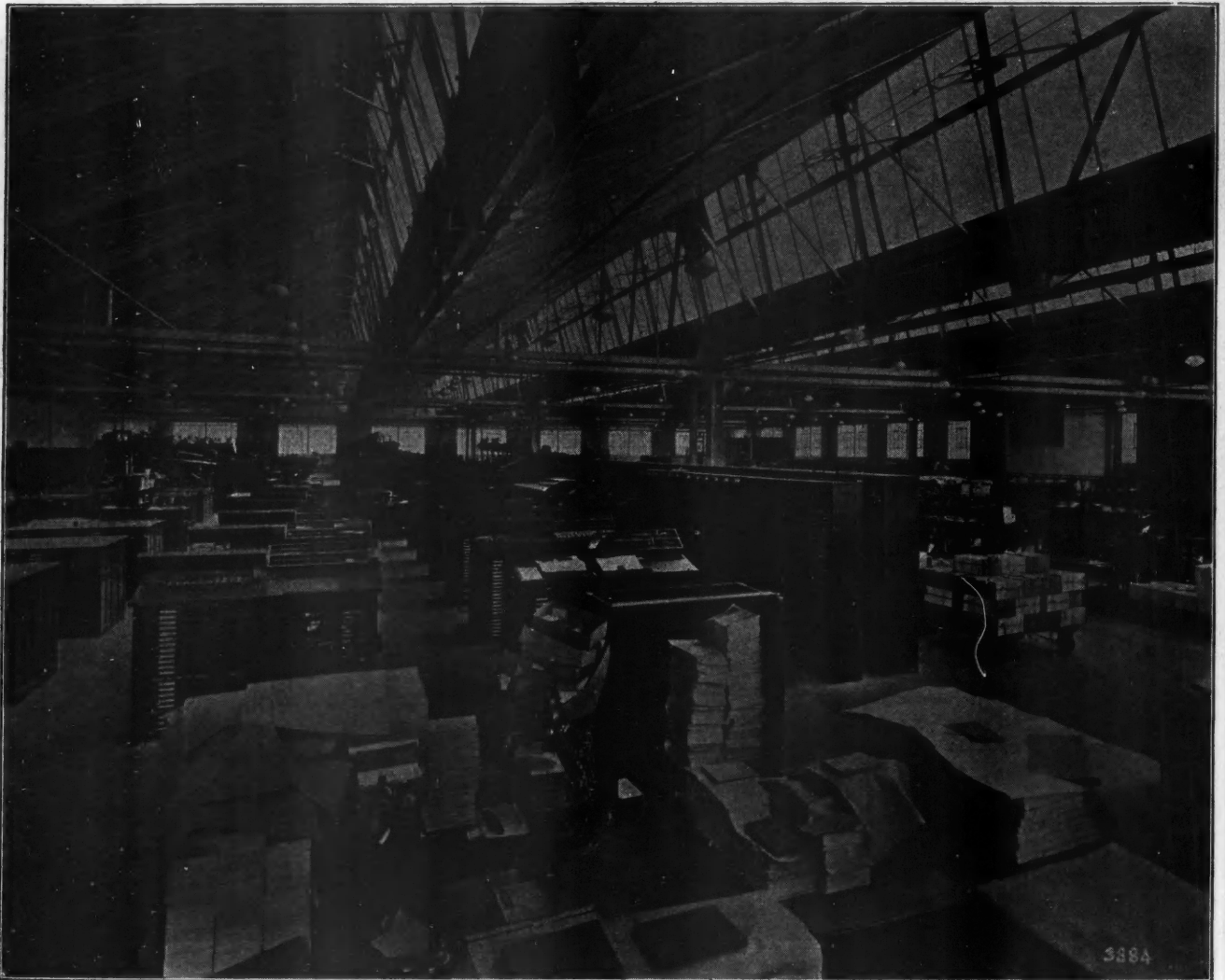
Illustration courtesy The Ballinger Company, Philadelphia. View of Saw-Tooth Printing Building from Composing Department Showing Unusual Daylight Illumination.
