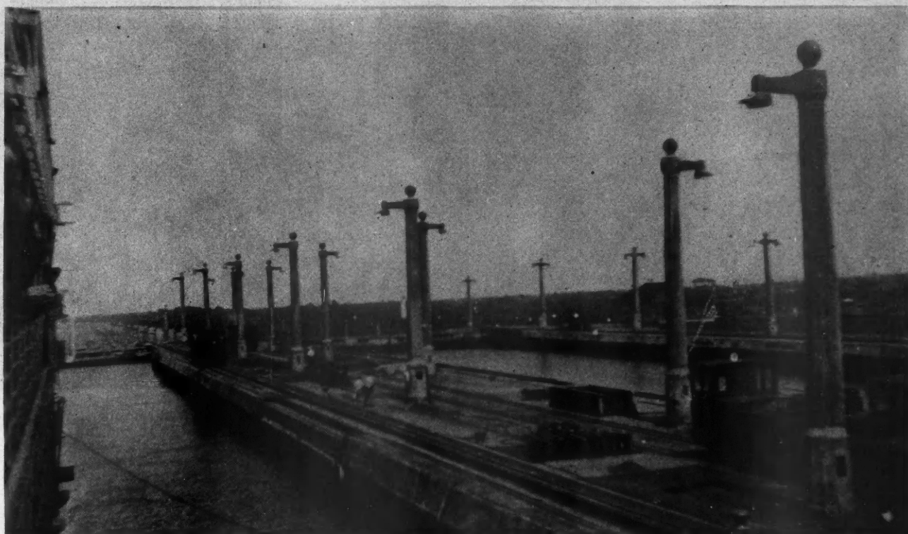
Gatun Lock. This Photograph Was Taken at Gatun Lock, Showing the Electric Mules, Taking Our Boat, the Steamship "Colombia" Through the Series of Three Locks on the Way to Colon. In bringing the boat from the Atlantic Coast to the Pacific up to different levels, one would imagine it would take considerable time to fill the lock with water. However, by a series of flood gates at the bottom, all of which are opened at once, it takes less than five minutes to raise the boat 38 feet. It takes approximately 6½ hours to go from Balboa to Christobal and one is impressed the whole journey by the fact that the entire organization and enterprise depicts American energy and thoroughness.
